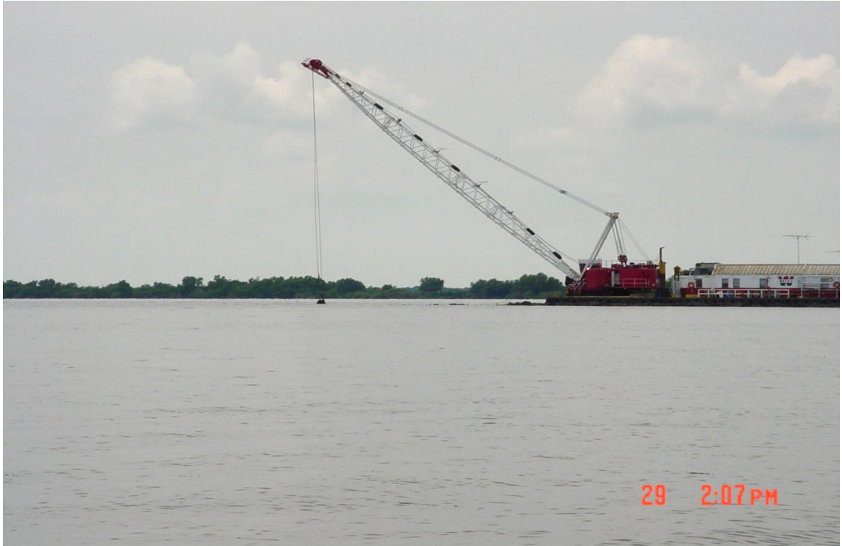
Figure 2 Sediment Trapping at the Jaws (TV-15) under construction on 7-2004.
