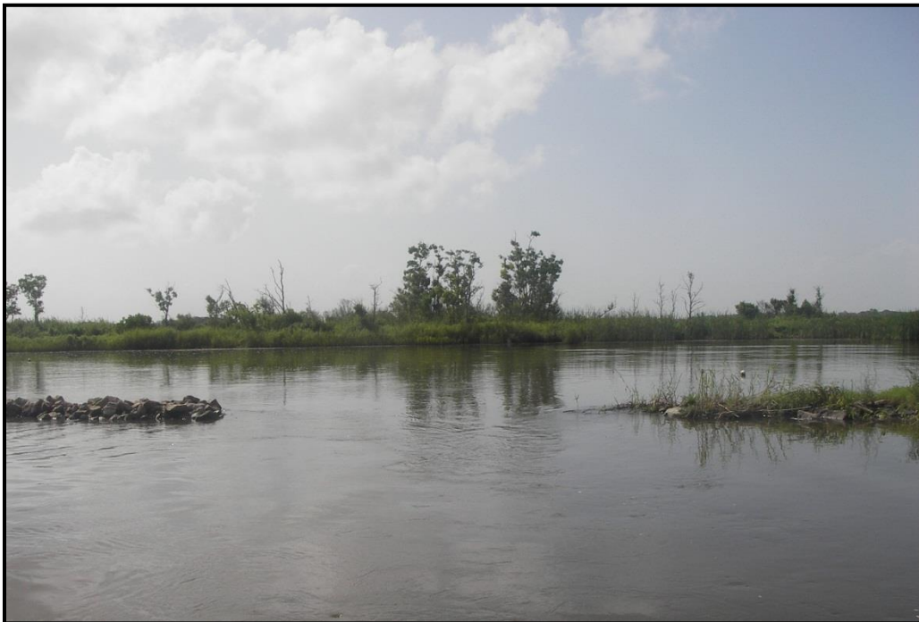
Photo No. 6, Rock plug gapped as part of maintenance event. (photo taken 07/02/2012)
