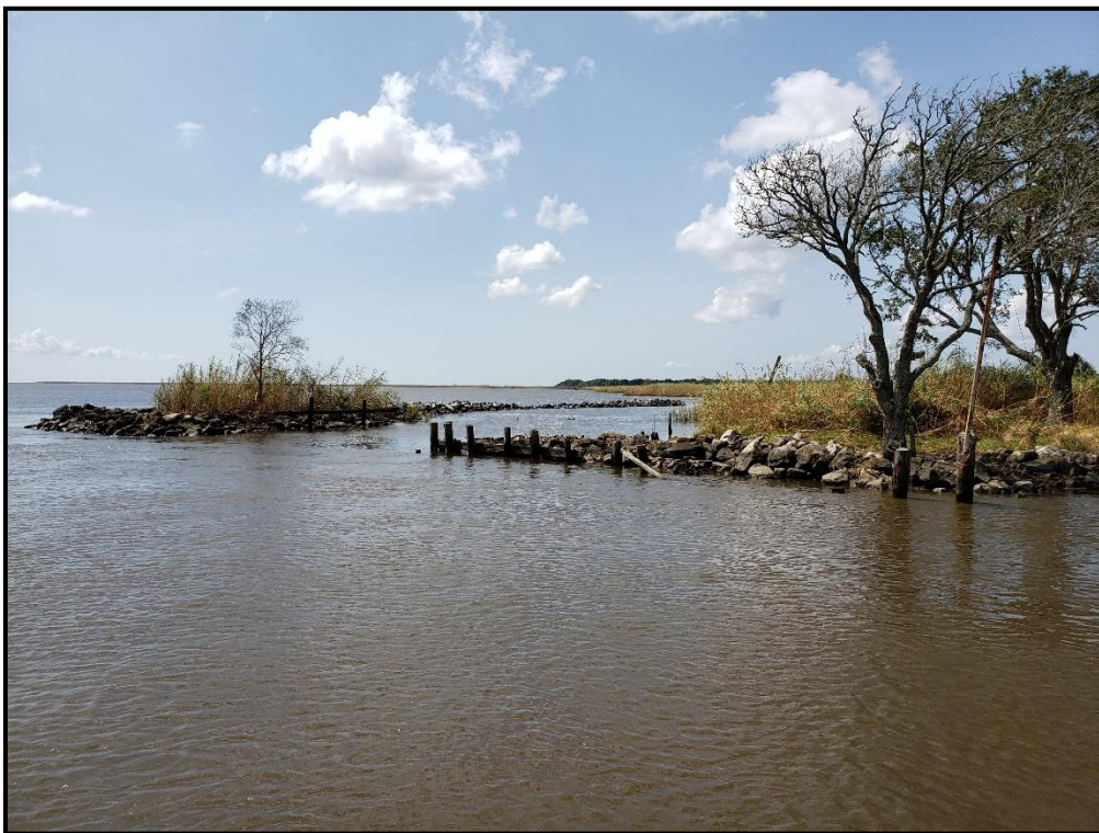
Photo No. 2, Rock revetment at Oaks Canal, west side
