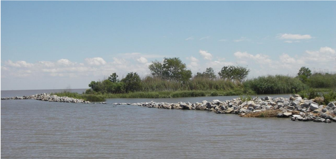
Photo No. 5 , Nourished Area No. 4, Plug (TV-14 Project- End of East West Canal Looking North)
