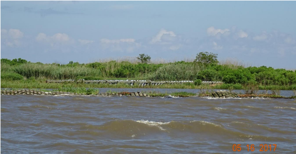
Photo No. 1, MC Cell No. 1 - Articulated Concrete Mat (2015 Maintenance Event)
