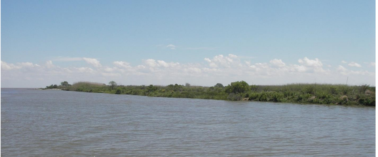
Photo No. 3, MC Cell No. 1, North South Canal Looking North
