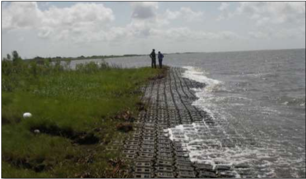
Photo 2- East side –Revetment of Gulf Shoreline
