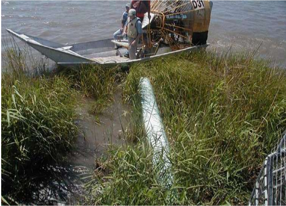
Photo 5—Area 3, 15-in. drain pipe on southern plug of north canal
