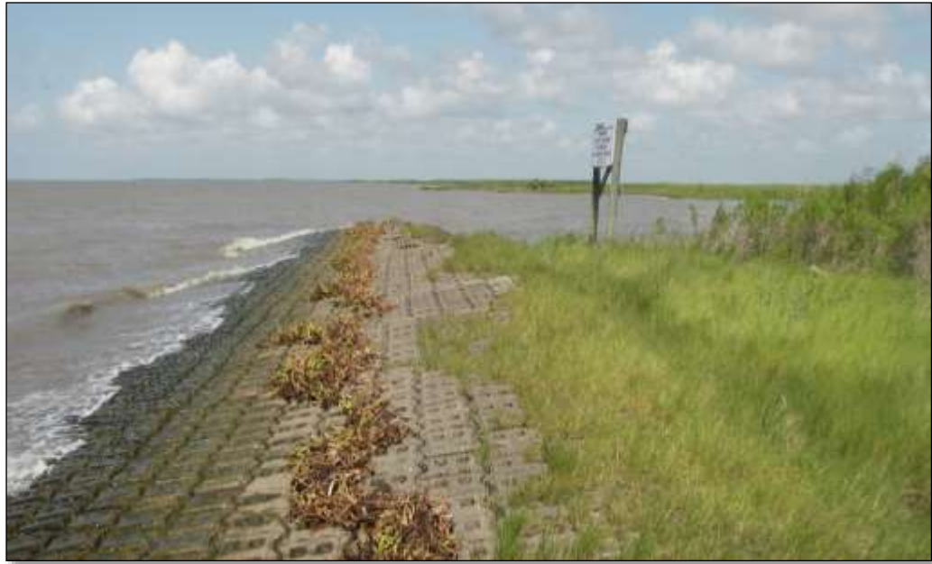
Photo 3—Area 2, Revetment on gulf shoreline
