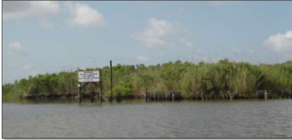
Photo 1- Timber Bulkhead on Hell Hole
