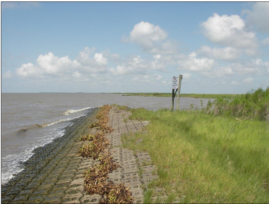
Photo 2, Area 2, West side of concrete mats.
