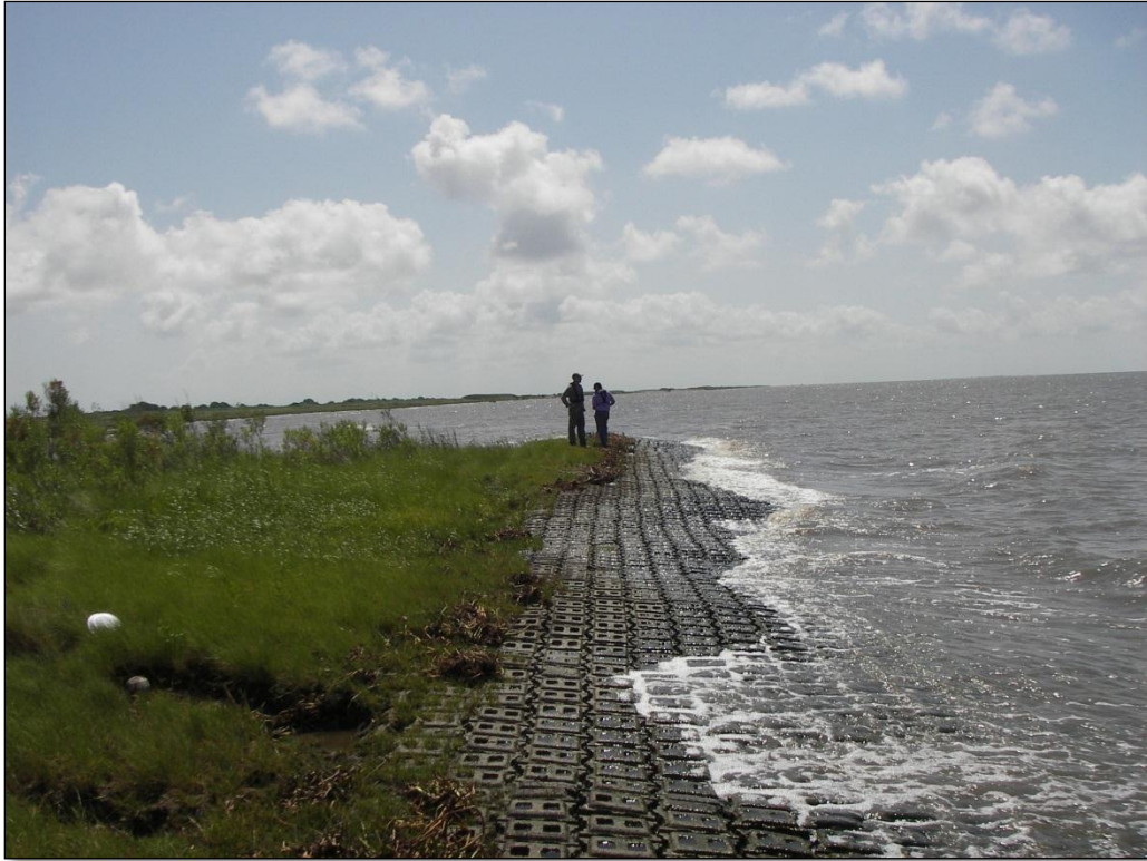
Photo 3, Area 2, East side of concrete mats.
