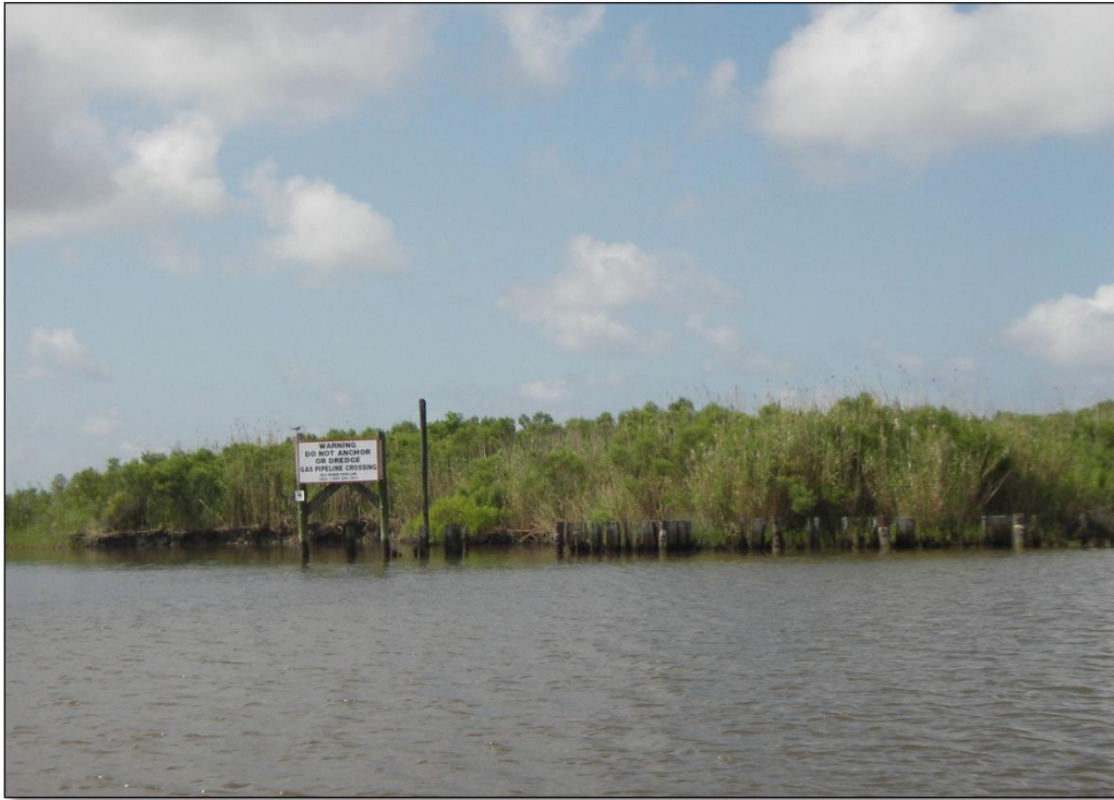
Photo 1, Area 1, Timber bulkhead.
