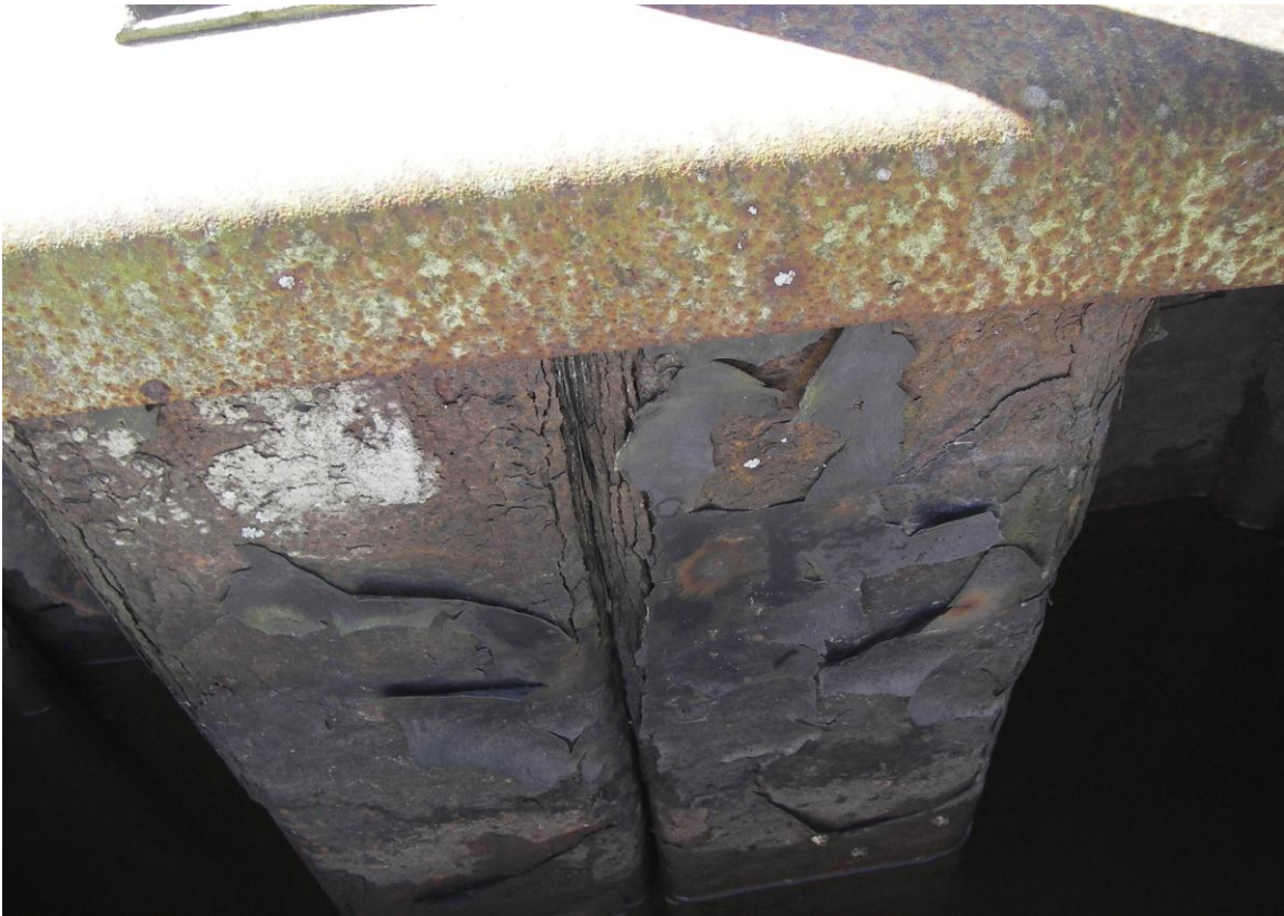
Photo 18 —typical rust on Fixed Crested Weir Sheet Pile
