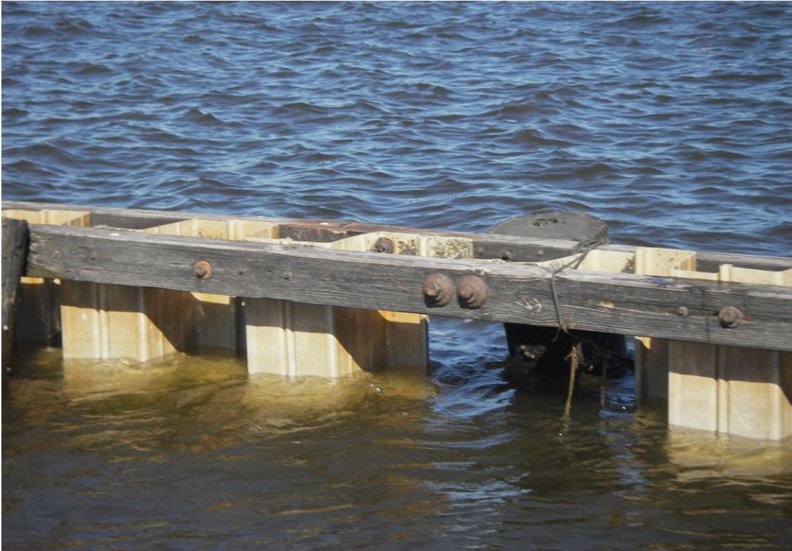
Photo 15 —Typical section of PVC wall
