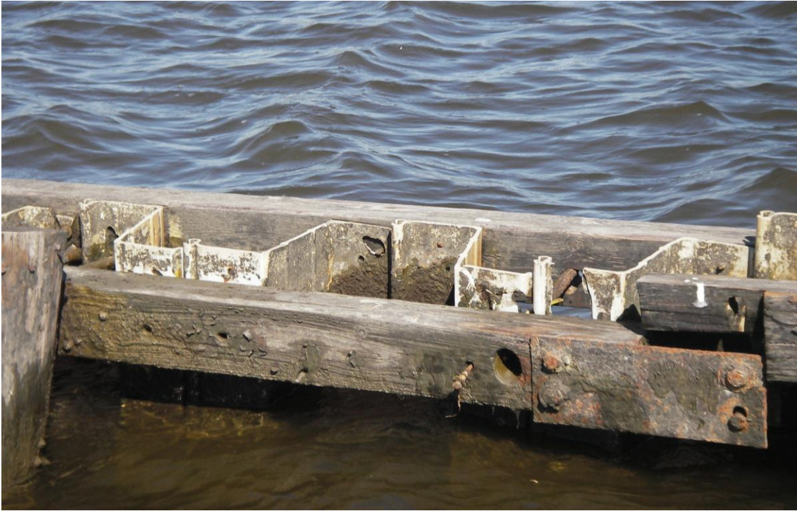
Photo 17 —rusted/broken hardware on old PVC wall
