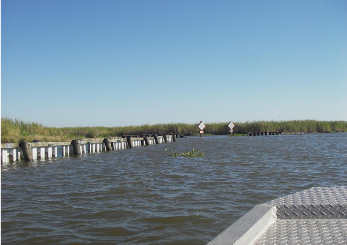
Photo 11 —Jackson Bayou structure (and new PVC wall)
