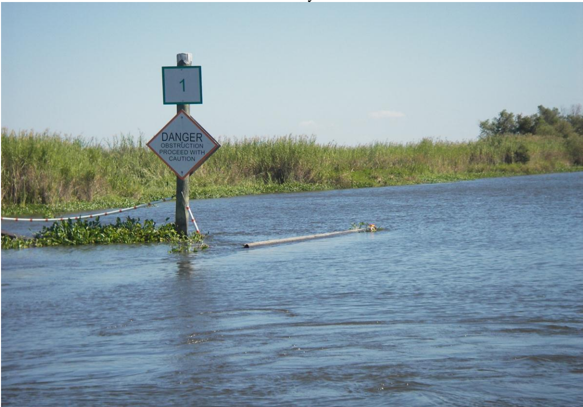
Photo 2—Broken pile and sign at Humble F Canal structure
