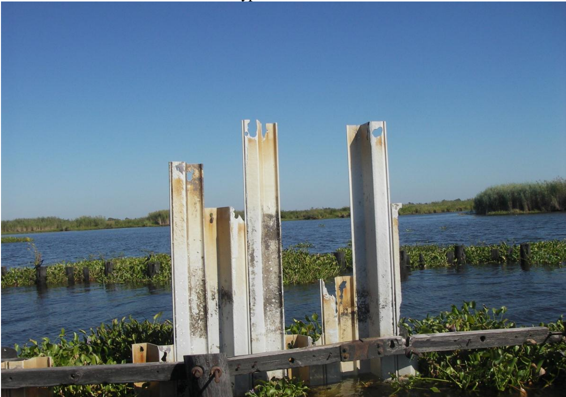
Photo 16 —rising sheet pile on PVC wall
