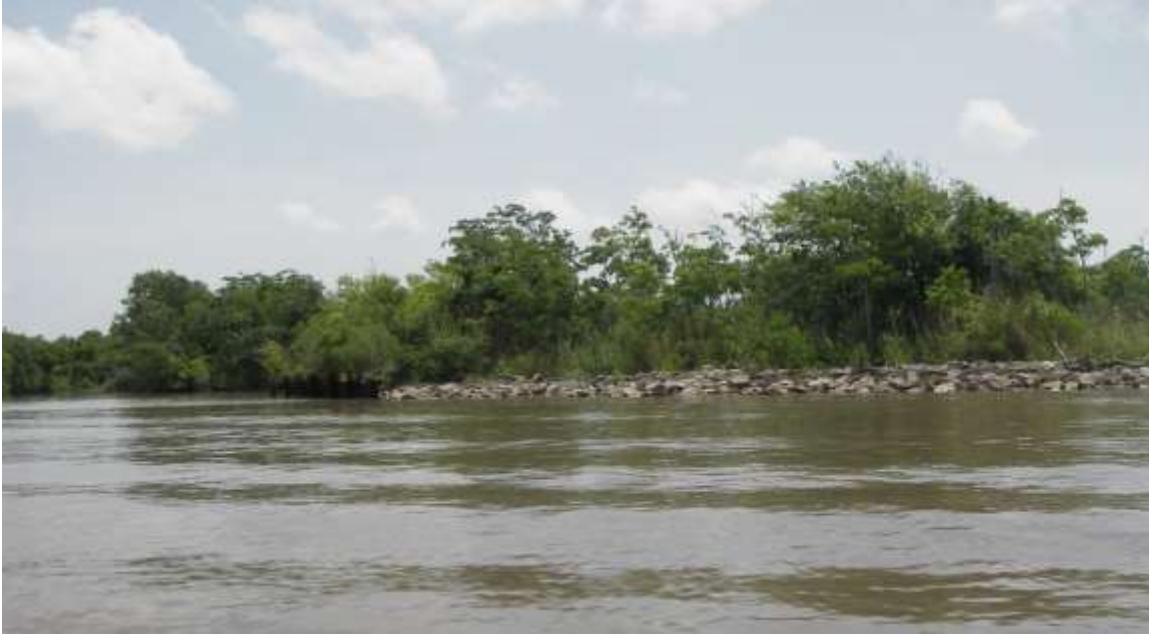
Photo No. 1 —north end of dike
