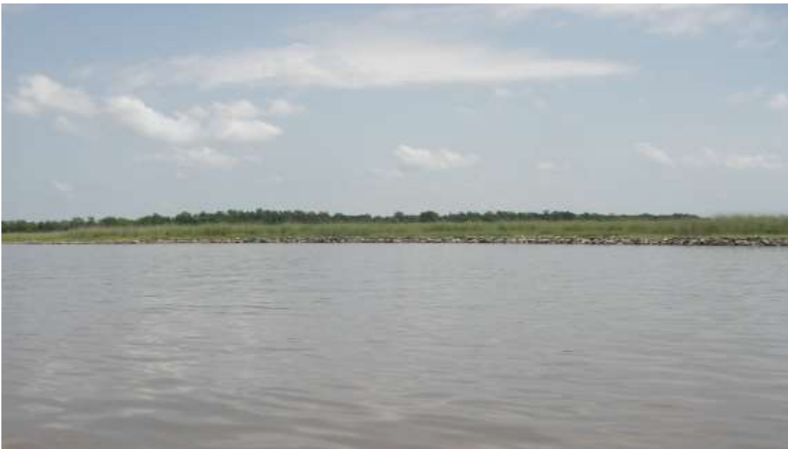
Photo No. 2 —typical reach of dike
