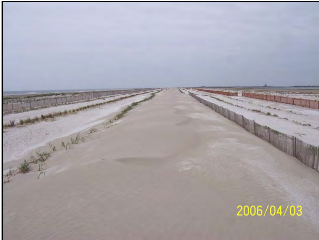
Photo 2. View of new sand fence (right), existing north sand fence row and sand dune (middle), and existing south sand fence row (left) standing on north fence dune looking west near mid project.
