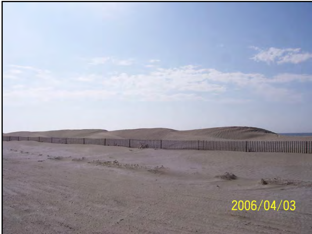
Photo 10. Photo of sand dune built up along the south side of the existing north fence row near east end of dune platform looking southeast. Material can also be seen on the north (near) side of fence.
