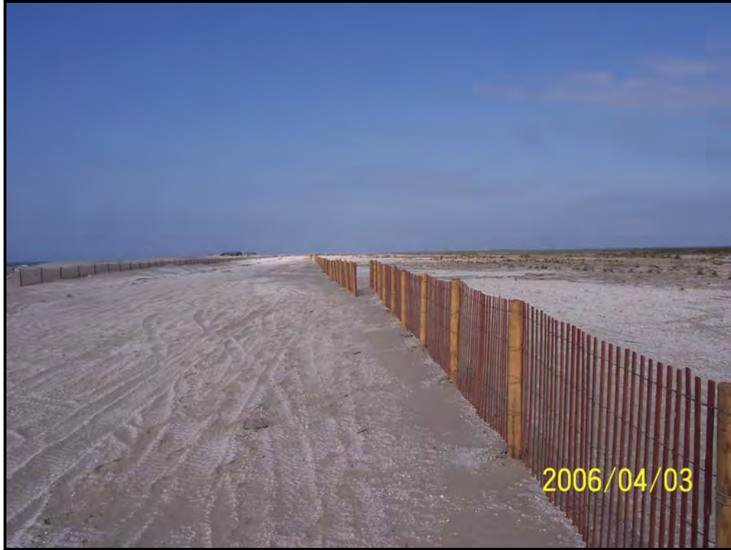
Photo 1. View of new sand fence east of camp looking west. Existing north row of fence can be seen on left.
