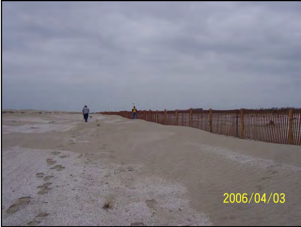
Photo 3. View of new fence near west end of project looking west. Wind-deposited sediments can be seen building up on the south side of the fence row.
