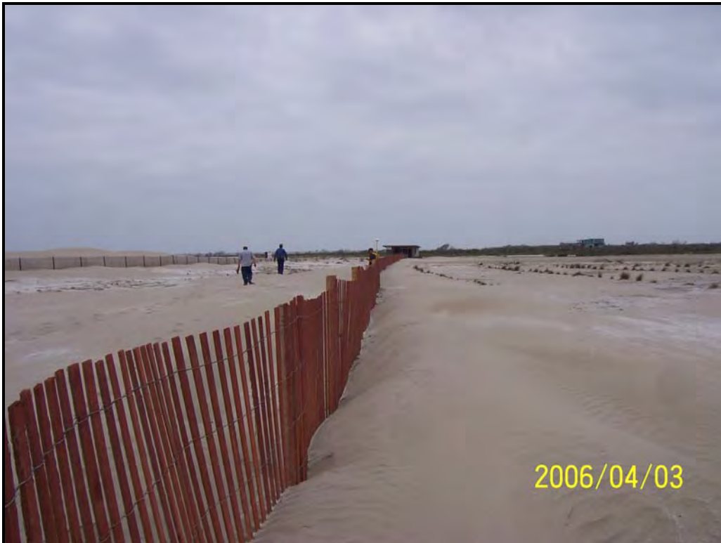
Photo 4. View of new fence near west end of project looking west. Wind-deposited sediments can be seen building up on the north side of the fence row also.
