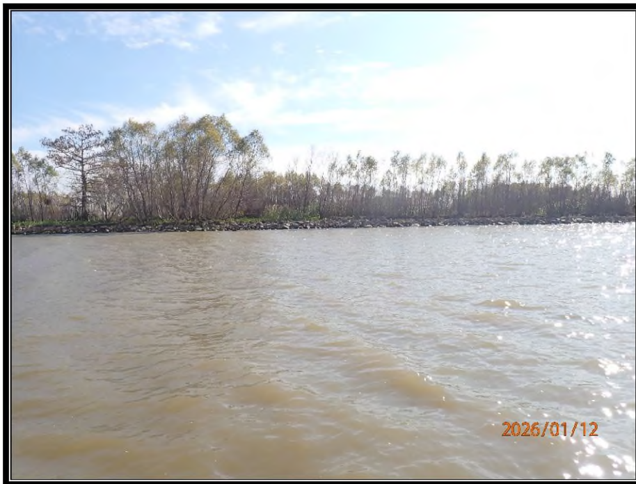
Photo No.16 - rock dike and marsh creation area along Bayou Chene on west side of Bayou Penchant.
