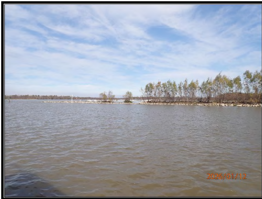
Photo No.12 – rock dike and marsh creation area along Bayou Chene and Bayou Penchant.
