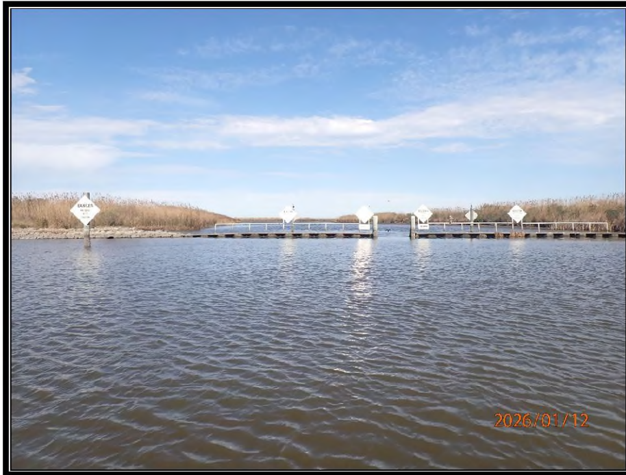
Photo No.9 – view of weir structure at Site No.5 along Bayou Decade near Lost Lake south of Site No.4 and rock dike tie in on the south side of the structure.
