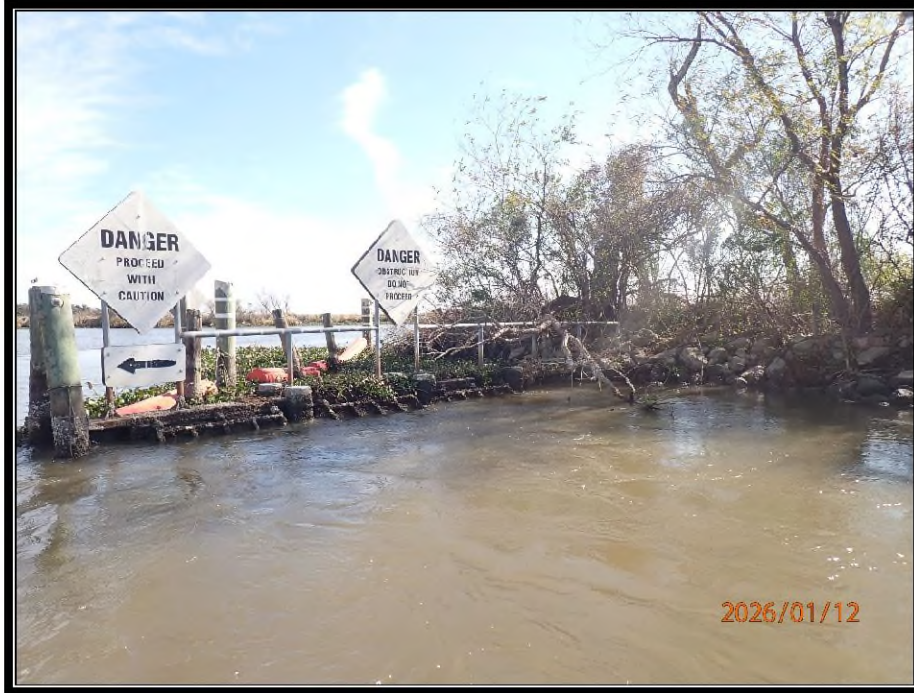
Photo No.3 – view of vegetative debris trapped between bulkhead and debris barrier at the Brady Canal Structure.
