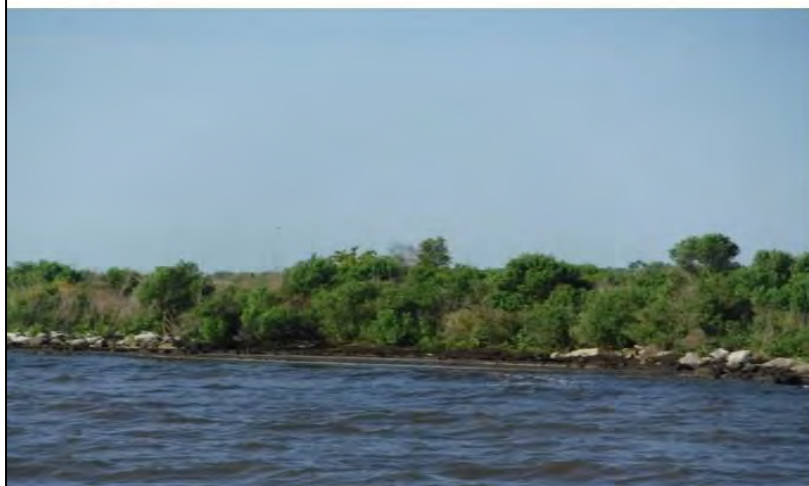
Photo 14 (8313) – near Sta. 415+00 – rock dike overgrown with vegetation with sediment buildup in front of structure (Southern Segment).
