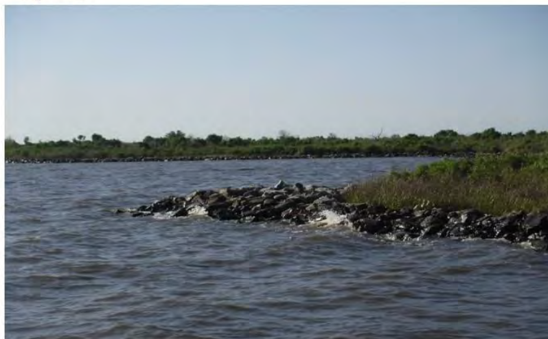
Photo No. 16 (8316) – near Sta. 423+00 – rock dike shoreline (Southern Segment).
