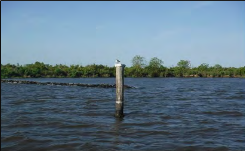
Photo No.9 (8303) – near Sta. 154+00 and 300+00 – missing sign at rock dike gap (End of North and beginning of Central Segment).
