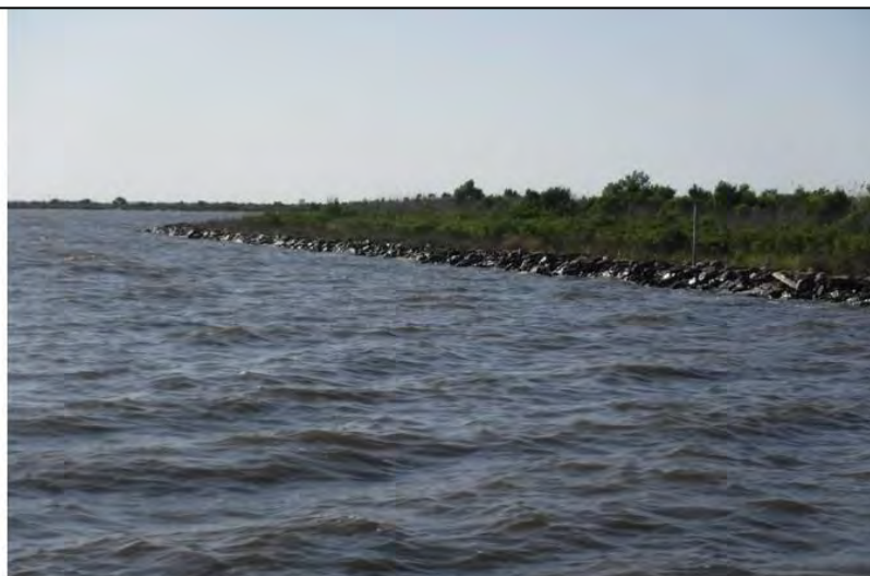
Photo No. 15 (8315) – near Sta. 417+00 – rock dike shoreline (Southern Segment).
