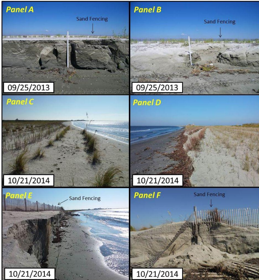
Figure 21. Oblique images depicting scarping of the West Belle Pass Barrier Headland Restoration (TE-52) project's dune feature in 2013 and 2014. Note the severe scarping that occurred several months after construction and the distance to the sand fencing in 2013 (Panels A and B). Panel B also shows channel formation during high water events along the eastern reaches of the dune feature. Several channels formed on the supratidal elevated expanded beach and dune template. Panels C and D display the eastern edges of the remaining dune. The dune feature no longer exists along the eastern reaches of the project. The area can be currently classified as washover and dune terrace landforms. Panels E and F exhibit the erosion of the dune all the way to the sand fencing which was placed in the center of the dune. Sand fencing only remains on the western and central reaches of the dune. The sand fencing that was installed on the eastern reaches of the dune has been leveled by wind and wave energy.
