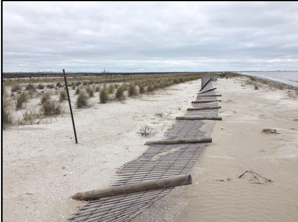
Photo A-5. View of damaged sand fencing, looking east.
