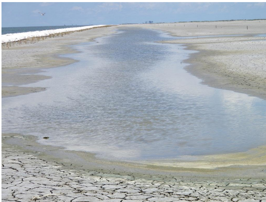
Photo 24: Typical containment borrow channel for the TE-48 marsh creation area (Raccoon_179). Note differential settlement after filing creates lower elevations in pre-dug areas.
