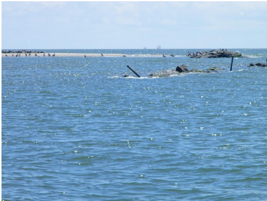
Photo 12: TE-29 breakwater #3 looking north (Raccoon_068). Note low elevation, leaning settlement plates, and lack of wave diffraction behind the breakwater. Also, note higher elevation of breakwater #1 and #2 in background.
