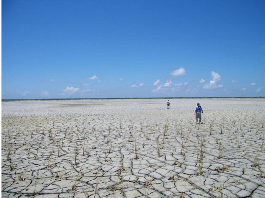
Photo 19: TE-49 marsh creation area looking south (Raccoon_148). Note persons walking on fill beyond locations plantings contractor could access on previous attempts indicating good settlement and compaction.
