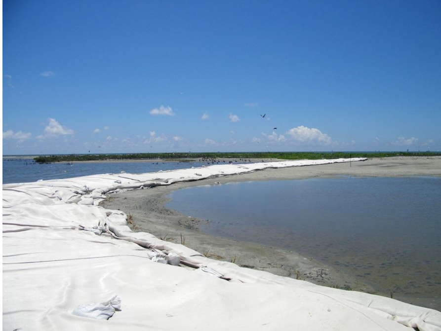
Photo 17: TE-49 marsh creation back dike eastern tie in looking southeast (Raccoon_141). Note slight low spot in fill area due to pipe wash out.
