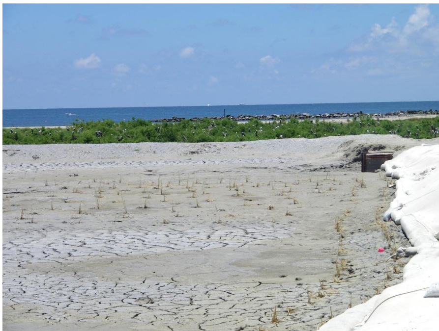
Photo 26: TE-48 marsh creation area western end containment tie-in (Raccoon_178). Note spill box still in place currently provides water exchange while sediment consolidates.
