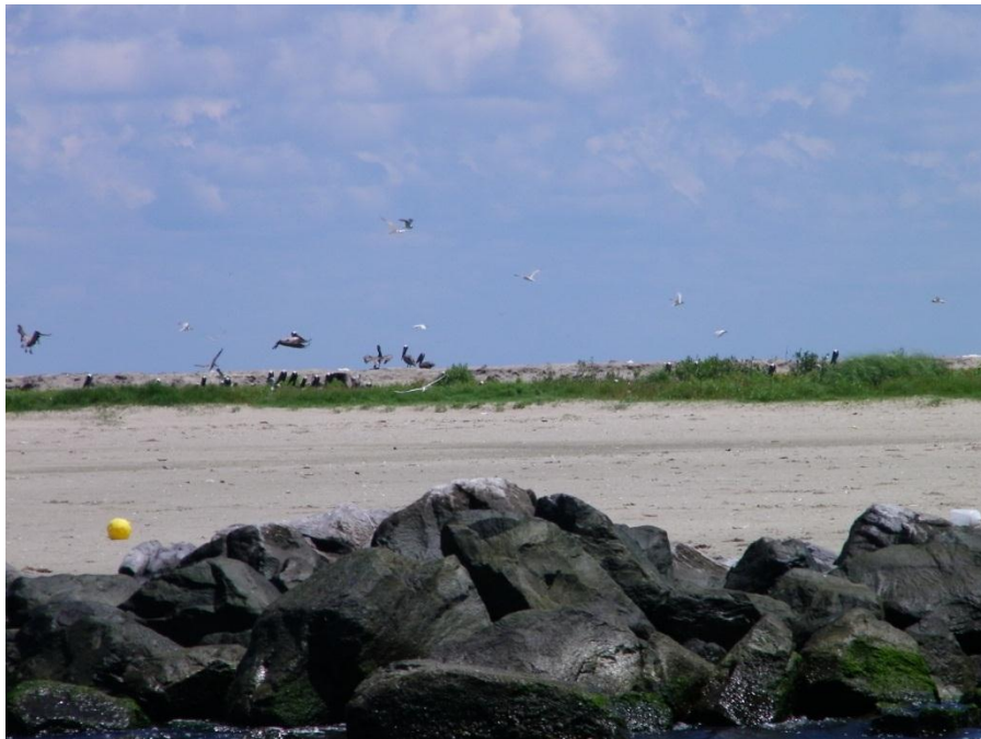
Photo 10: TE-48 breakwater #9 looking north (Raccoon_068). Note salient formation behind breakwater and narrow existing vegetation behind which is the unvegetated TE-48 marsh platform containment dike.
