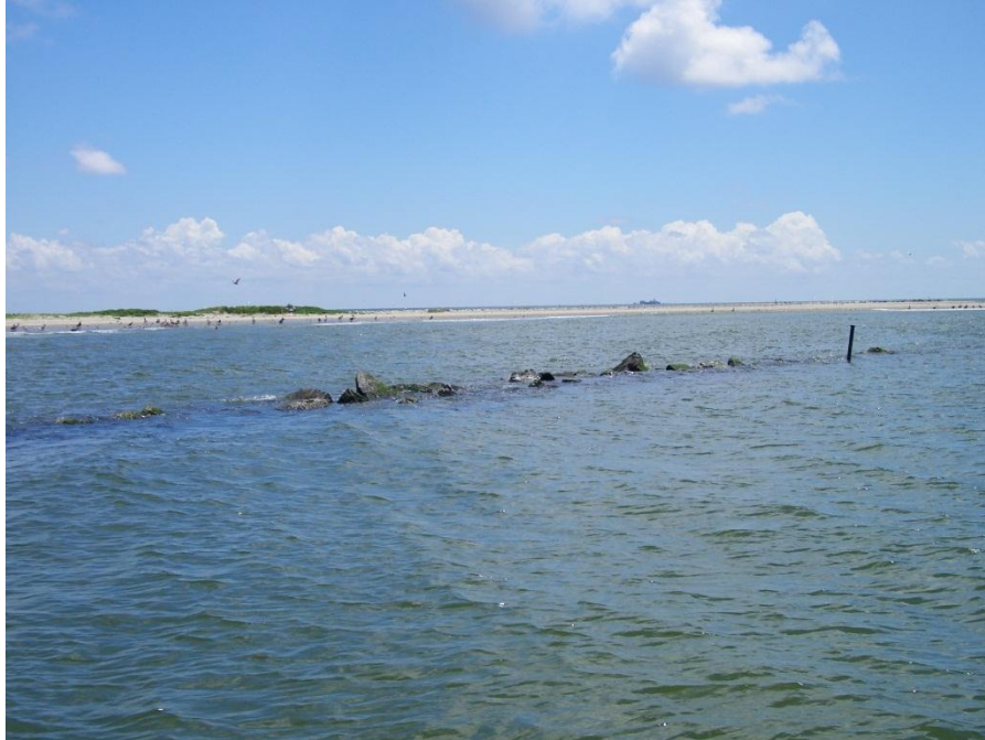
Photo 13: TE-29 breakwater #3 looking north (Raccoon_095). Note low elevation, lack of wave diffraction behind the breakwater, and no evidence of salient formation.
