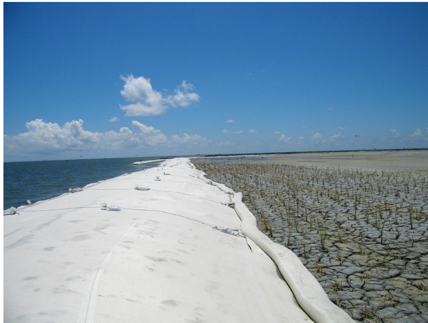
Photo 16: TE-48 marsh creation back dike looking east (Raccoon_131). Note geotextile coverage of the back dike in an attempt to postpone degradation until sediments consolidate and vegetative plantings spread. Also, note geotubes in background as the first attempt to protect the back dike.
