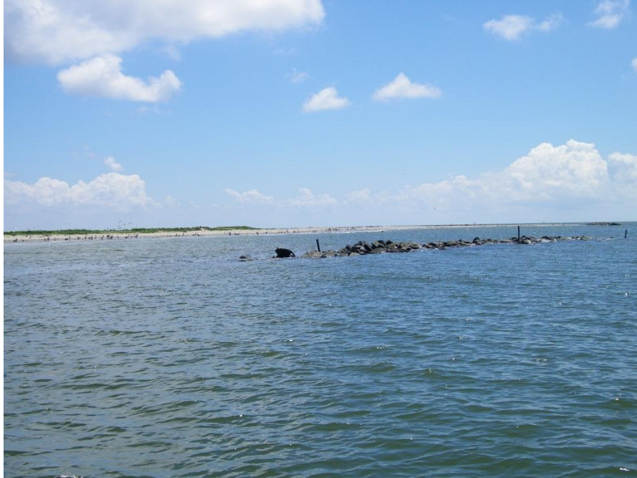
Photo 11: TE-29 breakwater #4 looking northeast (Raccoon_088). Note low elevation, leaning settlement plates, and lack of wave diffraction behind the breakwater.
