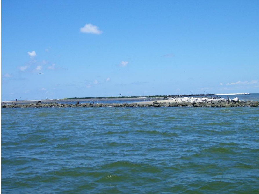
Photo 15: TE-29 breakwater #0 and TE-48 eastern terminal groin looking west (Raccoon_120). Note high elevation and significant sand accumulation along groin.
