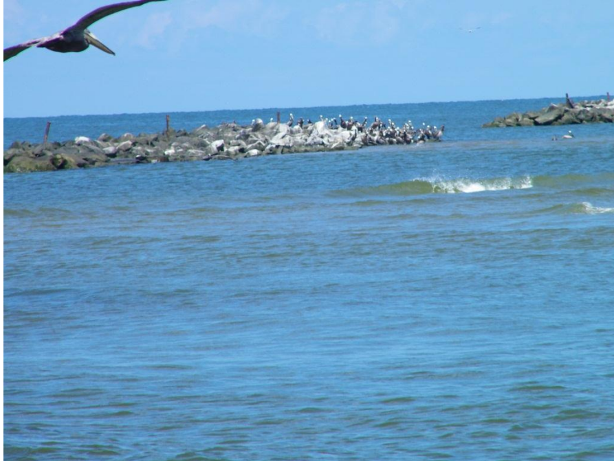
Photo 3: Behind TE-29 breakwater #5 looking west (Raccoon_042). Note higher crest elevation of breakwaters, and wave diffraction from breakwaters and salients.
