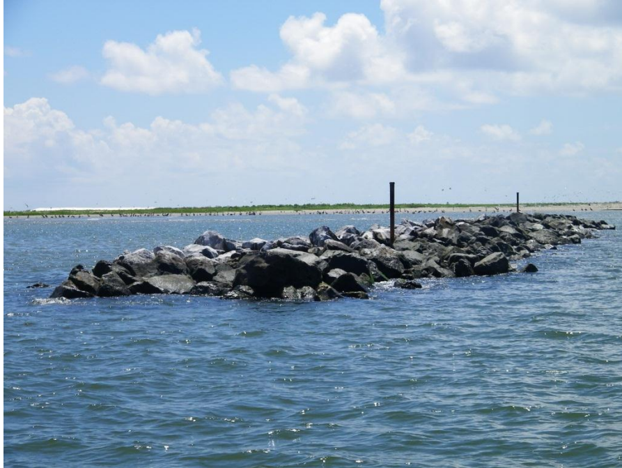
Photo 5: West end of TE-48 breakwater #15 looking west (Raccoon_052). Note high crest elevation of breakwaters, and intact settlement plates.
