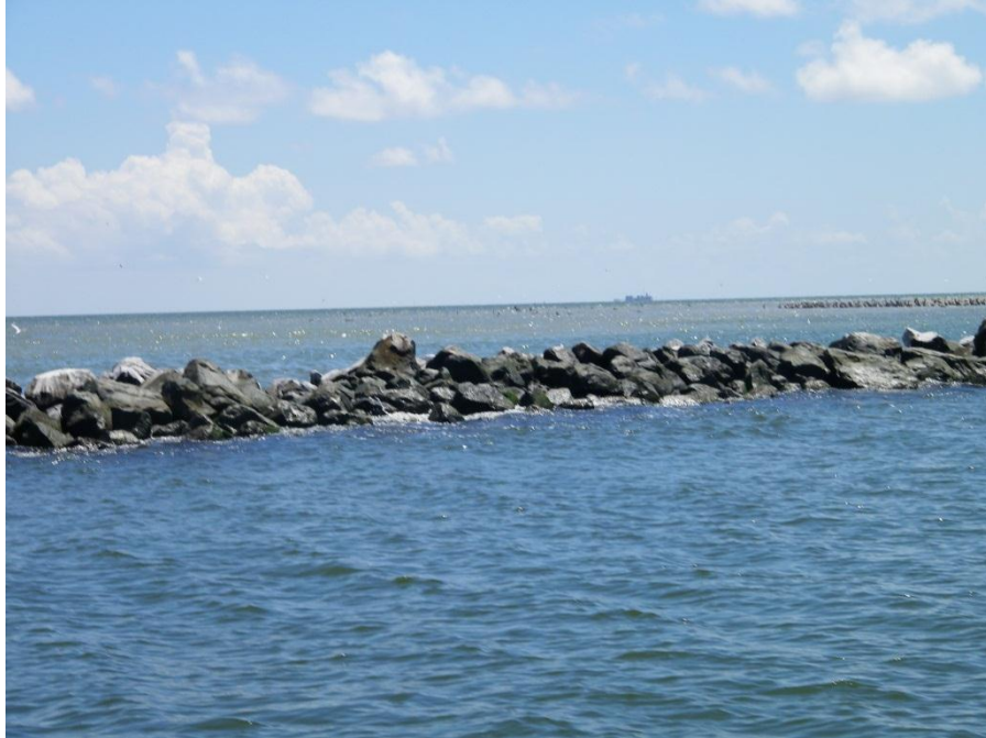
Photo 7: TE-48 breakwater #14 looking north (Raccoon_052). Note breach in background with obvious shallow shoal.
