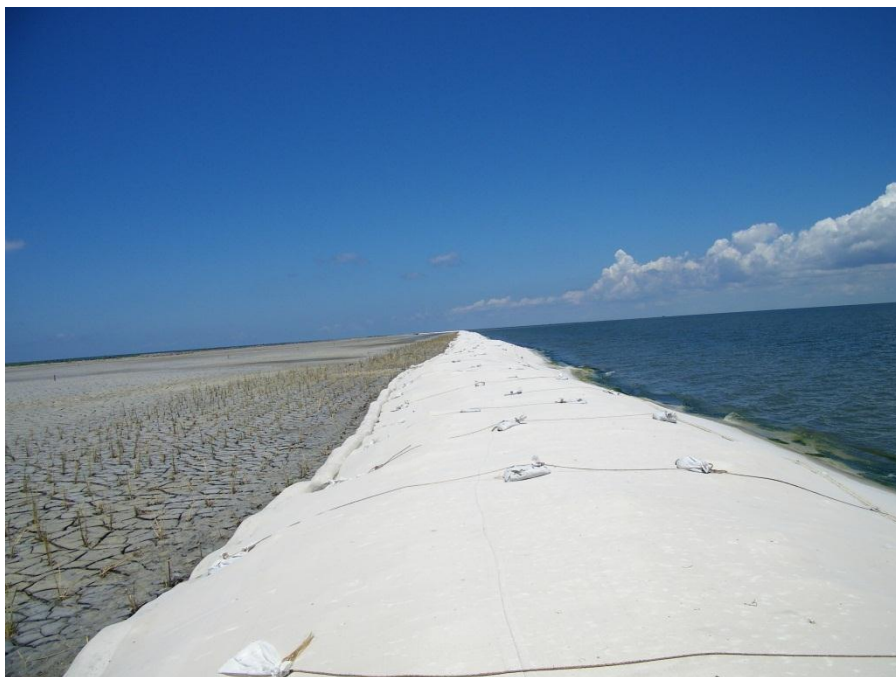
Photo 20: TE-48 marsh creation area back dike looking west (Raccoon_150). Note geotextile cover on dike and first plantings along inside, indicating where contractor could access.
