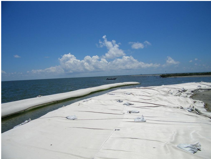
Photo 18: TE-48 marsh creation area back dike looking east (Raccoon_143). Note geo-tubes in as the first attempt to protect the back dike.
