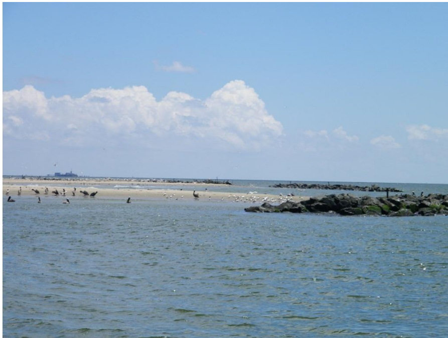
Photo 14: TE-29 breakwaters #2 – 0 and TE-48 eastern terminal groin looking north (Raccoon_098). Note high elevation, significant salient formation.
