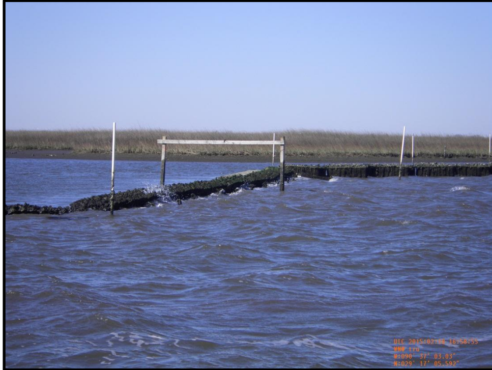
Photo B-7: View of intersection of A-Jacks and ReefBlks along Segment A.
