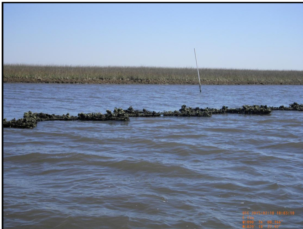
Photo B-18: View of offshore ReefBlk units along Reach E.
