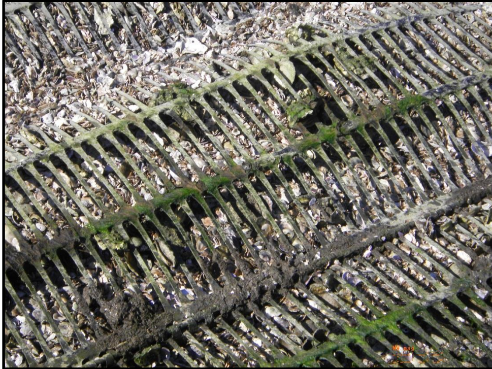
Photo B-3. Southern end of Gabion Mats along Reach Close-up view of the gabion mats and fill material at Reach A.
