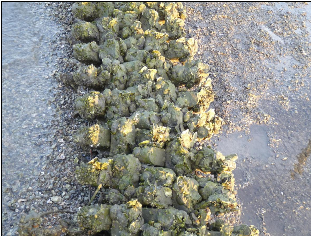
Figure 56. A-Jacks at Reach-B in winter 2014 survey showing underlying geotextile mat with limestone used as a base, and the mixed in pieces of oyster and mussel shells washed up from the bay by waves and from shell chipped off reef populations. Windward (bay side) to the right and leeward (marsh side) to the left.
