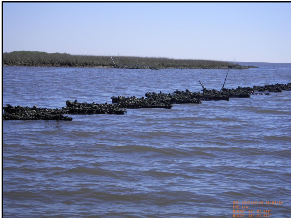
Photo B-20: View of offshore ReefBlk Units along Segment E.
