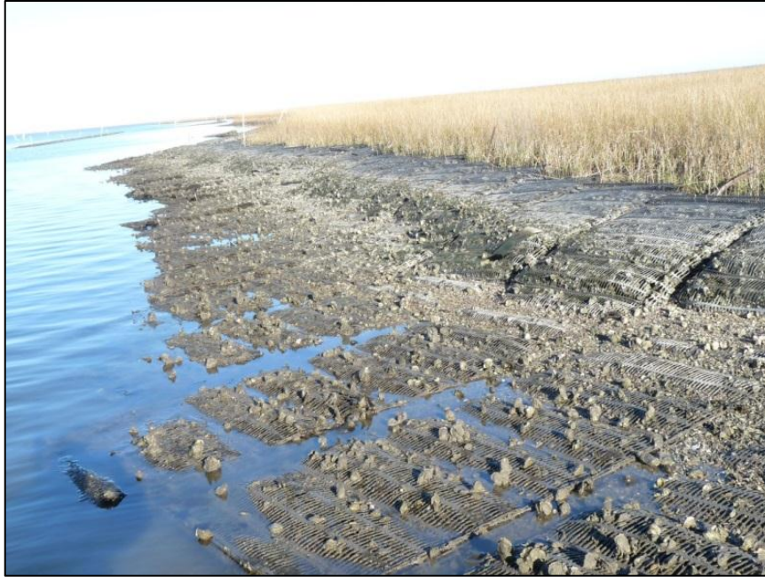
Figure 46. Photo showing the distribution of oysters and emergent reef across Gabion Mats at Reach- B during the winter 2014 survey, seven years post construction.
