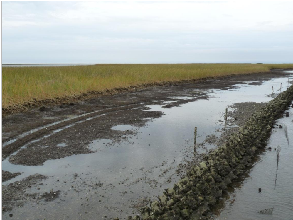
Figure 30. Boat dual-propeller tracks remain behind A-Jacks at Reach-E showing how activities associated with laying oil boom impacted marsh shoreline. Winter 2010 photo several months after crews had removed the oil boom from the marsh. Similar tracks observed at Reach-E behind ReefBlks.
