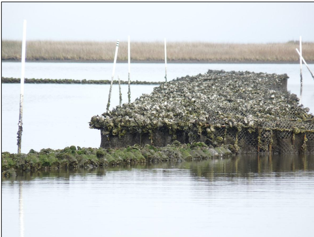
Figure 60. Reach B showing tops of ReefBlk with oysters colonized on the iron rebars winter 2014. Note the absence of oysters and shell below the top rebars. The A-Jacks tie-ins are in the foreground, which show how the tops of the bay-facing arms had little recruitment.
