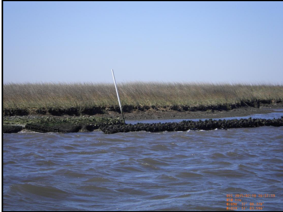
Photo B-5: Gabion Mats intersect with A-Jacks along Reach A.
