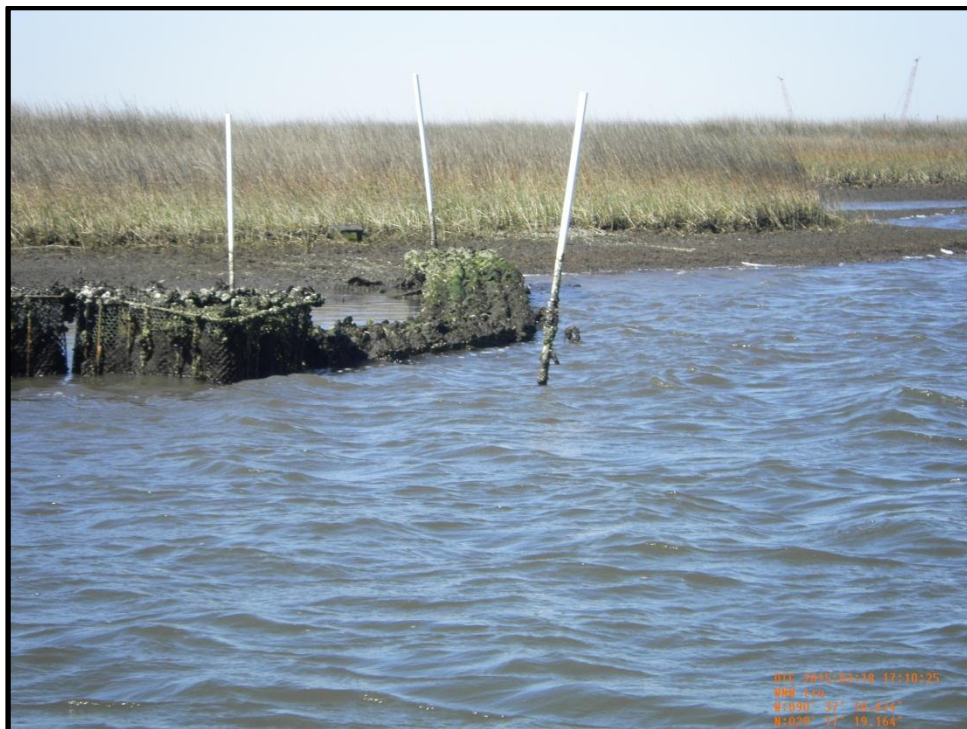
Photo B-14: View of ReefBlks and A-Jack tie-in to shoreline along Segment B.
