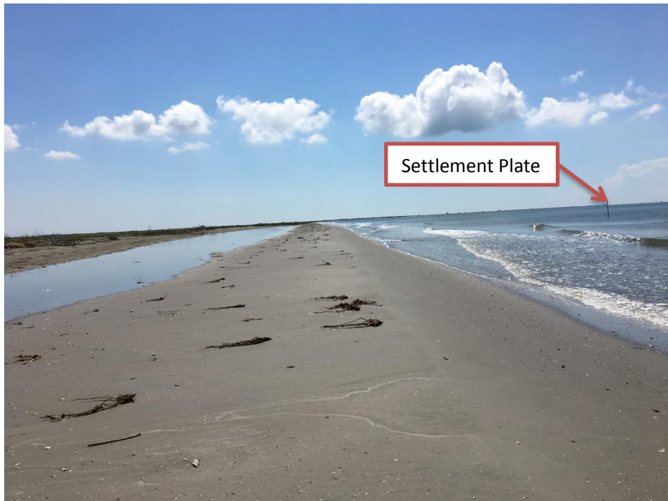
Photo 10: View of beach erosion, looking east. Note: settlement plate installed on the center of the dune is currently in the Gulf.
