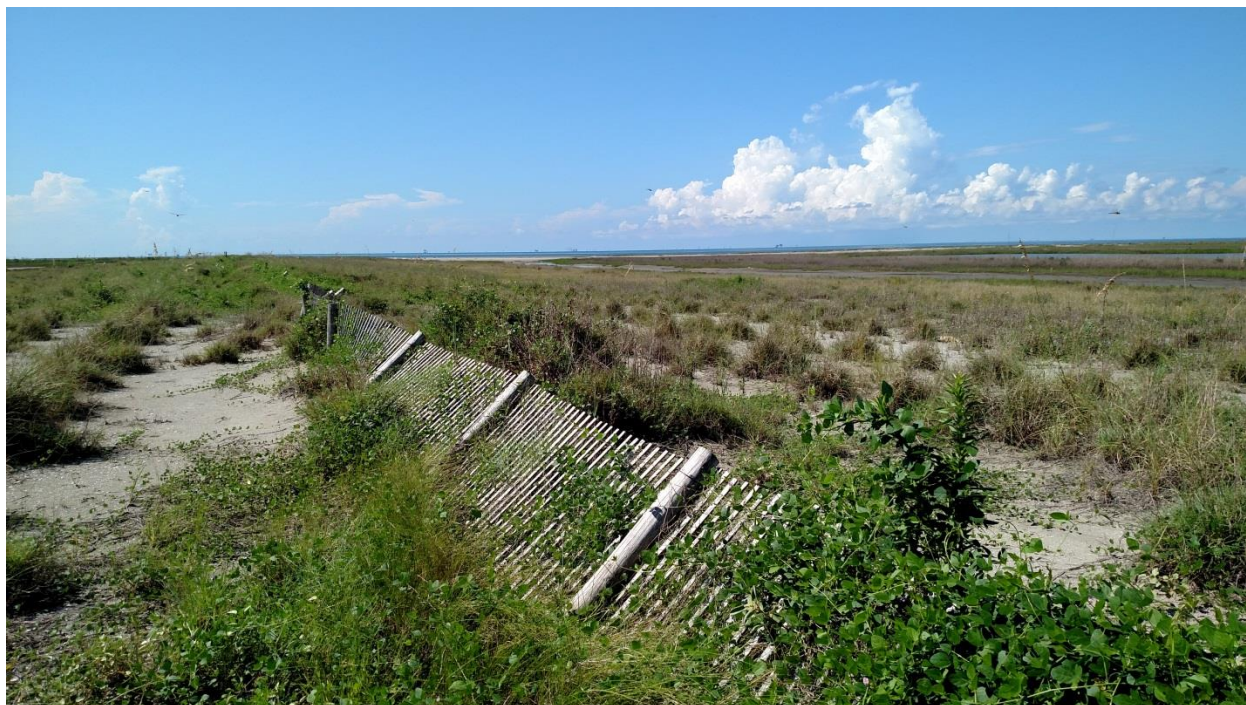
Photo 5: View of successful vegetative planting & sand fence, looking south.
