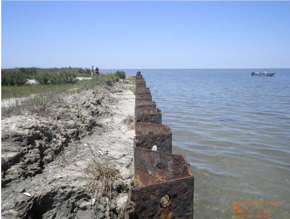
Photo 2: View of sheet pile plug in northern containment dike, looking west.
