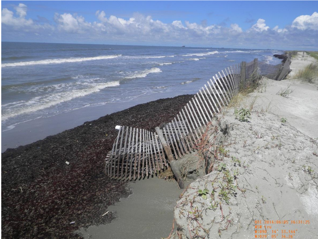
Photo 17: View of the damaged sand fence along the beach dune, looking southwest
