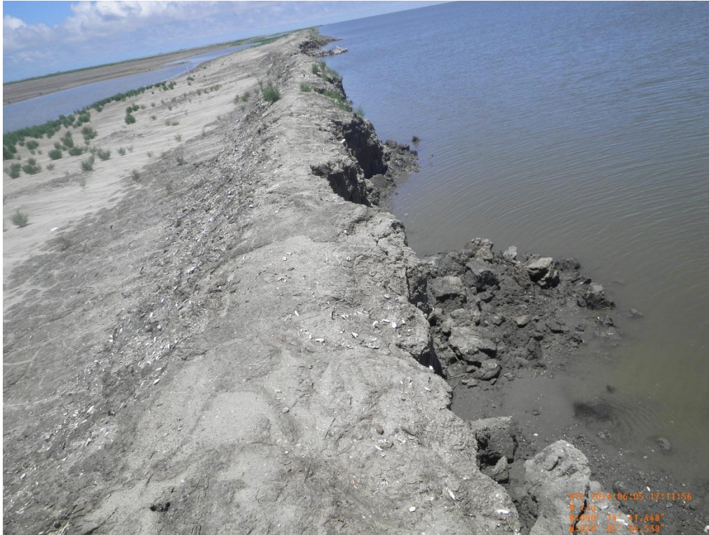
Photo 25: Close up of the erosion found on the northern containment dike
