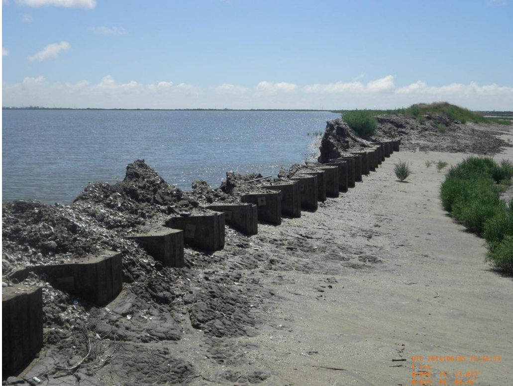
Photo 1: View of sheetpile plug in northern containment dike
