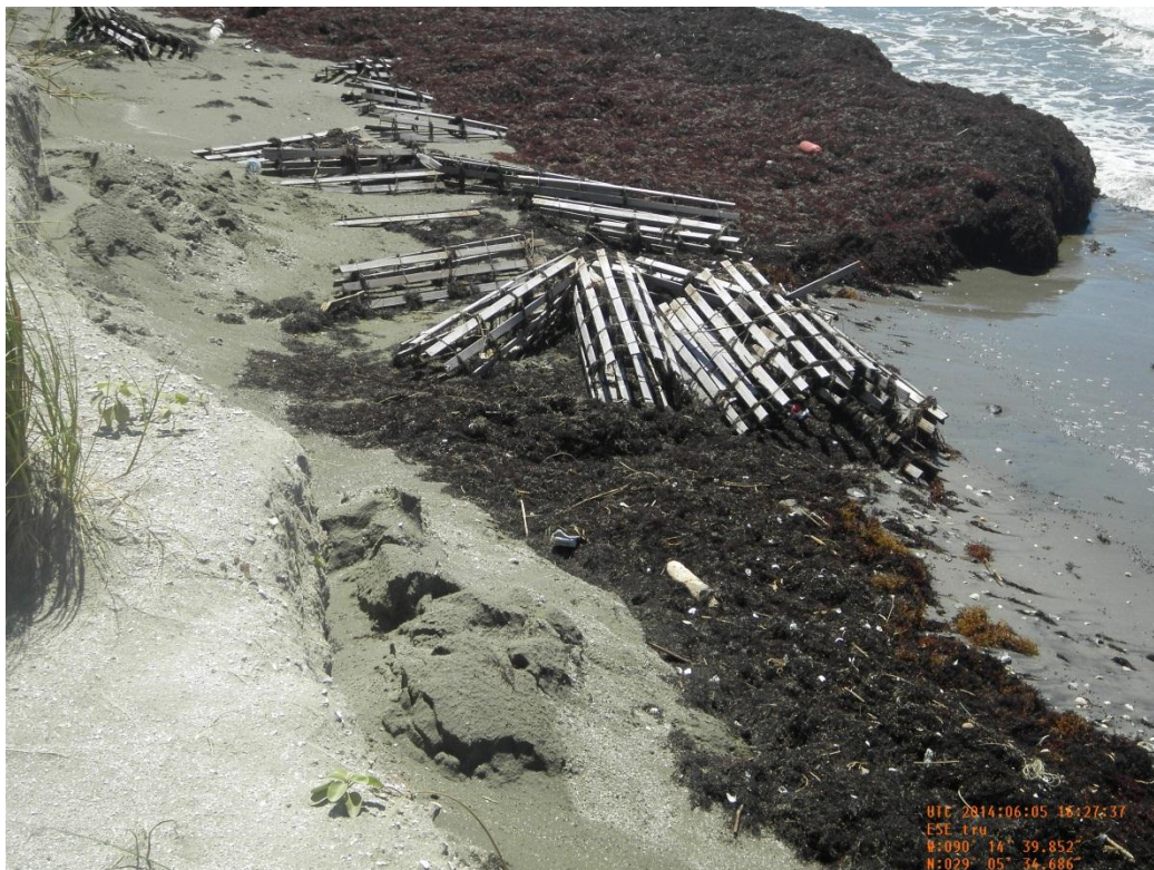
Photo 16: Destroyed sand fencing due to the erosion of the beach dune
