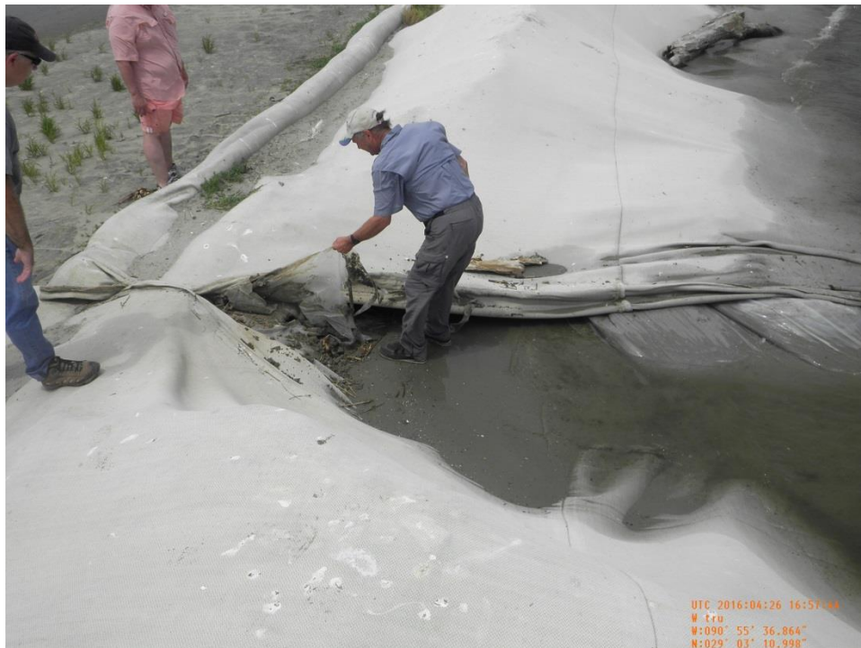
Photo 33 (0180) – View of a new tear in geotextile fabric and erosion near Sta. 25+00
