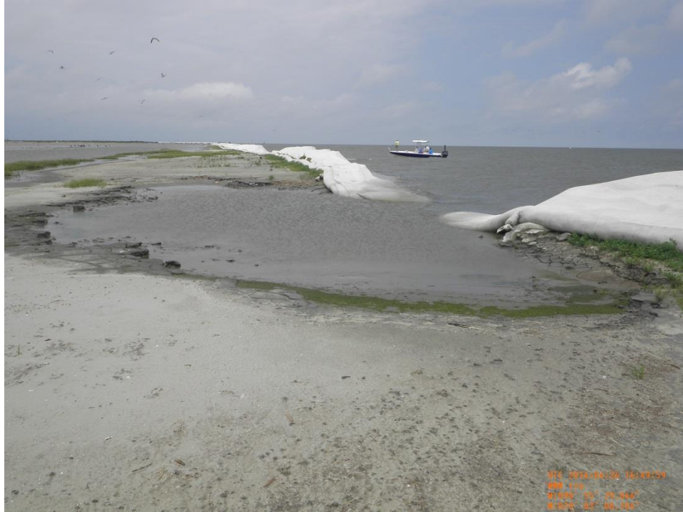
Photo 30 (0166) Breach through geotextile fabric near Sta. 20+00
