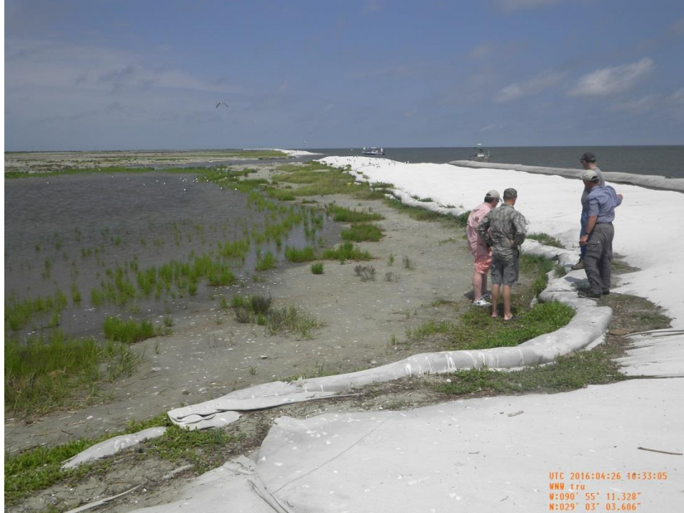
Photo 18 (0120) – View of geotextile fabric and geotubes along back containment dike near Sta. 5+00 looking west
