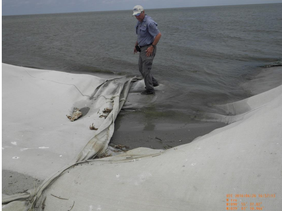
Photo 32 (0177) – View of a new tear in geotextile fabric and erosion near Sta. 25+00.
