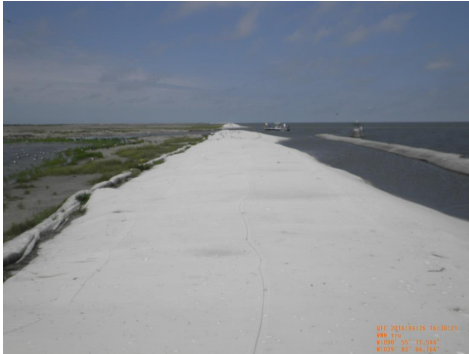
Photo 20 (0108) – View of geotextile fabric along back containment dike near Sta. 1+00 looking west
