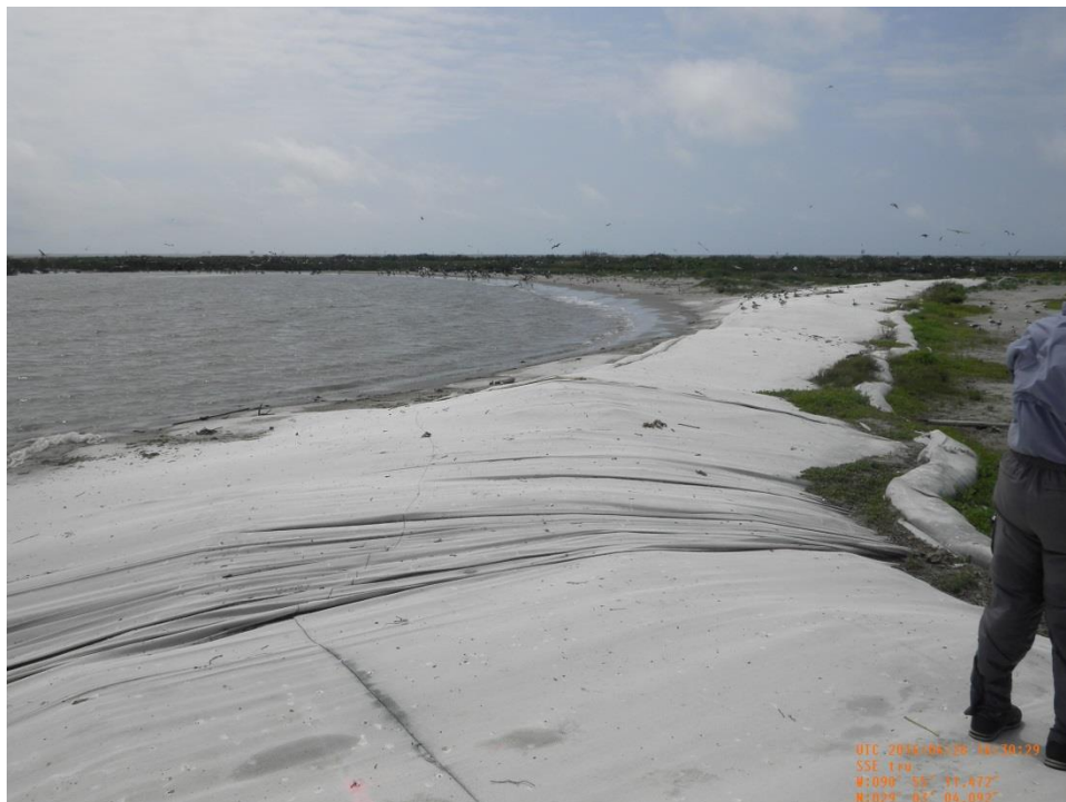
Photo 19 (0109) – View of geotextile fabric and geotube along back containment dike near Sta. 5+00 looking south east
