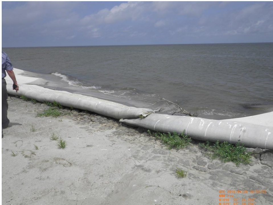
Photo 31 (0173) – View of geotextile fabric tear near Sta. 23+00 and erosion of containment.
