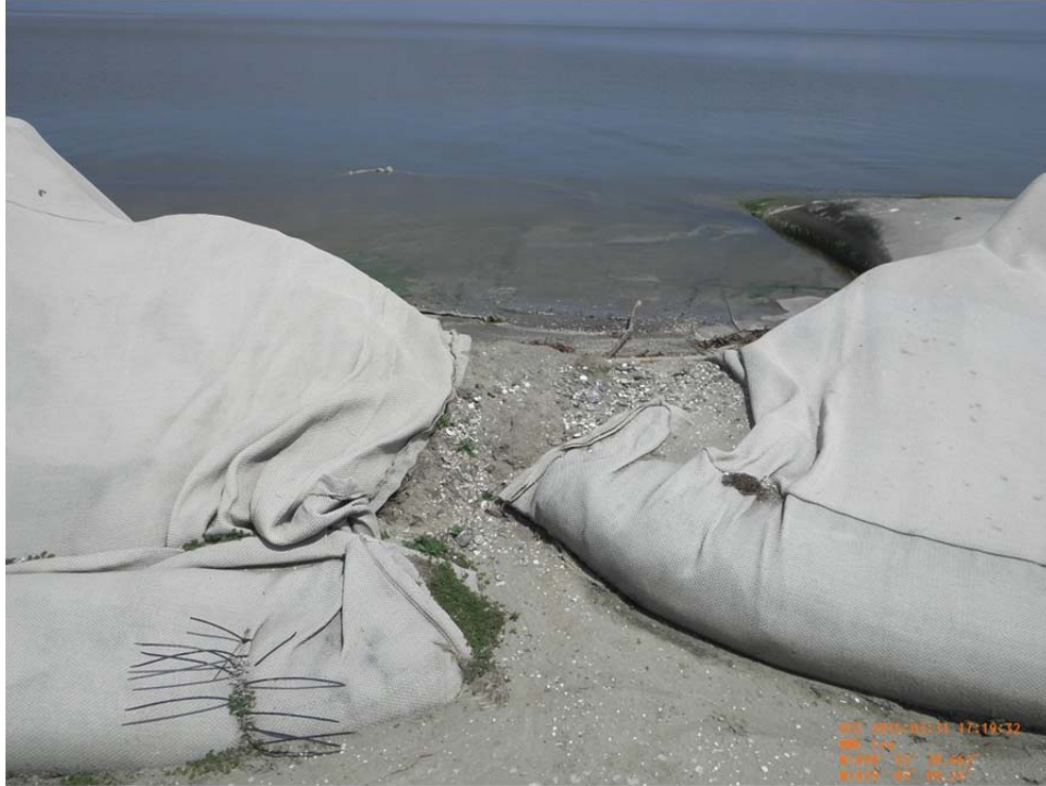
Photo 17: (1284) - View of tear in geotextile fabric and erosion of containment near Sta. 17+00.
