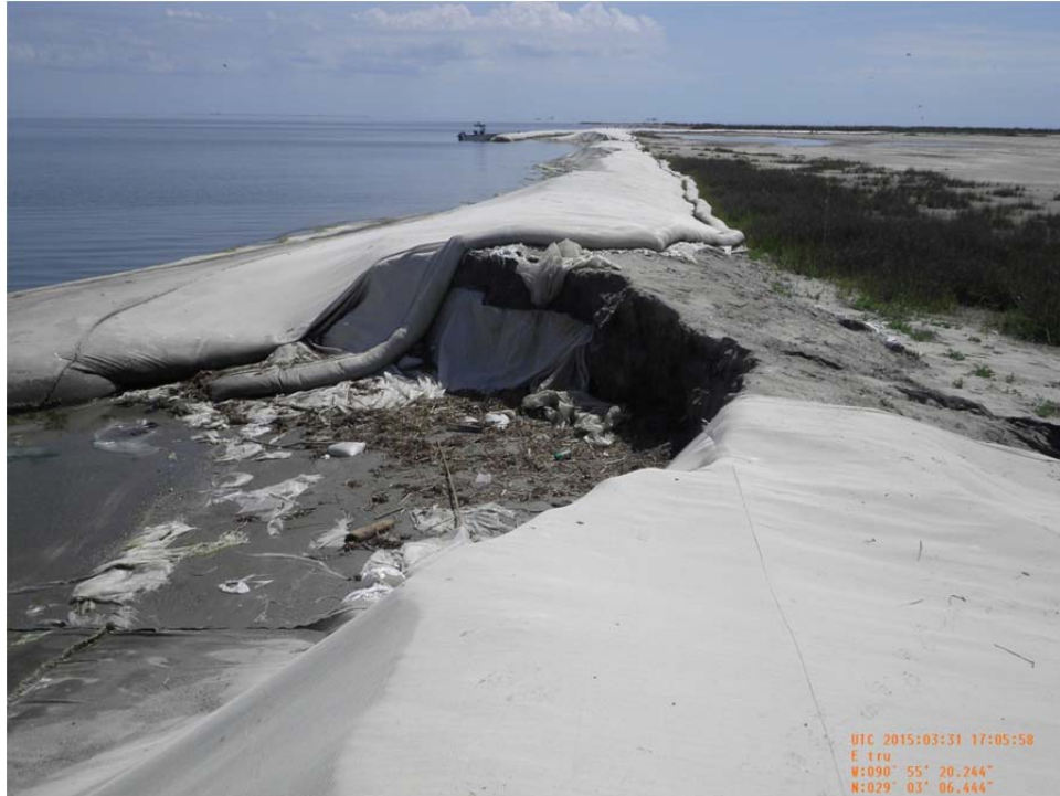
Photo 11: (1260) – View of torn geotextile fabric and erosion near Sta. 8+00.
