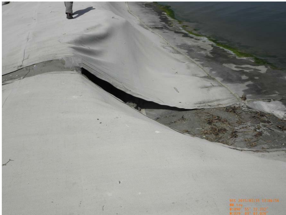
Photo 12: (1262) – View of torn geotextile fabric along back containment near Sta. 10+00
