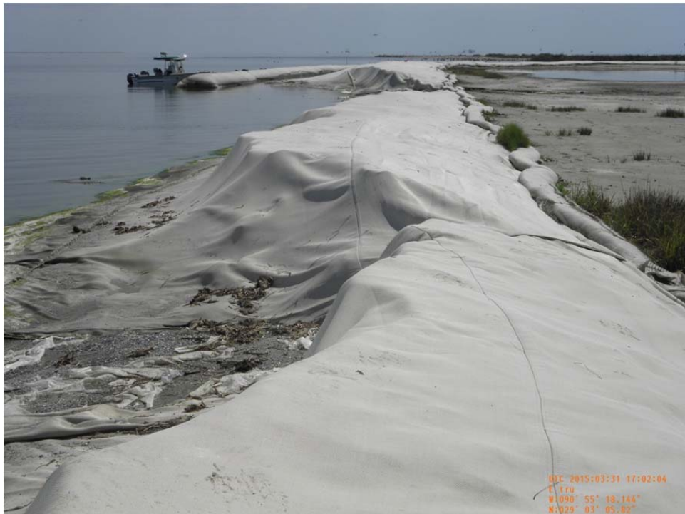
Photo 10: (1253) – View of geotextile fabric tear near Sta. 7+00 and erosion of containment.
