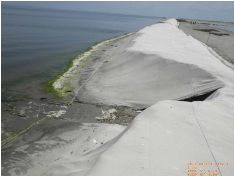
Photo 22: (1298) – View of geotextile fabric along containment near Sta. 22+00 looking east.
