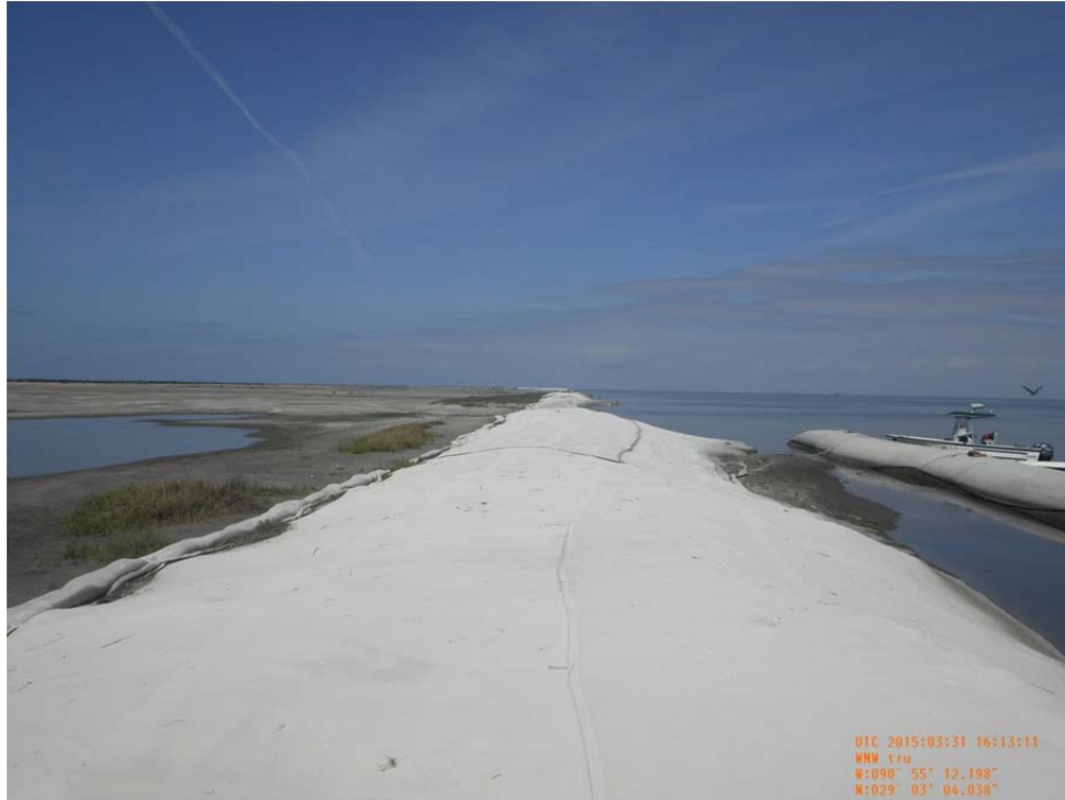
Photo 3: (1232) – View of geotextile fabric along back containment dike near Sta. 1+00 looking west.
