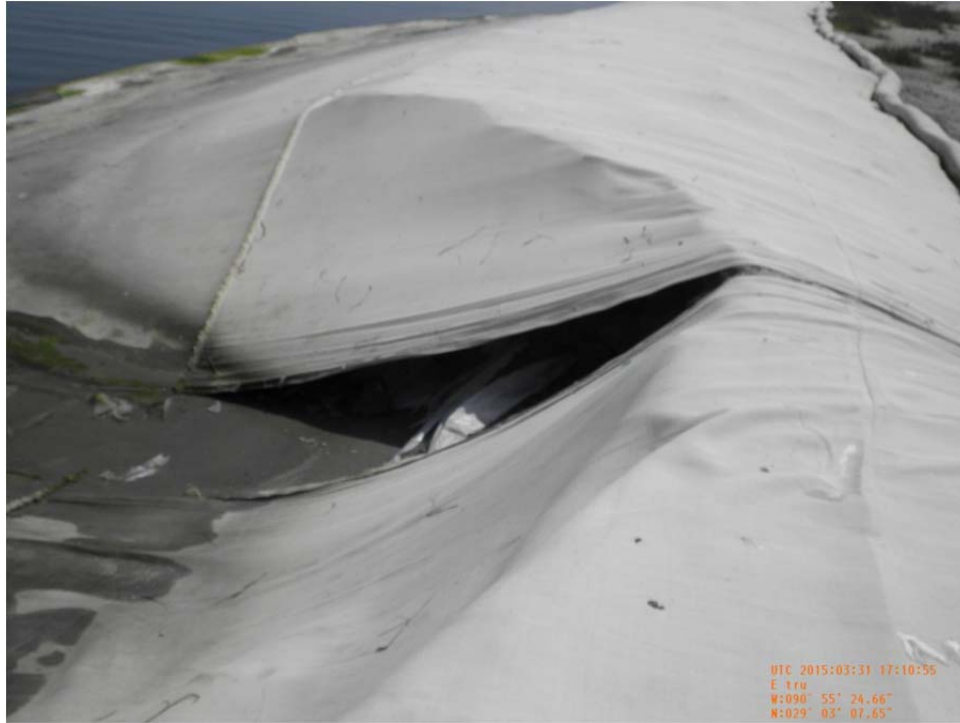
Photo 13: (1270) - View of torn geotextile fabric and erosion along back containment near Sta. 13+00.
