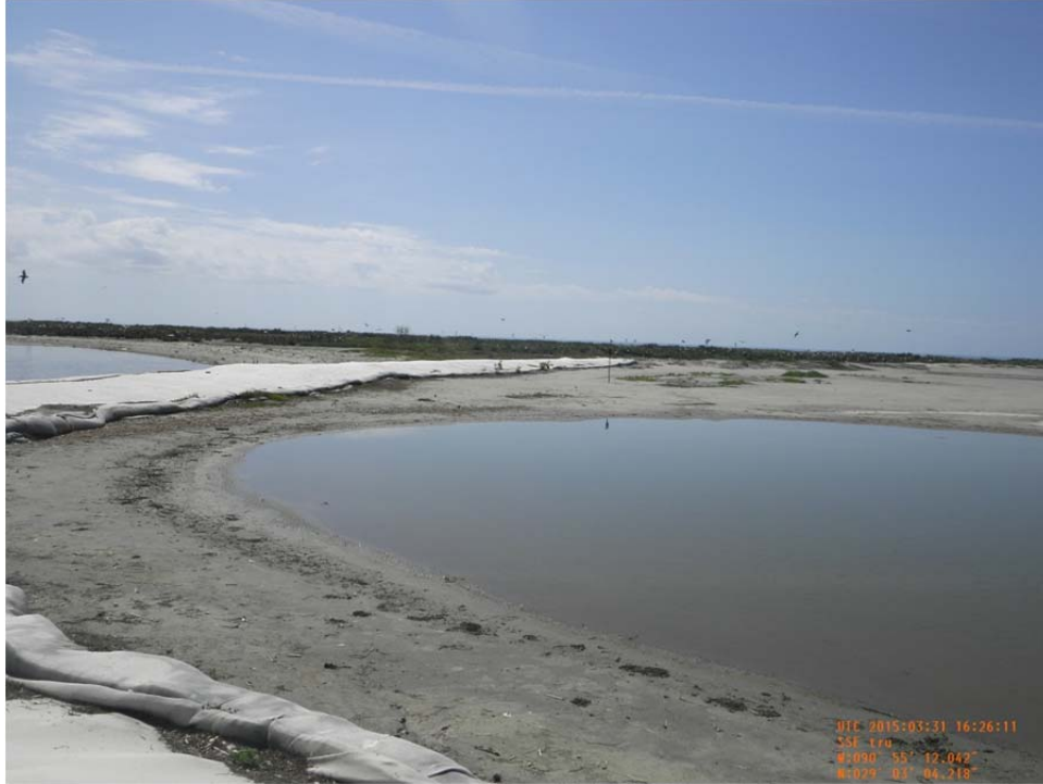
Photo 5: (1235) – View of marsh fill area and geotextile fabric containment from Sta. 1+00 looking south.
