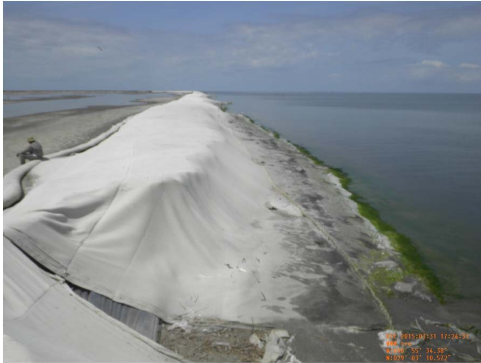
Photo 21: (1294) – View of geotextile fabric along containment near Sta. 22+00 looking west.
