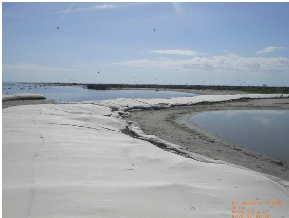
Photo 2: (1230) – View of geotextile fabric and geotube along back containment dike near Sta. 5+00 looking east.
