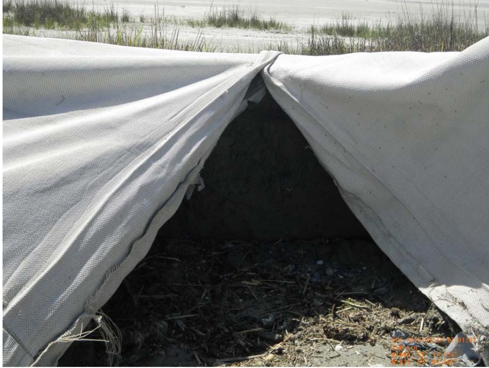
Photo 9: (1249) – Tear in geotextile fabric near Sta. 7+00
