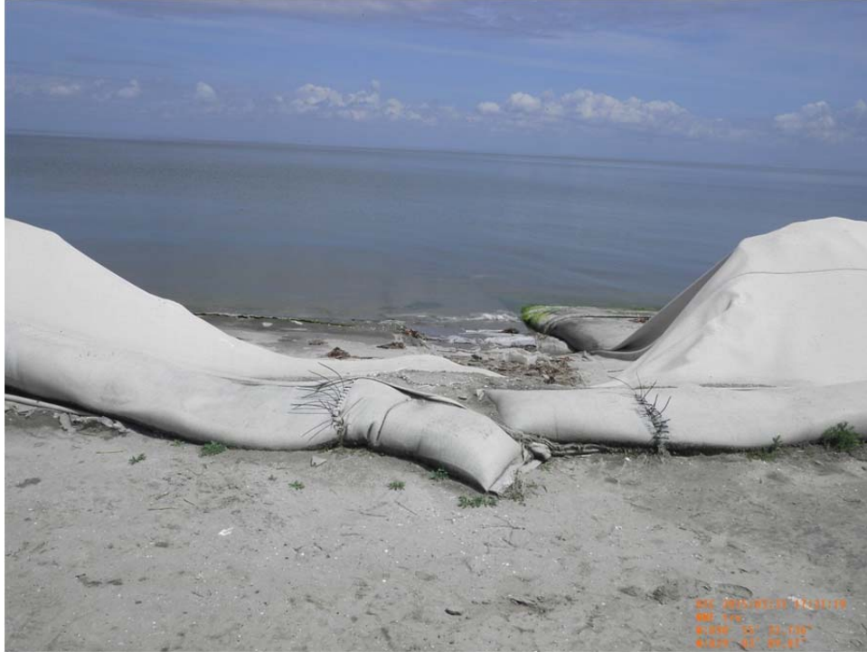
Photo 19: (1286) – View of large breach in containment near Sta. 20+00.
