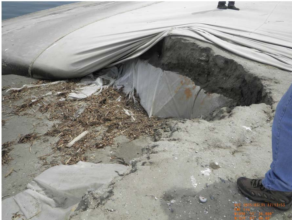
Photo 16: (1278) - View of tear in geotextile fabric along containment near Sta. 15+00.
