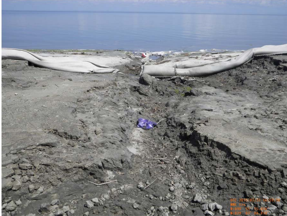
Photo 7: (1245) – View of erosion along the geotextile fabric along containment near Sta. 4+00.
