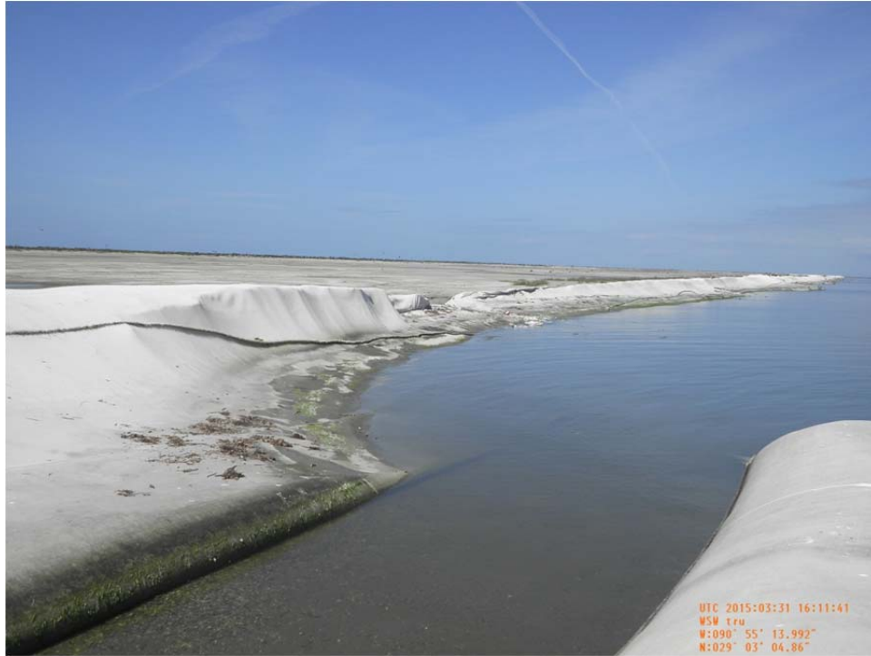
Photo 1: (1228) – View of geotextile fabric and geotubes along back containment dike near Sta. 5+00 looking west.
