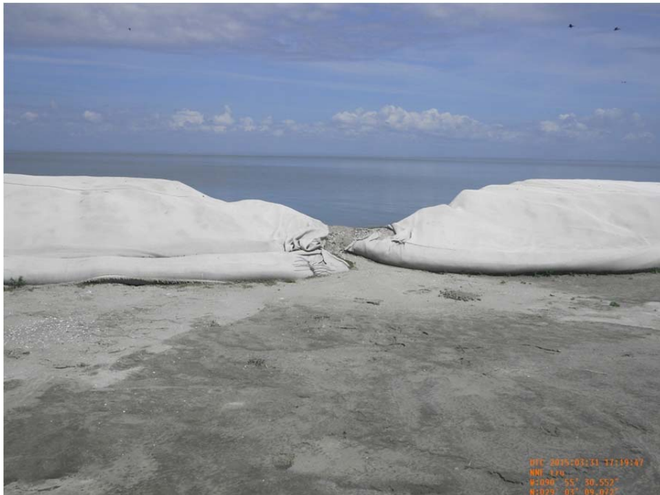
Photo 18: (1285) - View of tear in geotextile fabric and erosion of containment near Sta. 17+00.
