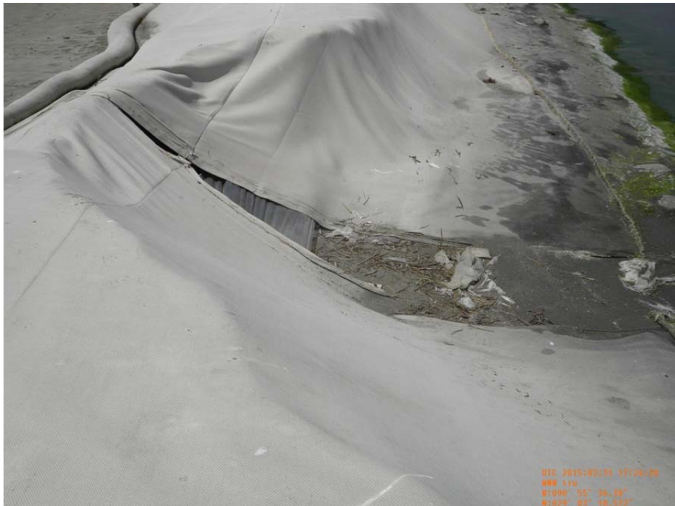
Photo 20: (1292) – View of tear in geotextile fabric along containment near Sta. 22+00.
