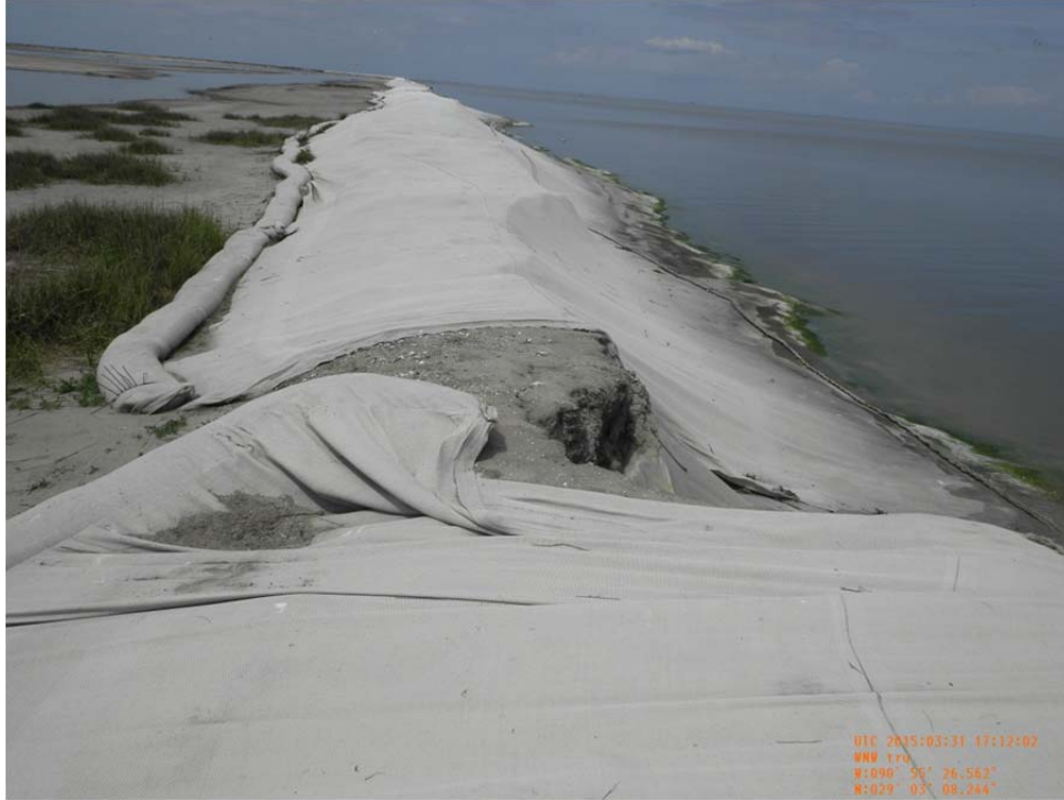
Photo 15: (1273) - View of tear in geotextile fabric along containment near Sta. 15+00.
