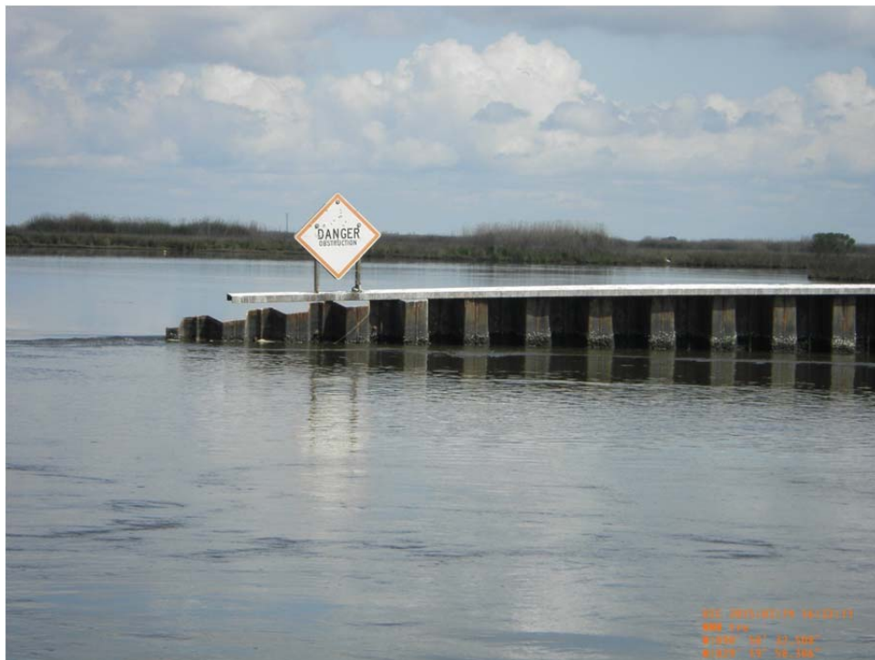
Photo 18: view of the center section of the damaged sheet pile along Sheetpile Plug No.2.
