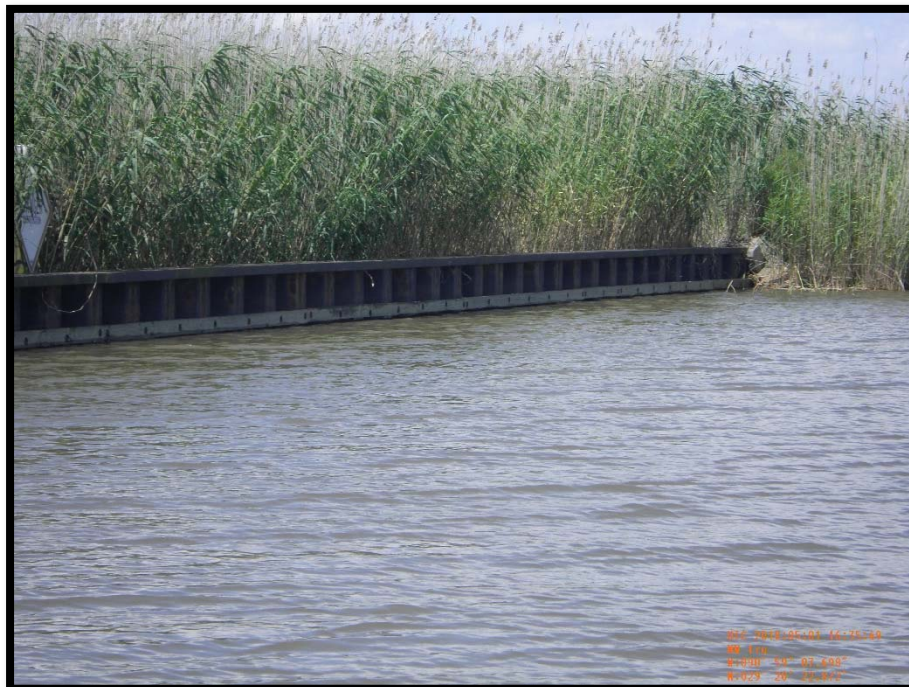
Photo No.20 – View of Steel Sheetpile Plug No.1 and bank tie-in on west side of structure located along Y-Canal east of Lake Pagie.
