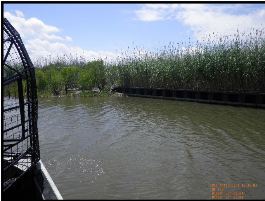
Photo No.22 – View of Steel Sheetpile Plug No.1 and bank tie-in on east side of structure located along Y-Canal east of Lake Pagie.
