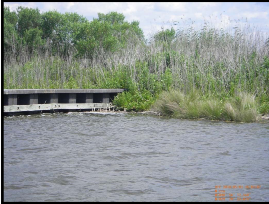
Photo No. 11 - View of the east bank tie-in and articulated mats of Steel Sheetpile Plug No.3
