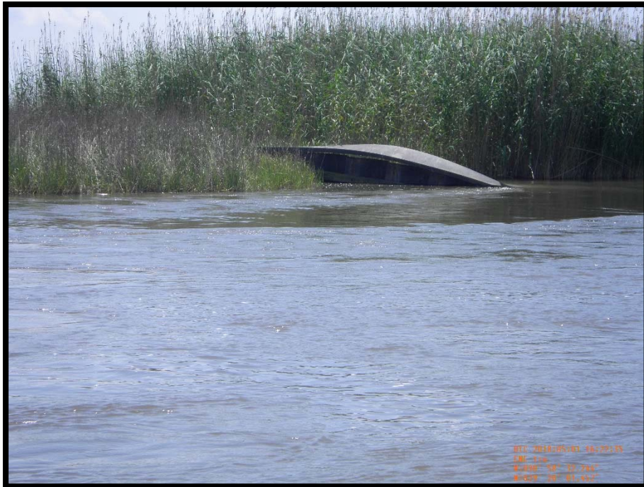
Photo No.18 – View of damaged steel sheetpile section and east bank tie-in of Sheetpile Plug No.2.
