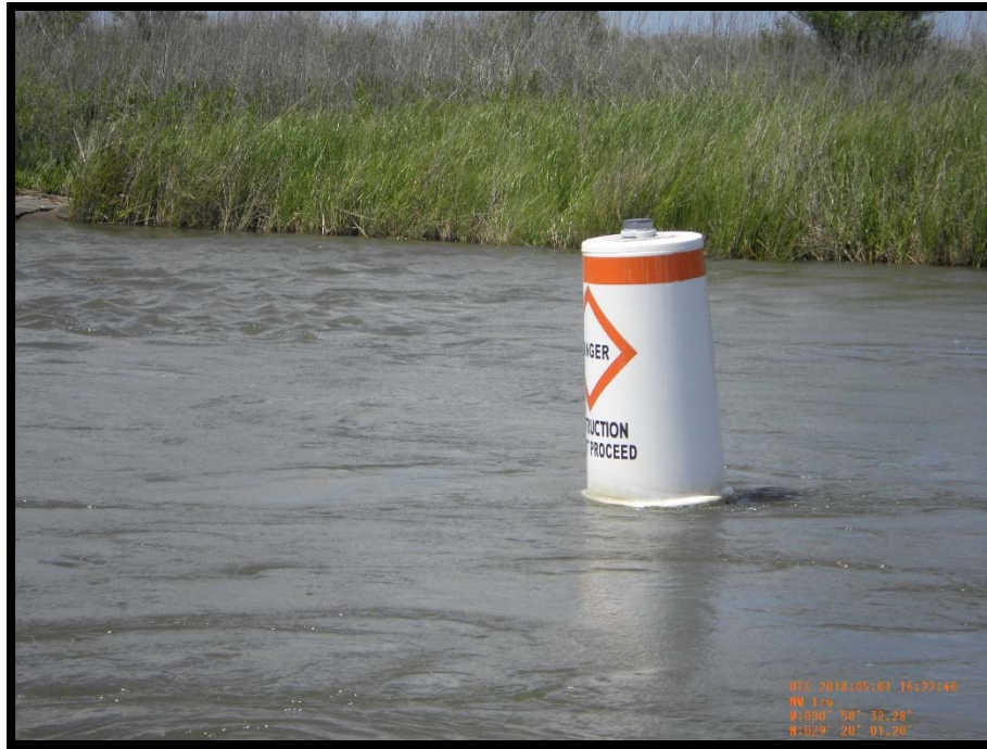
Photo No. 19 – View of floating/lighted buoy installed on both sides of damaged Sheetpile Plug No.2. Two (2) buoys were installed on both sides of the structure.
