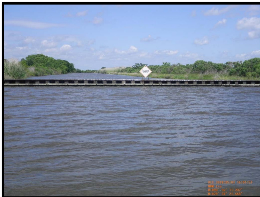
Photo No.10 – View of steel Sheetpile Plug No 3 located at the end of an existing channel along the south bank of Raccourci Bay.
