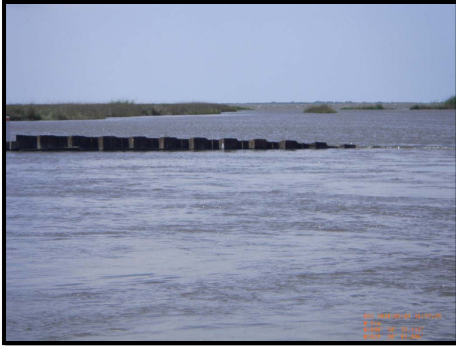
Photo No.17 – View of damaged center section of Steel Sheetpile Plug No. 2
