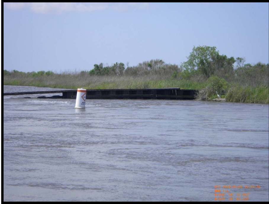
Photo No.15 – View of west bank tie-in and damaged sheet pile section and floating/lighted buoy of Steel Sheetpile Plug No. 2.
