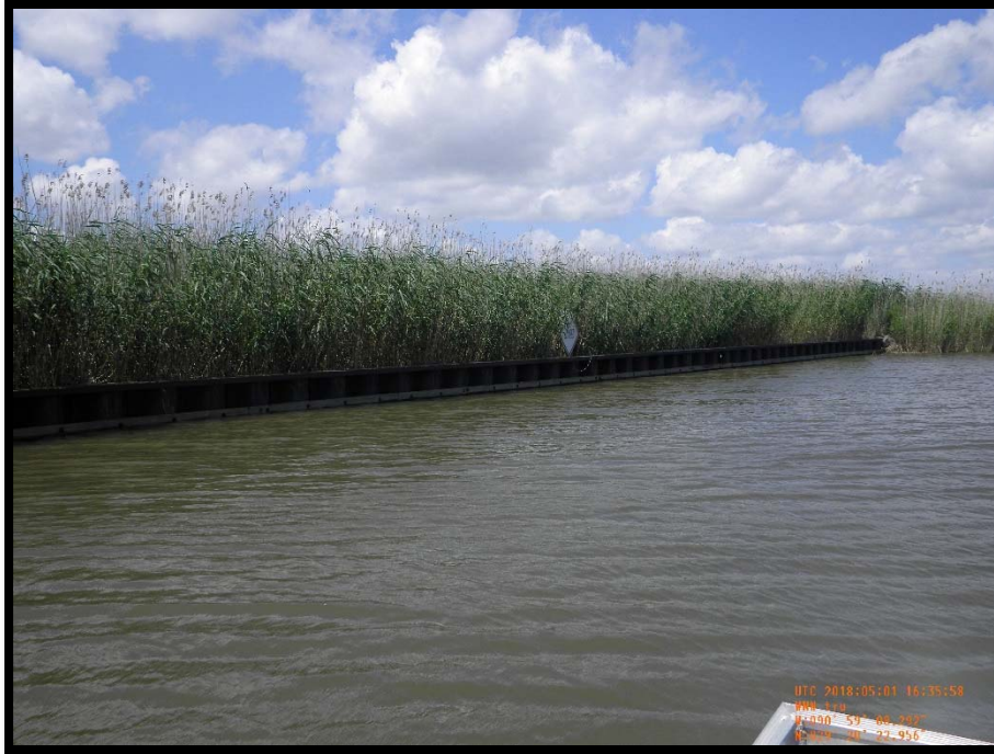
Photo No.21 – View of Steel Sheetpile Plug No.1 located along Y-Canal east of Lake Pagie.
