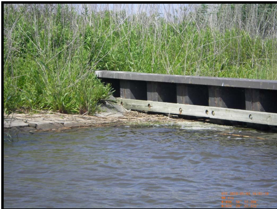
Photo No. 12 - View of the west bank tie-in and articulated mats of Steel Sheetpile Plug No.3
