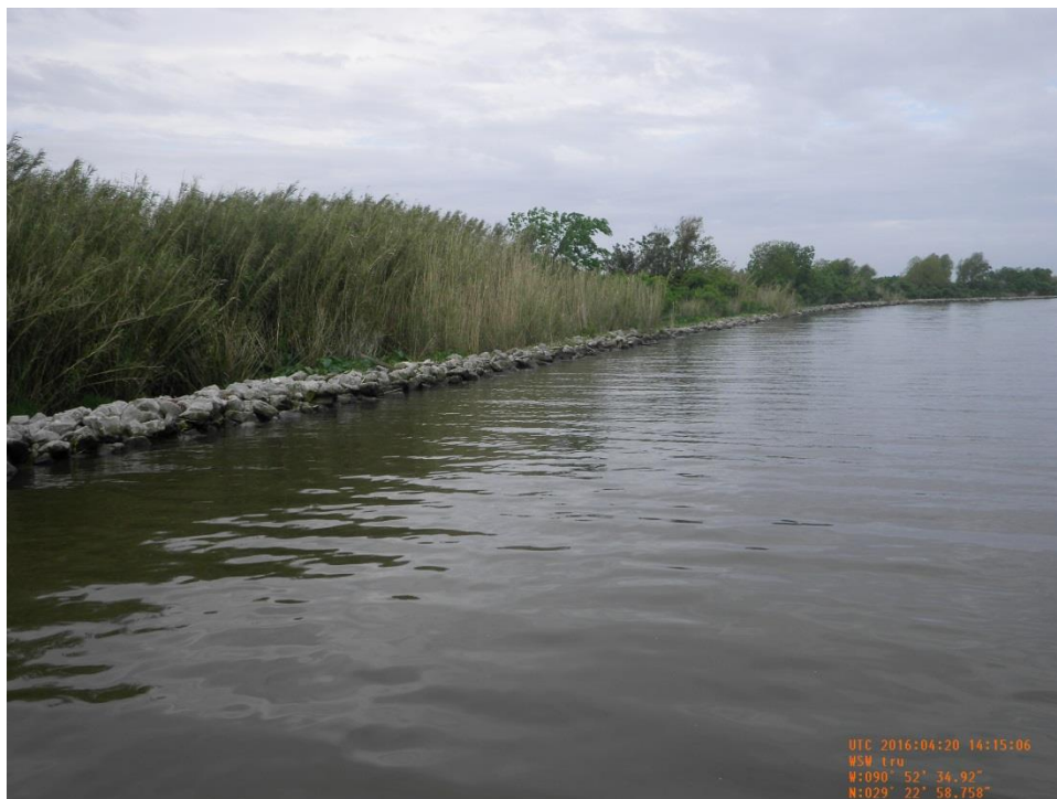
Photo 2: View of earthen embankment and rock revetment along south bank of Bayou Decade near Sta. 80+00 looking westward.
