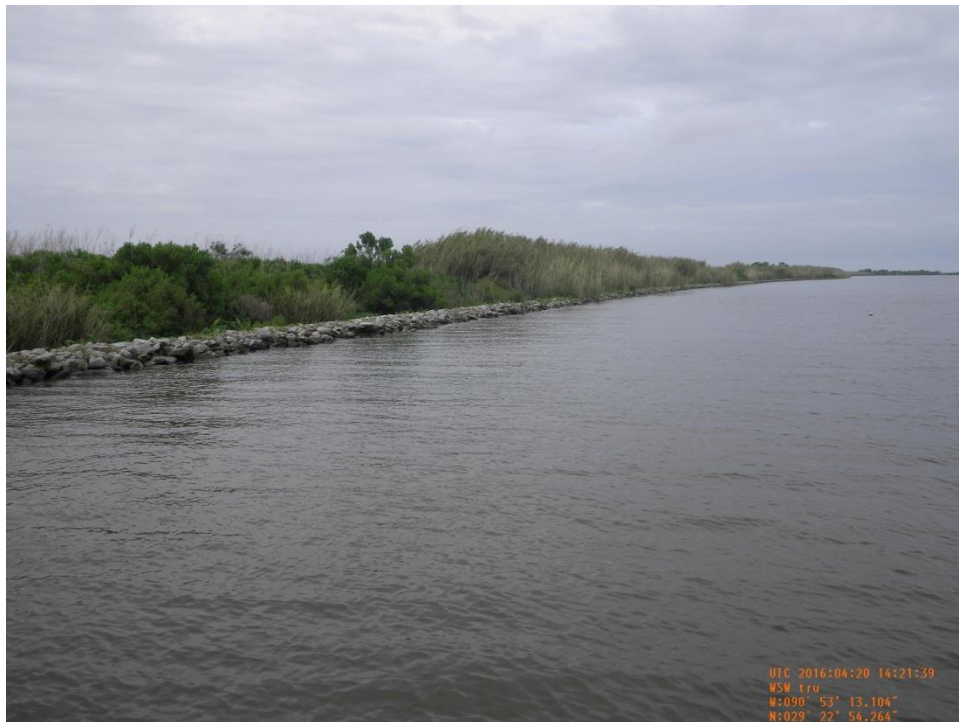
Photo 4: View of earthen embankment and rock revetment along the south bank of Bayou Decade near Sta. 46+00 looking westward.
