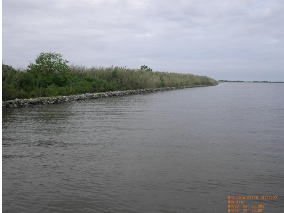
Photo 5: View of earthen embankment and rock revetment on the south bank of Lake Decade near Sta. 36+00 looking westward.
