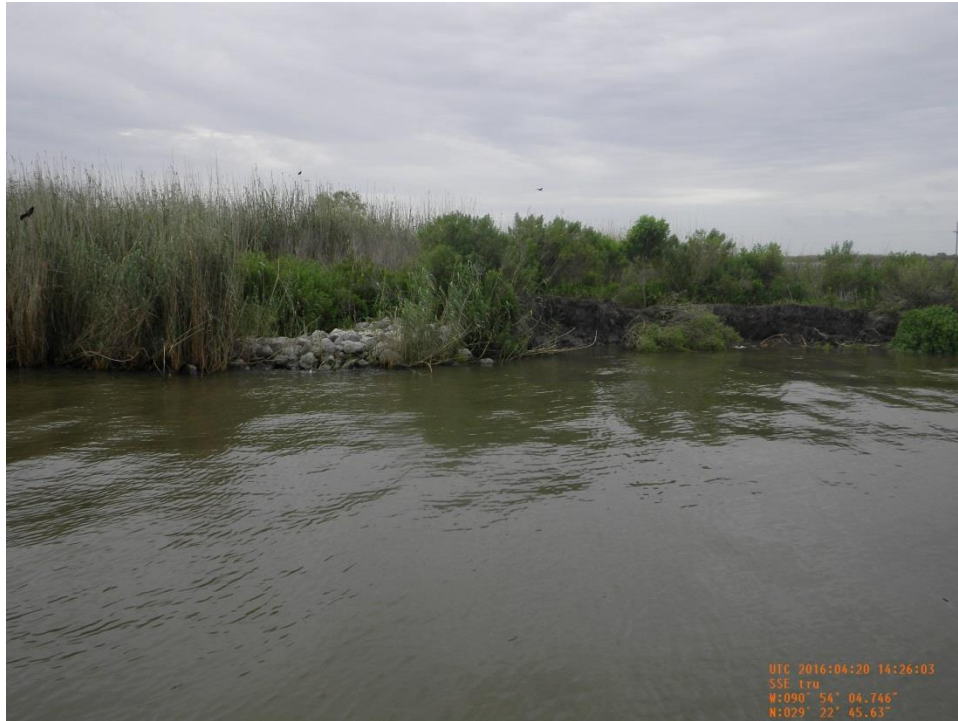
Photo 11: View of earthen embankment and rock revetment on the west end (Sta. 0+10) of the South Lake Decade.
