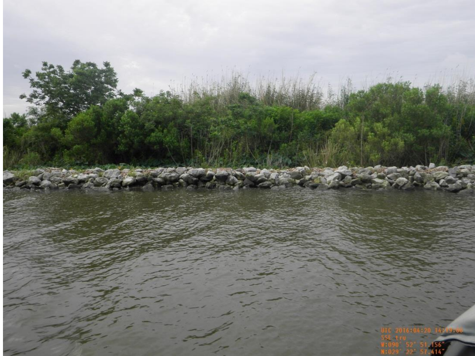
Photo 3: View of earthen embankment and rock revetment along south bank of Bayou Decade near Sta. 66+00.
