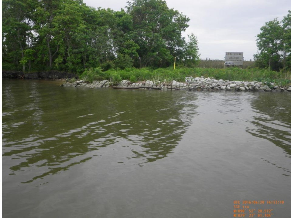
Photos 1: View of earthen embankment and rock revetment at east end of project along south bank of Bayou Decade near Sta. 86+00.
