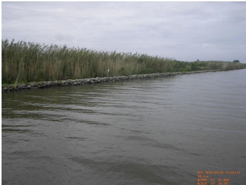
Photo 6: View of earthen embankment and rock revetment on the south bank of Lake Decade near Sta. 26+00 looking westward.
