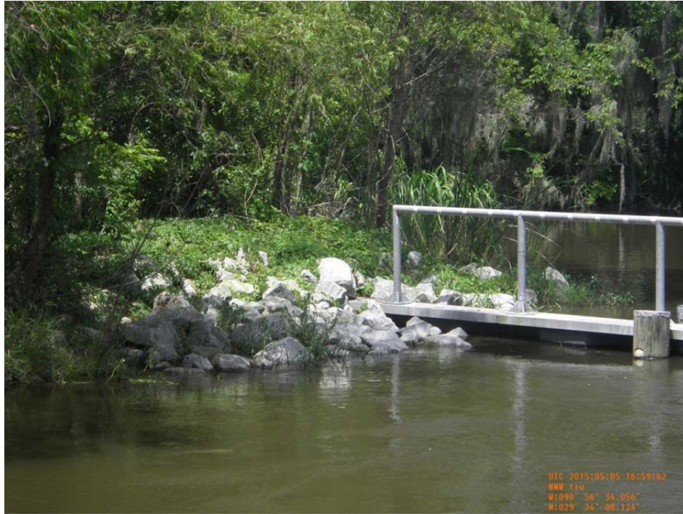
Photo 11: View of steel sheetpile tie-in to bank and rock riprap protection on the south side of the structure.
