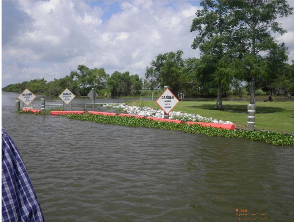
Photo 7: View of steel sheetpile weir with flapgates, rock bank protection and floating debris barrier along the north bank of Brady Canal near the Apache Camp.
