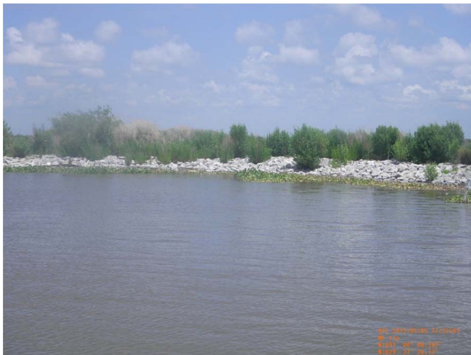
Photo 16: View of rock shoreline revetment on the north bank of Bayou Decade northeast of Structure No.4 along Reach 2 near Sta. 04+00.
