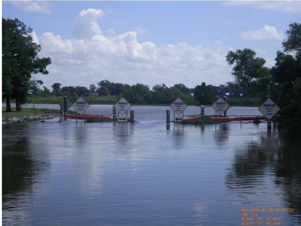
Photo 9: Over all view of the steel sheetpile structure, floating debris barrier, warning signs and rock bank protection across Brady Canal at Bayou Penchant.
