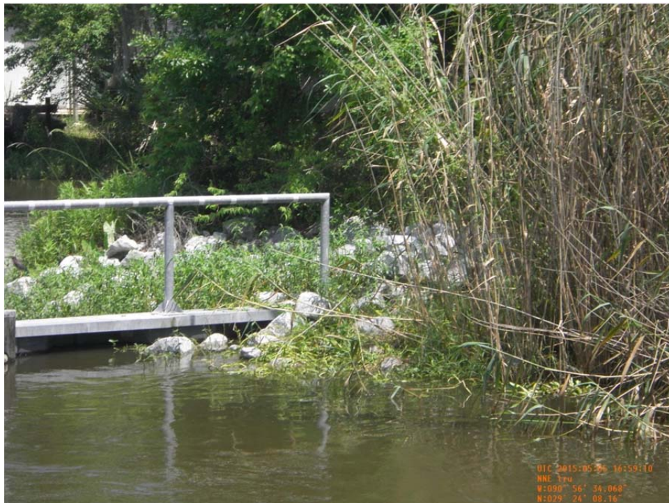
Photo 12: View of steel sheetpile tie-in to bank and rock riprap protection on the north side of the structure.
