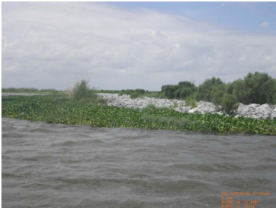
Photo 14: View of rock revetment along the north bank of Bayou Decade near Sta. 35+00 of Reach 3.
