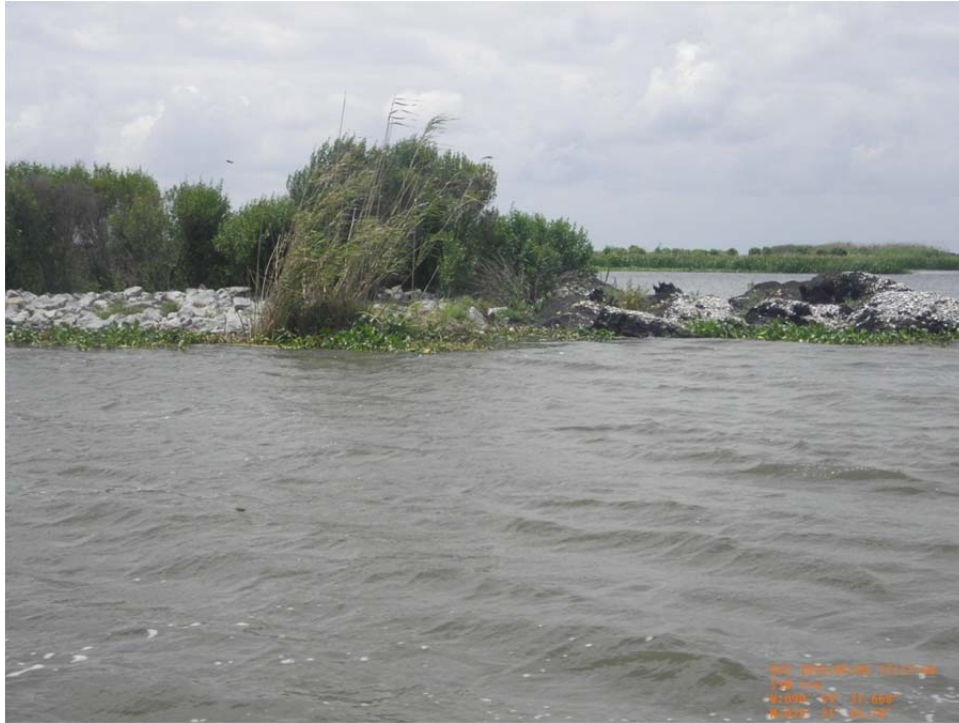
Photo 13: View of rock shoreline revetment at the entrance of Voss Canal along the west bank near Sta. 39+11 of Reach 3.
