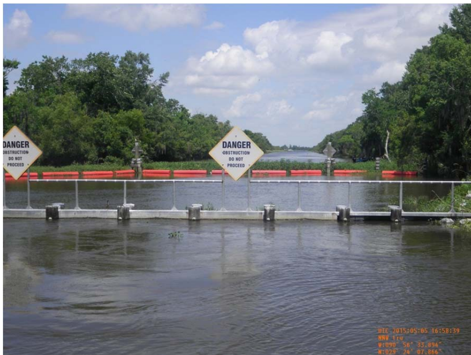
Photo 10: View of steel sheetpile weir with flapgates, floating debris barrier and warning signs across Superior Canal.
