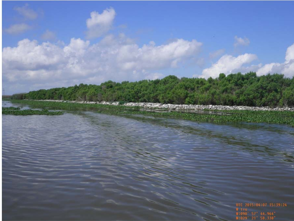
Photo 40: view of earthen embankment with rock rip rap armament along the north bank of Bayou Decade west of Structure No.6
