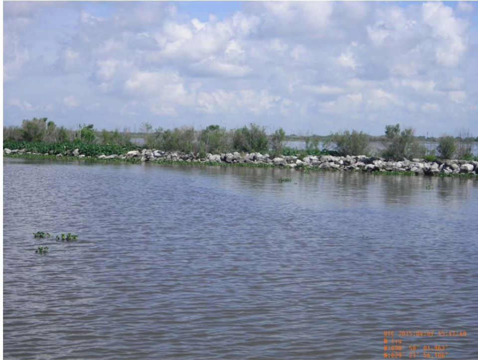
Photo 42: view of rock dike along the north bank of Bayou Decade between Structure No.6 and No.7, a rock rip rap plug.
