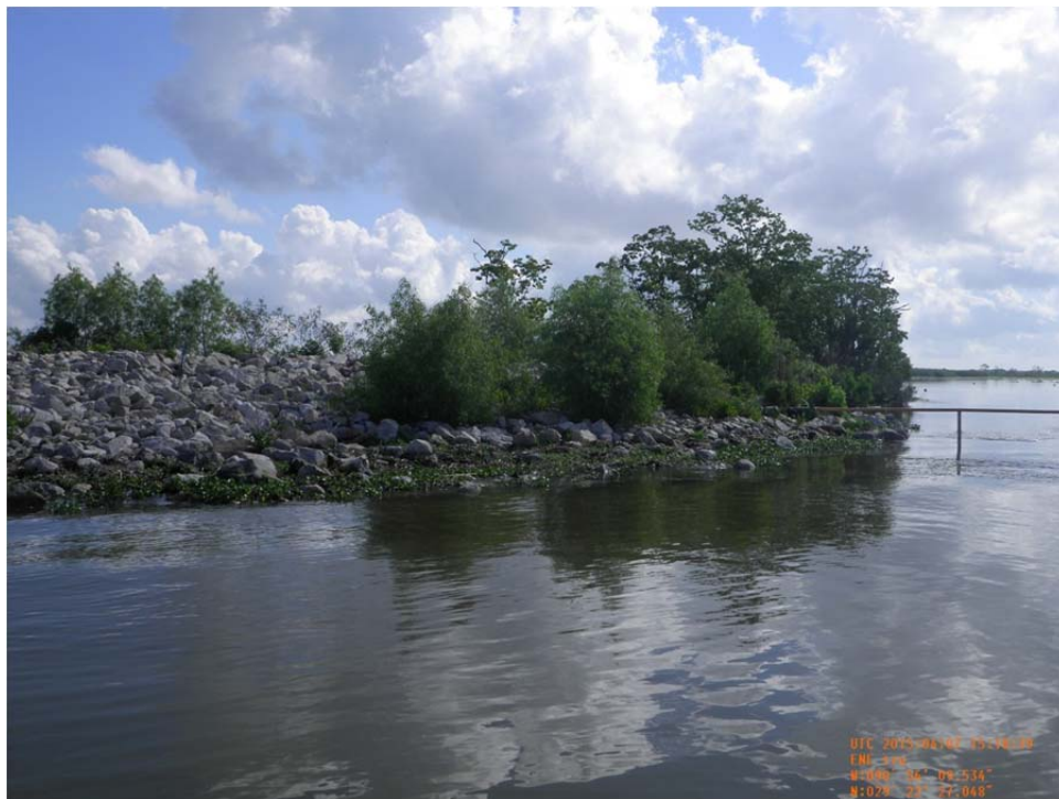
Photo 19: View of north bank tie-in of Structure No.24 located along the north bank of Jug Lake. The embankment was refurbished and rock riprap apron was installed during the 2012 Maintenance Project.
