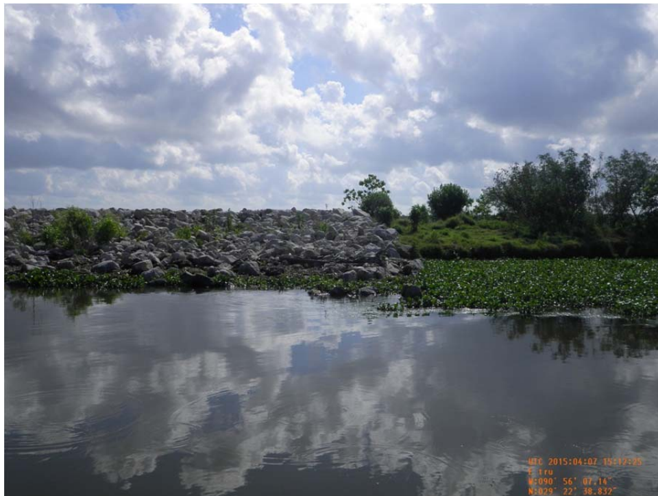
Photo 15: View of the rock armament of the earthen embankment on the south side of Structure No.23. The earthen embankment was refurbished and the rock armor installed in 2012.
