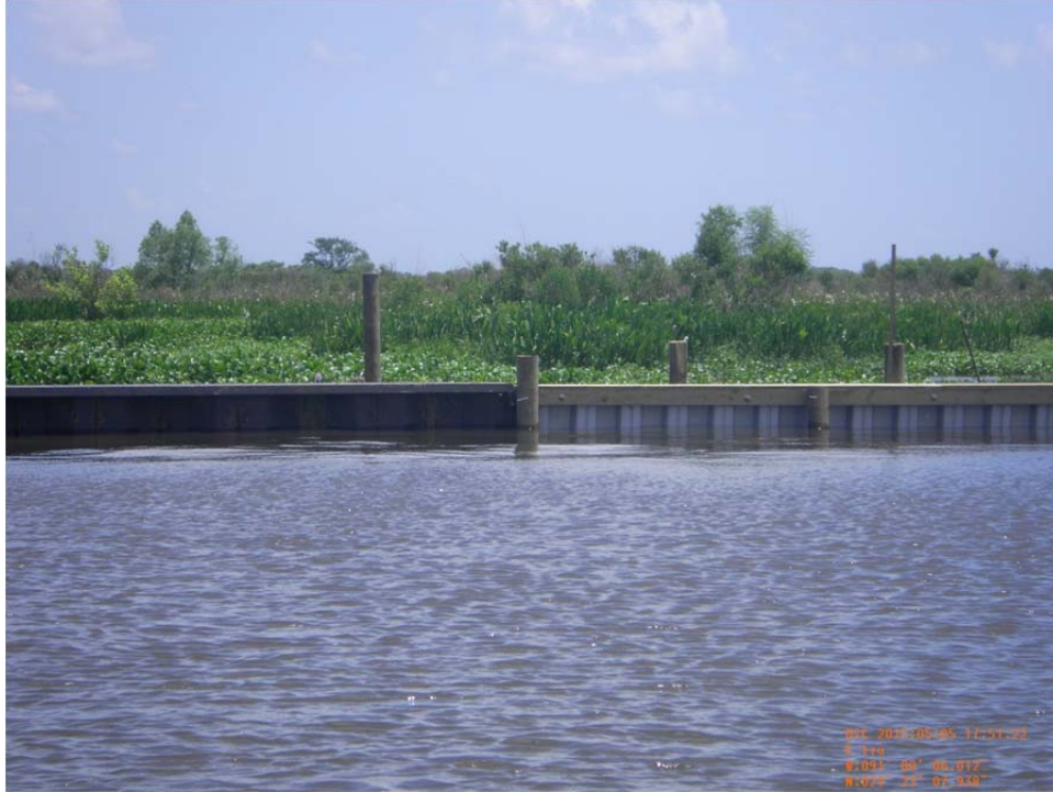
Photo 8A: view of the south section of the steel sheetpile wall and new constructed vinyl sheetpile installed by the adjacent camp owner.
