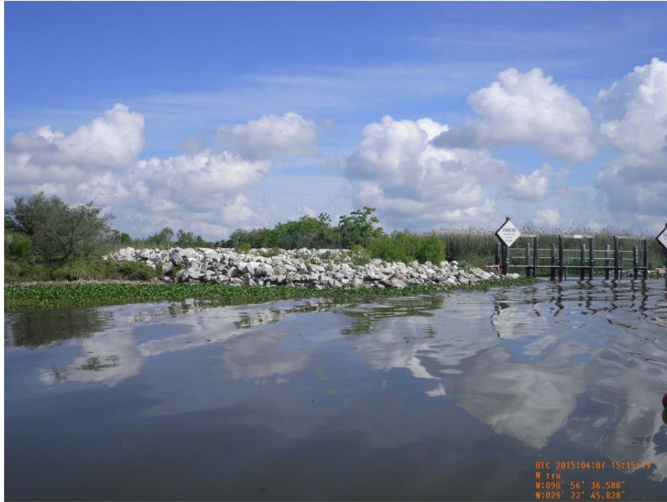
Photo 14: view of rock rip rap revetment on the south side Structure No. 21, a variable crested weir with three (3) stop log bays. The earthen embankment was refurbished and the rock rip rap revetment was installed in 2012.
