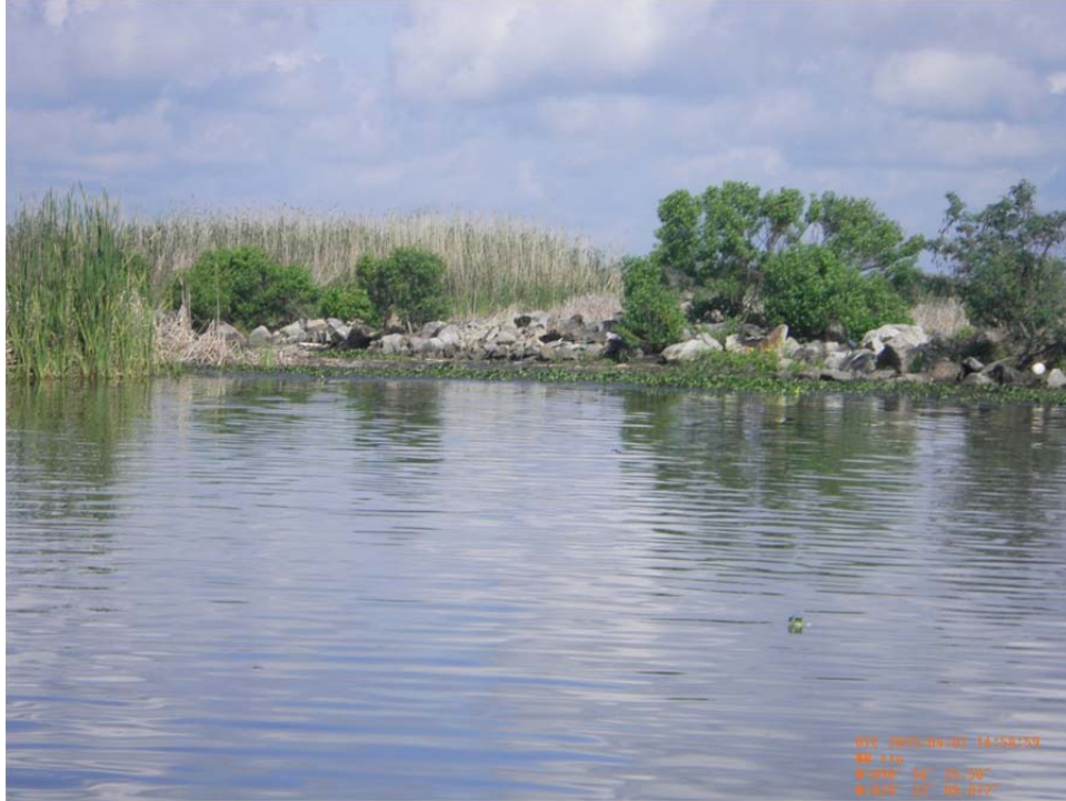
Photo 26: View of the rock armored embankment along the north bank of Bayou Decade.
