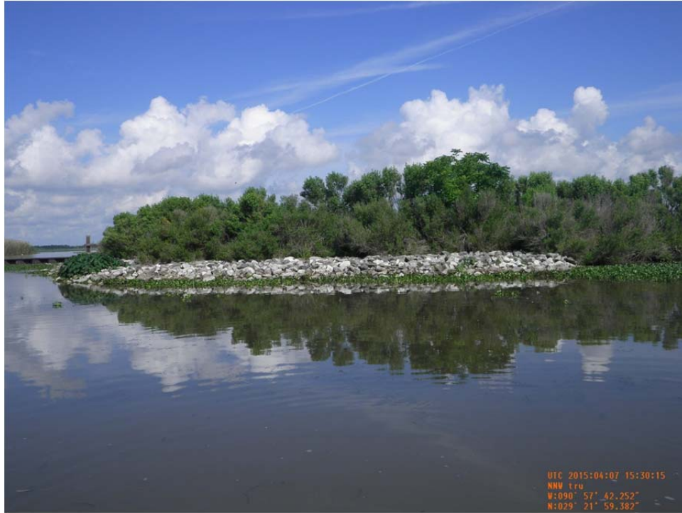
Photo 1: view of rock revetment on the east side of Structure No.6, a fixed crested weir with barge bay, along the north bank of Bayou Decade.
