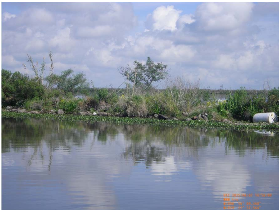
Photo 23: View of the rock armored embankment along the north bank of Bayou Decade near the mouth of Turtle Bayou. The rock armament was installed under the 2003 Maintenance Project. This structure was identified as Breaches 1 through 4.
