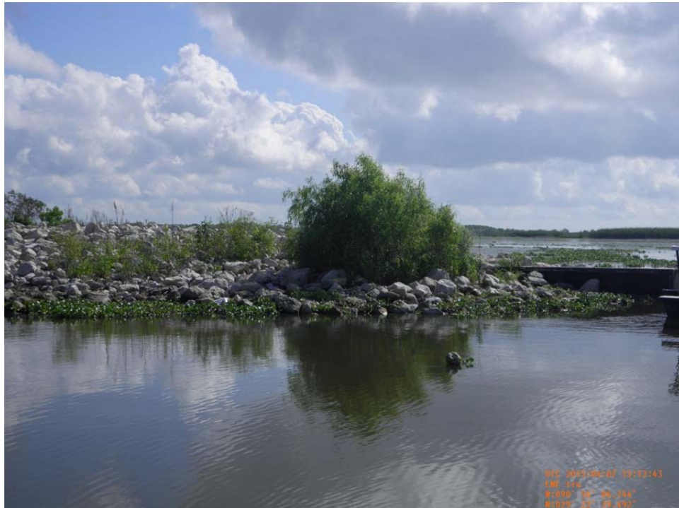
Photo 17: View of the rock armament of the earthen embankment on the north side of Structure No.23. The earthen embankment was refurbished and the rock armor installed in 2012.
