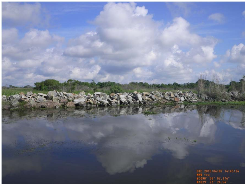
Photo 39: View of rock plug closure located along an existing location canal west of Superior Canal. This structure was constructed under the 2003 Maintenance Event, identified as Breach 7.
