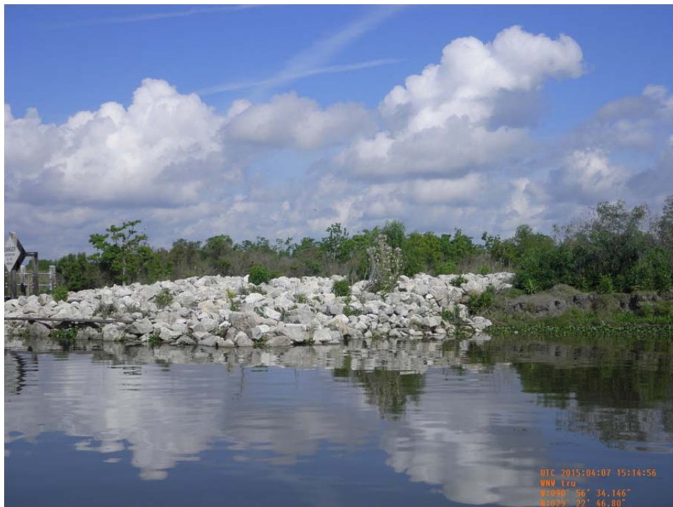
Photo 13: view of rock rip rap revetment on the north side Structure No. 21. The earthen embankment was refurbished and the rock rip rap revetment was installed in 2012.
