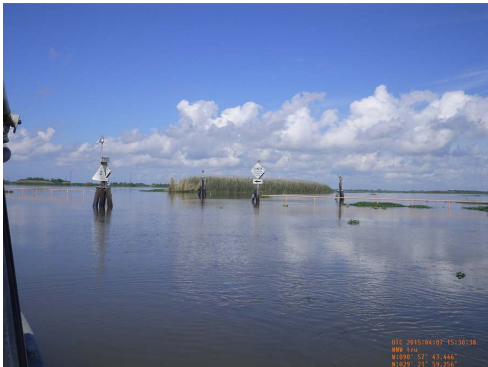
Photo 2: view of Structure No.6, a fixed crested weir with barge bay and navigational aids and signage on both sides of the structure.
