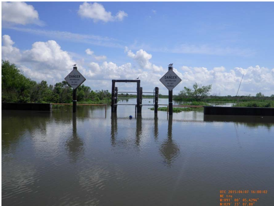
Photo 9: an overall view of the variable crested weir with stop log bay (Structure No.14)
