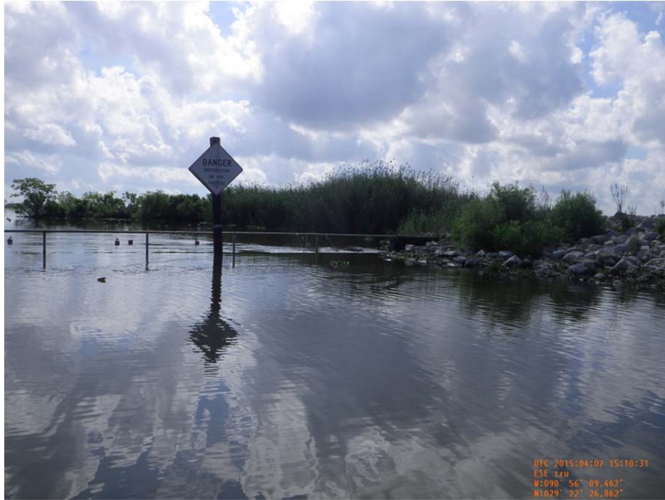
Photo 18: View of south bank tie-in of Structure No.24 located along the north bank of Jug Lake. The embankment was refurbished and the rock riprap apron was installed during the 2012 Maintenance Project.
