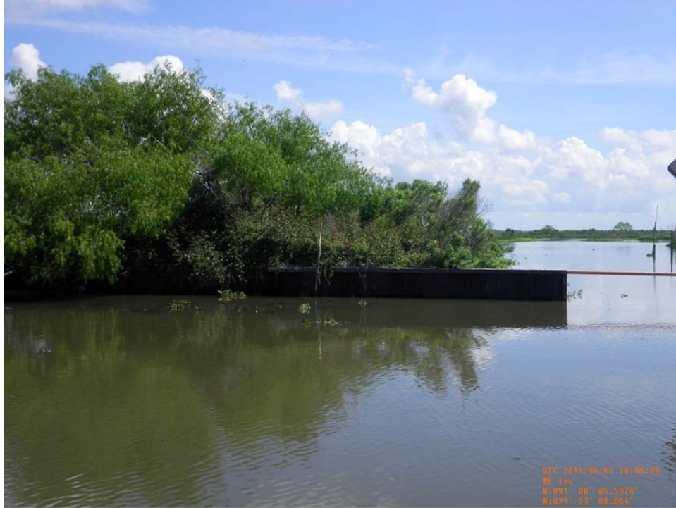
Photo 10: view of the north section of the steel sheetpile wall and bank tie-in at Structure No.14. The structure is a variable crest weir with a single stop log bay.
