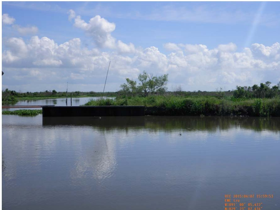
Photo 8: view of the south section of the steel sheetpile wall and bank tie-in at Structure No.14. The structure is a variable crest weir with a single stop log bay.
