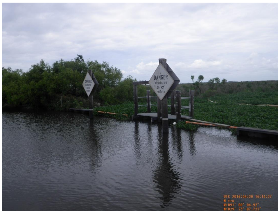
Photo 9: view of the north section of the steel sheetpile wall and bank tie-in at Structure No.14. The structure is a variable crest weir with a single stop log bay.
