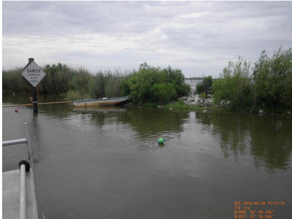
Photo 15: View of south bank tie-in of Structure No.24 located along the north bank of Jug Lake. The embankment was refurbished and the rock riprap apron was installed during the 2012 Maintenance Project.
