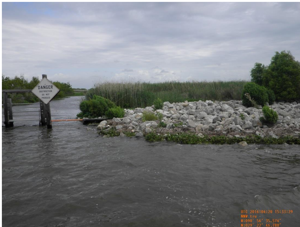
Photo 12: view of rock rip rap revetment on the north side Structure No. 21.
