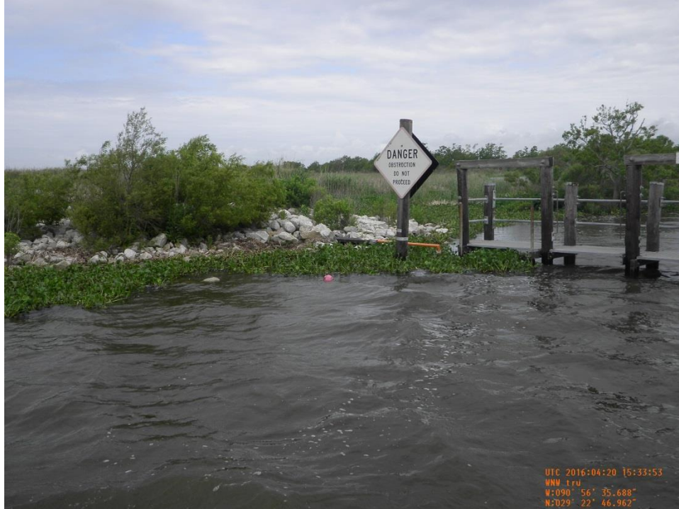
Photo 13: view of rock rip rap revetment on the south side Structure No. 21.
