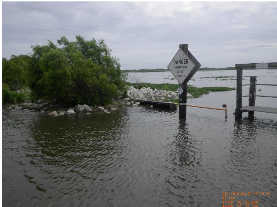
Photo 14: View of the rock armament of the earthen embankment on the north side of Structure No.23. The earthen embankment was refurbished and the rock armor installed in 2012.
