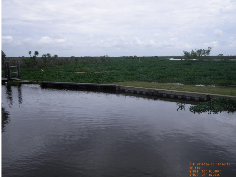
Photo 7: view of the south section of the steel sheetpile wall and new constructed vinyl sheetpile installed by the adjacent camp owner.
