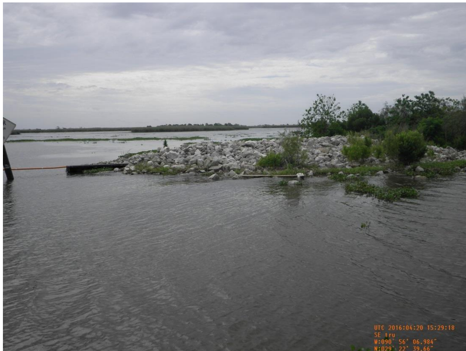
Photo 12: View of the rock armament of the earthen embankment on the south side of Structure No.23. The earthen embankment was refurbished and the rock armor installed in 2012.
