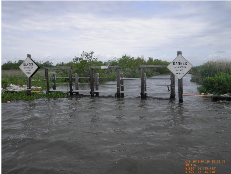
Photo 11: view of rock rip rap revetment on the north side Structure No. 21, a variable crested weir with three (3) stop log bays. The earthen embankment was refurbished and the rock rip rap revetment was installed in 2012.
