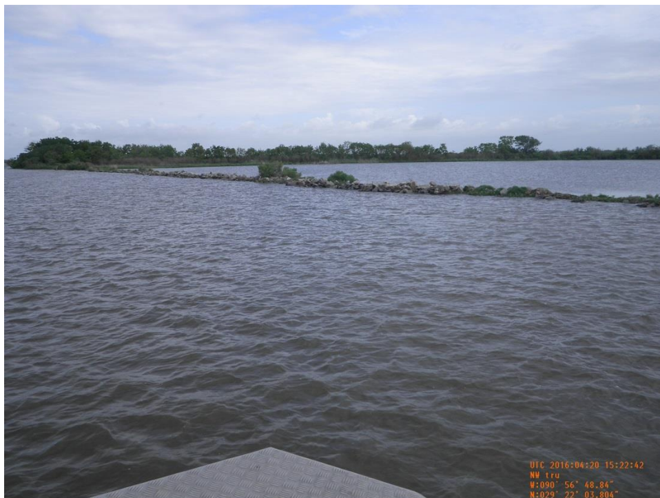
Photo 24: View of the rock armored embankment along the north bank of Bayou Decade near Jug Lake.
