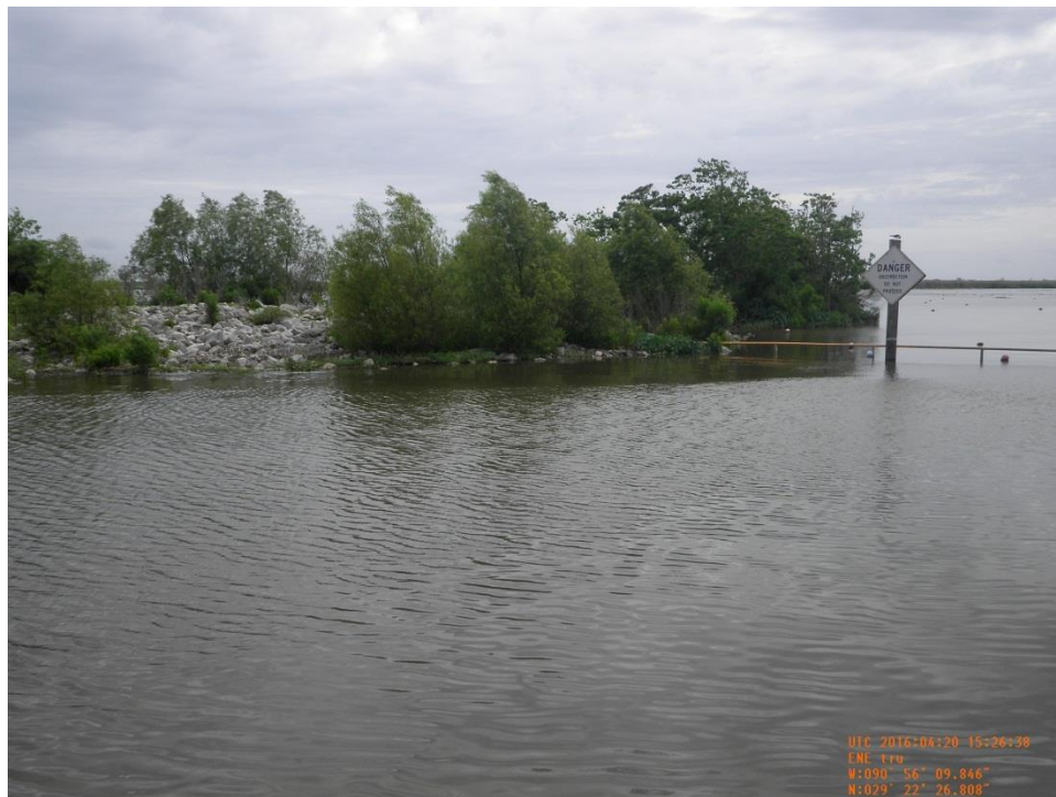
Photo 16: View of north bank tie-in of Structure No.24 located along the north bank of Jug Lake. The embankment was refurbished and rock riprap apron was installed during the 2012 Maintenance Project.
