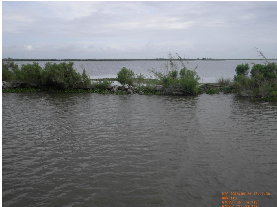
Photo 20: View of the rock armored embankment along the north bank of Bayou Decade near the mouth of Turtle Bayou. The rock armament was installed under the 2003 Maintenance Project. This structure was identified as Breaches 1 through 4.
