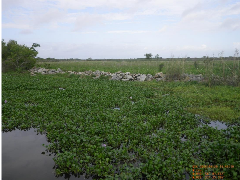
Photo 31: View of rock plug closure located along an existing location canal west of Superior Canal. This Structure was constructed under the 2003 Maintenance Event, identified as Breach 7
