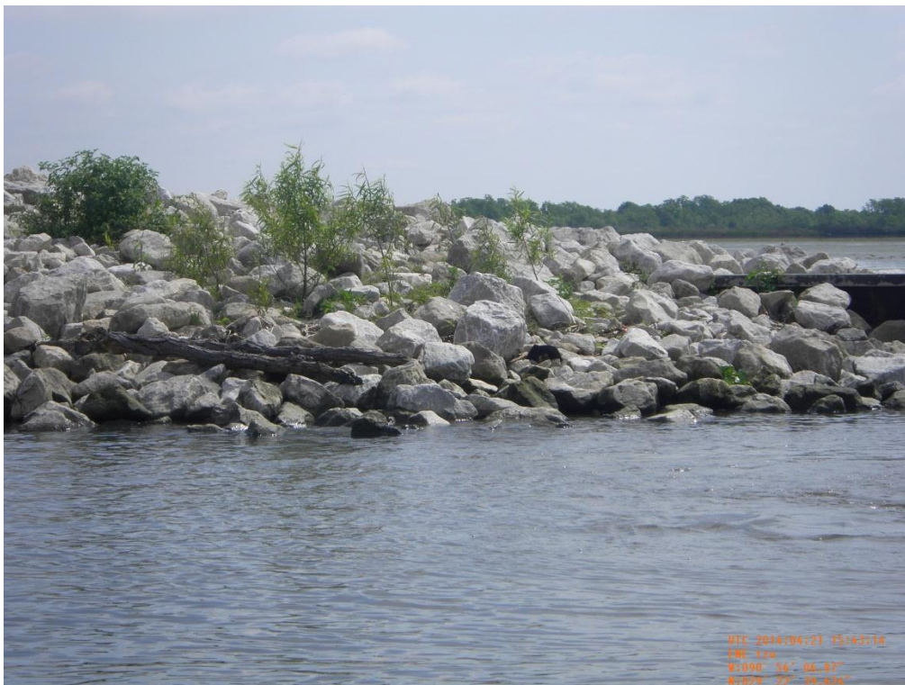
Photo 13: View of the rock armored embankment tie-in located on the northern side of Structure 23
