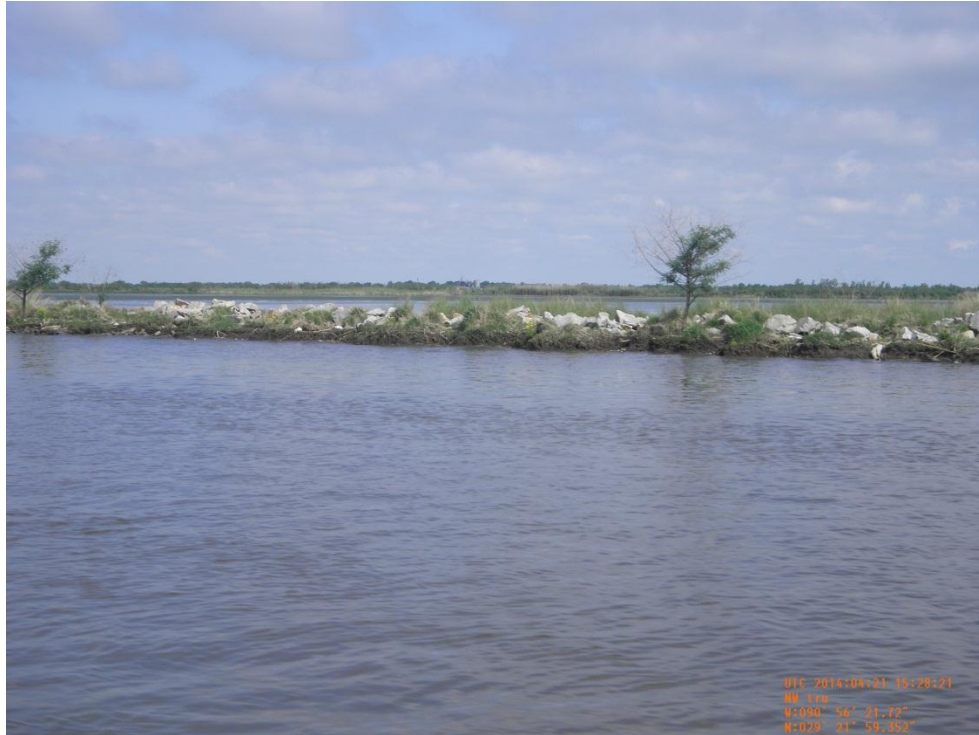
Photo 5: View of the rock armored embankment along the north side of Bayou DeCade between Turtle Bayou and Jug Lake taken from Bayou DeCade
