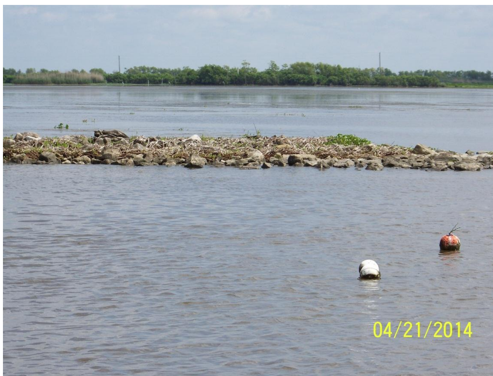
Photo 28: View of northern end of Structure 10 fixed crest rock weir with barge bay
