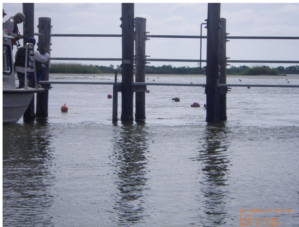
Photo 12: View of Structure 23 variable crest weir timbers, warning signs and steel piping
