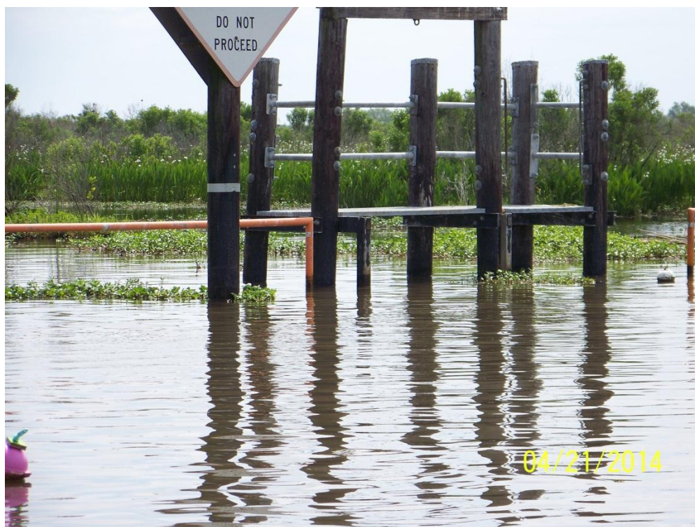
Photo 32: Overall view of Structure 14 variable crest weir timbers, warning signs, and steel piping
