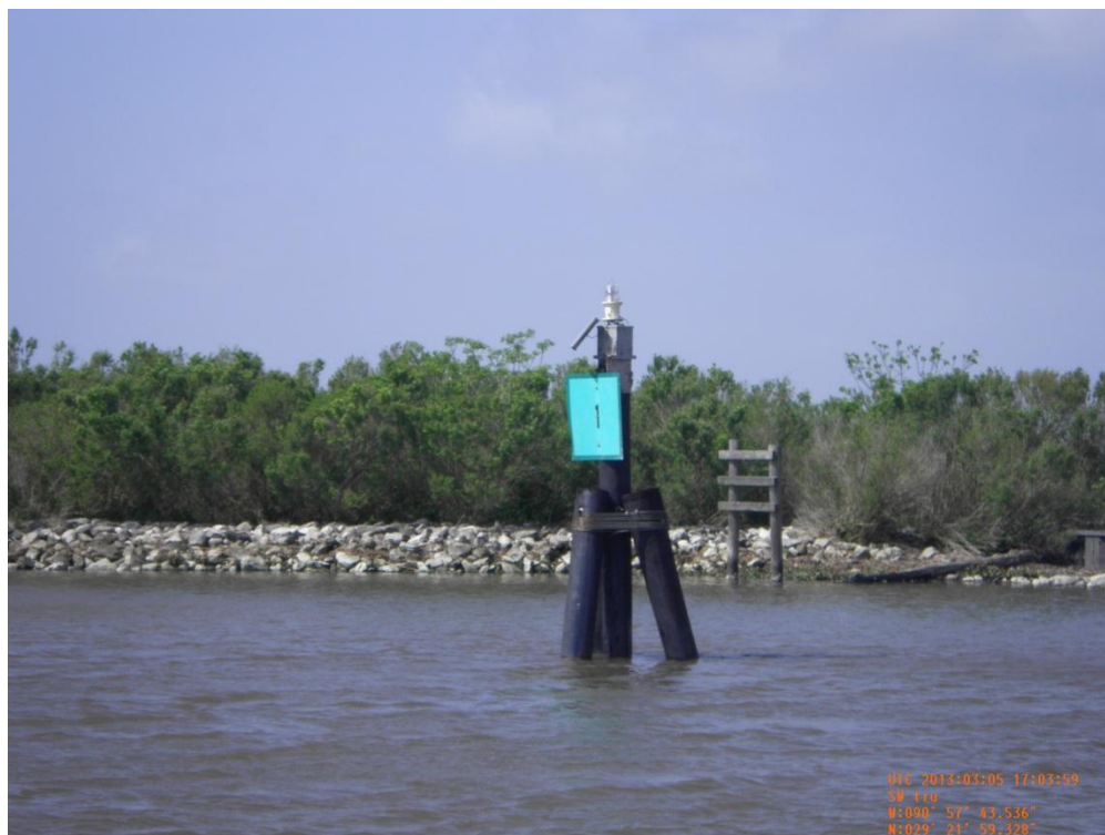
Photo 25: View of Structure 6 replaced timber pile dolphin included in 2012 Maintenance Project
