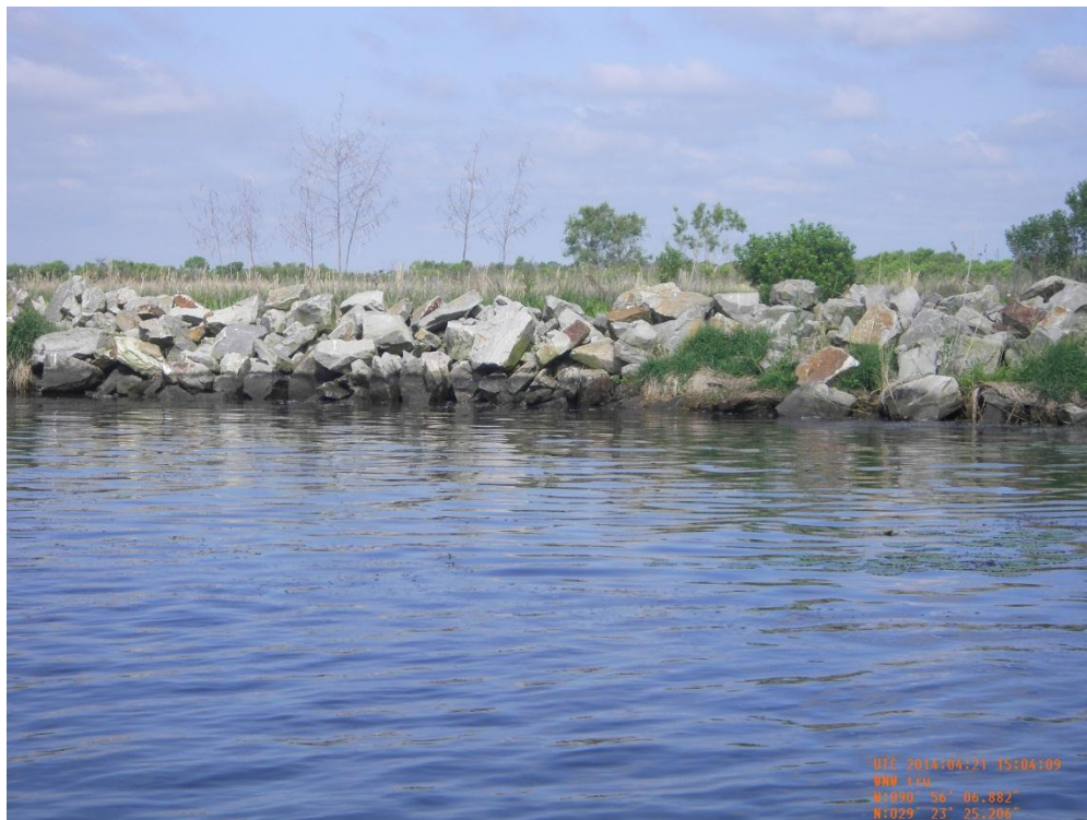
Photo 1: Breach 7 located in an oilfield access canal off of Superior Canal. There is no visible settlement or displacement of the rock fill material.
