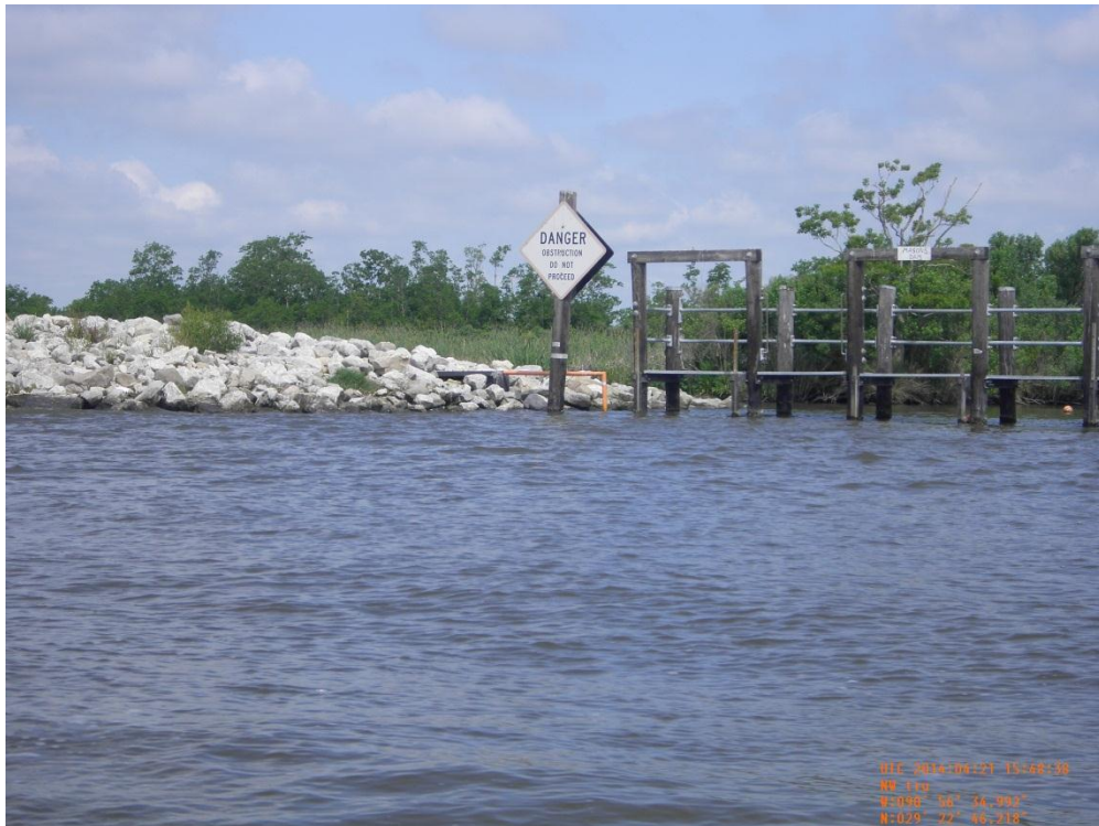
Photo 18: View of the rock armored embankment tie-in on the west side of Structure 21
