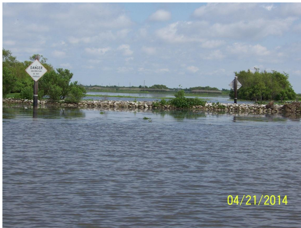
Photo 27: View of Structure 7 rock plug along the north bank of Bayou Decade
