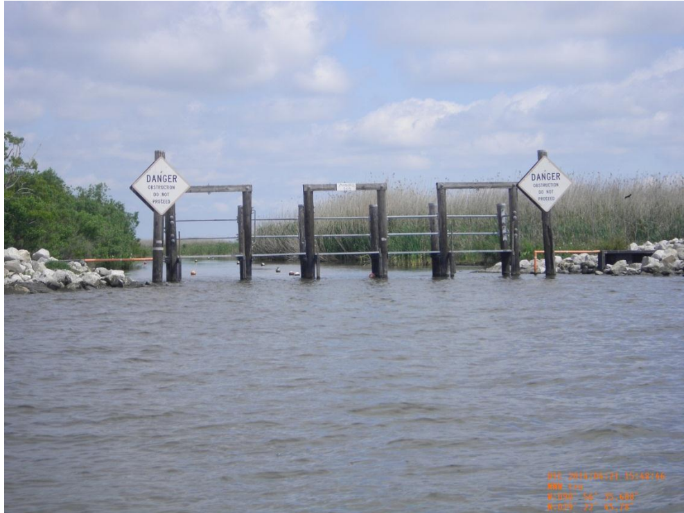
Photo 17: View of Structure 21 variable crest weir timbers, warning signs and steel piping
