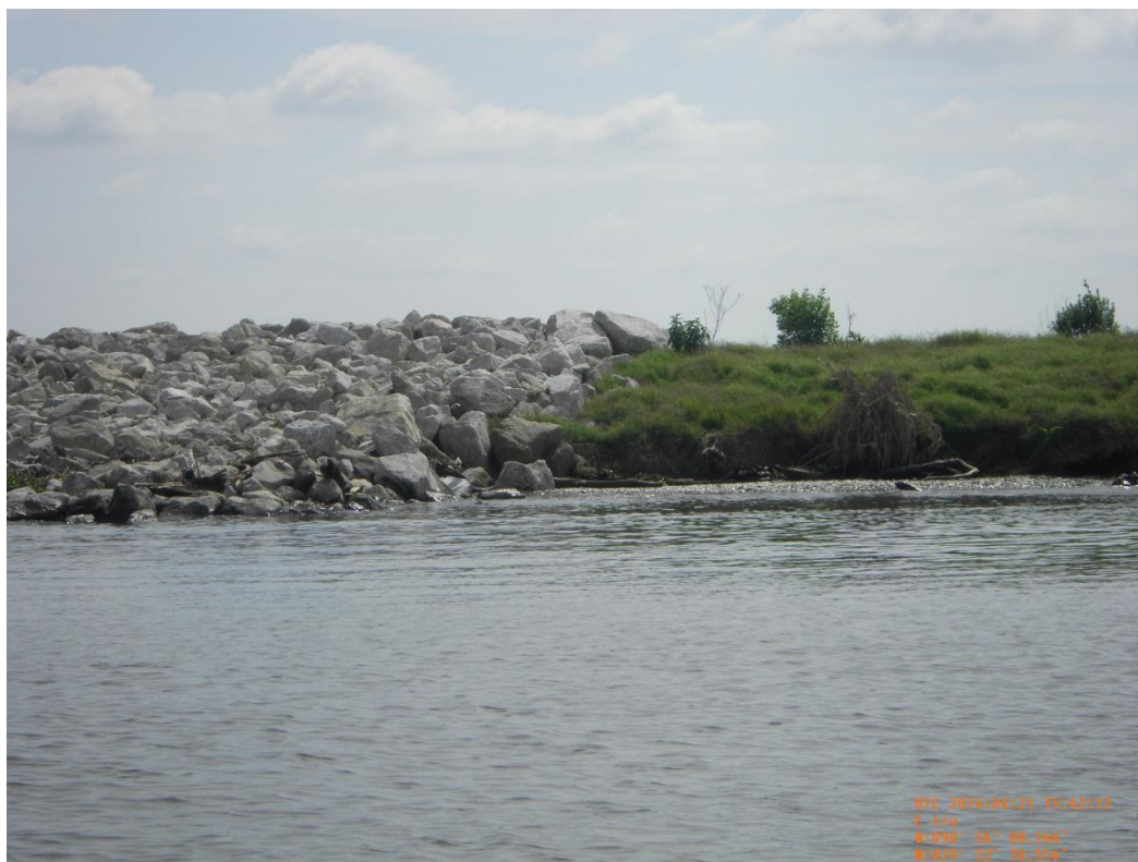
Photo 11: View of the rock armored embankment on the southern end of Structure 23
