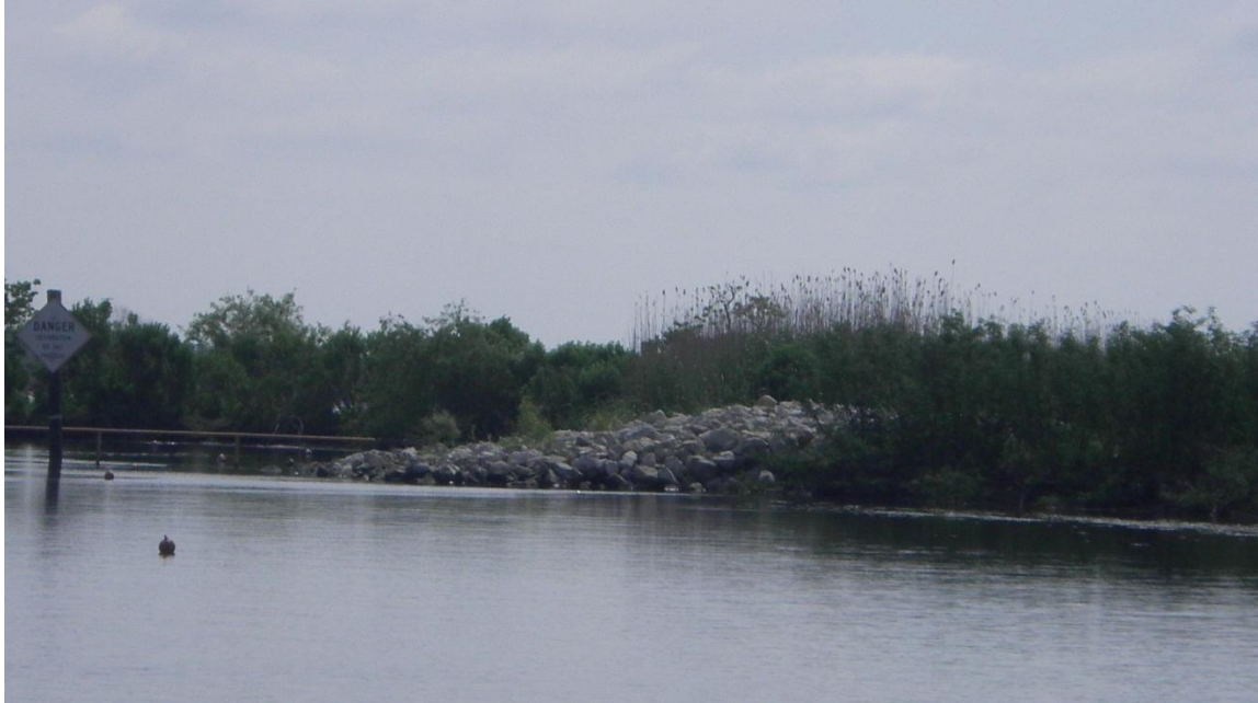
Photo 9: View of the rock armored embankment tie-in located on the southern end of Structure 24
