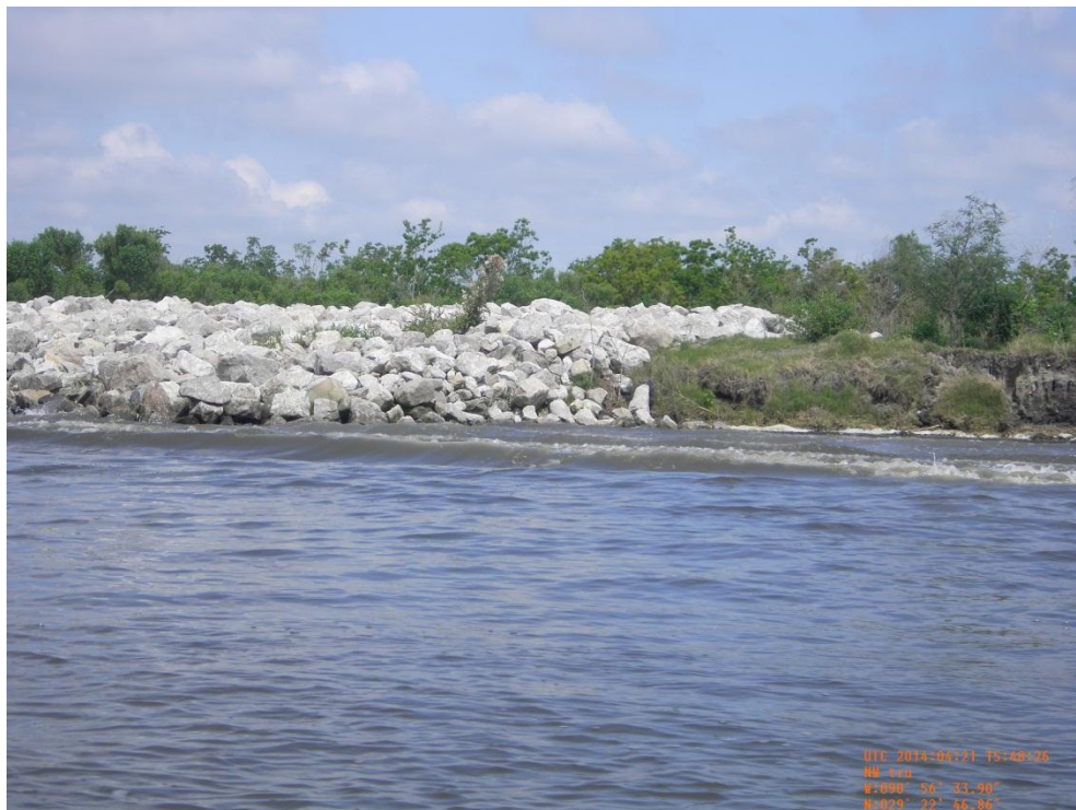
Photo 16: View of the rock armored embankment tie-in on the east side of Structure 21
