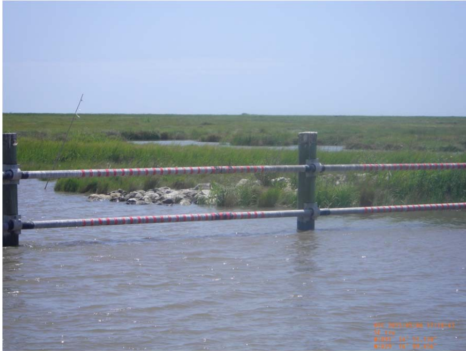
Photo 13: View of rock plug tie-in to bank line and timber barricade system on the southwest side of Structure No.6.
