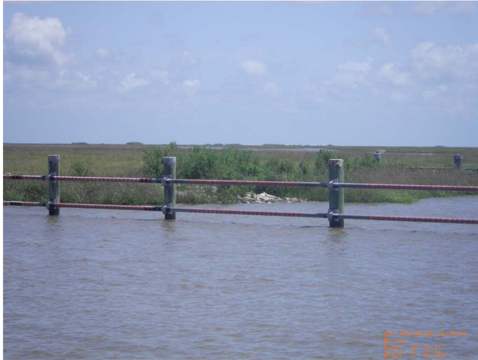
Photo 5: Rock plug tie-in to marsh on the north bank and timber barricade system at Structure No.9.
