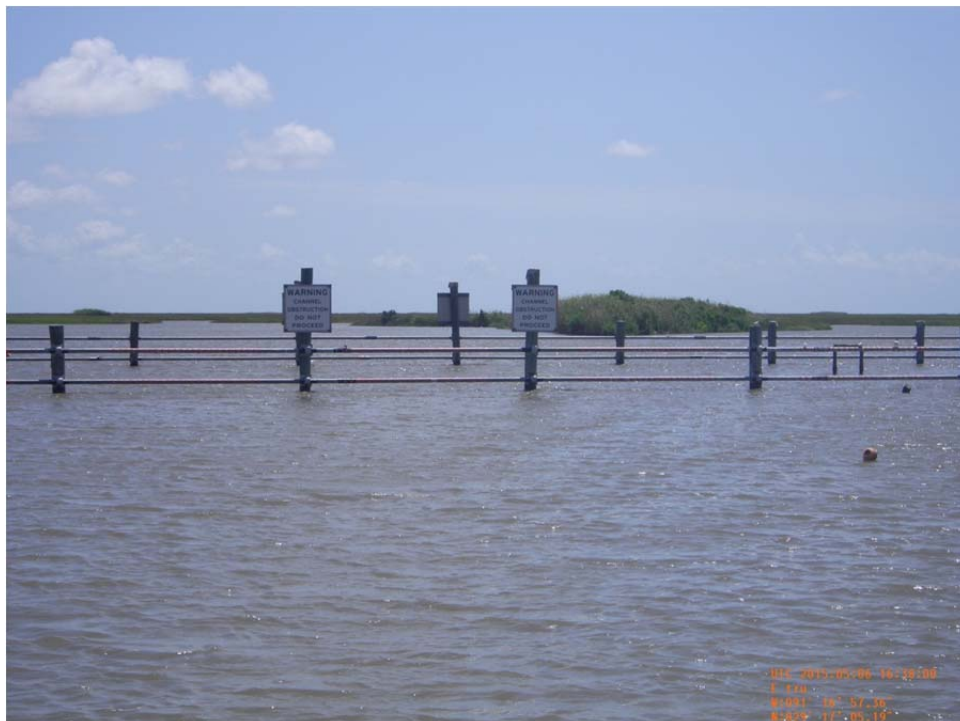
Photo 4: View of rock plug, timber barricade and signage of Structure No.9.
