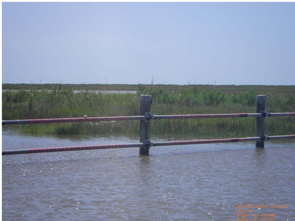
Photo 6: Rock plug tie-in to marsh on the south bank and timber barricade system at Structure No.9
