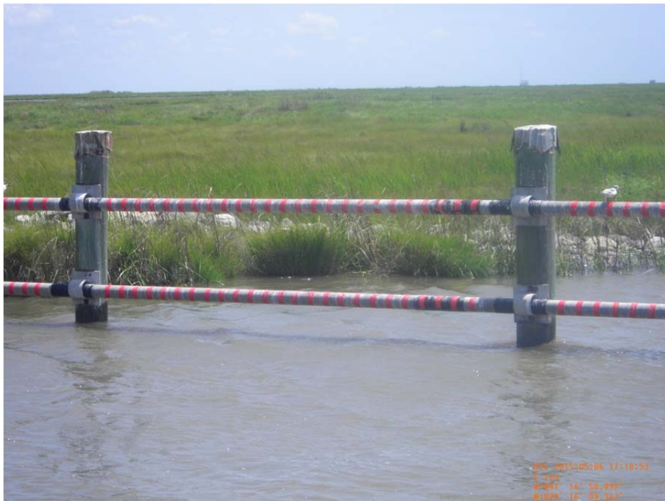
Photo 14: View of rock weir tie-in to bank line and timber barricade system on the northeast side of Structure No.6.
