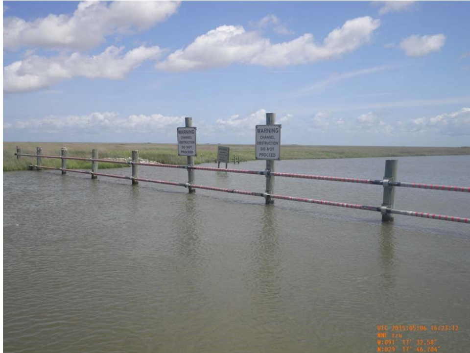
Photo 3: Overall view of rock plug, timber barricade structure and warning signs on Structure No.1.
