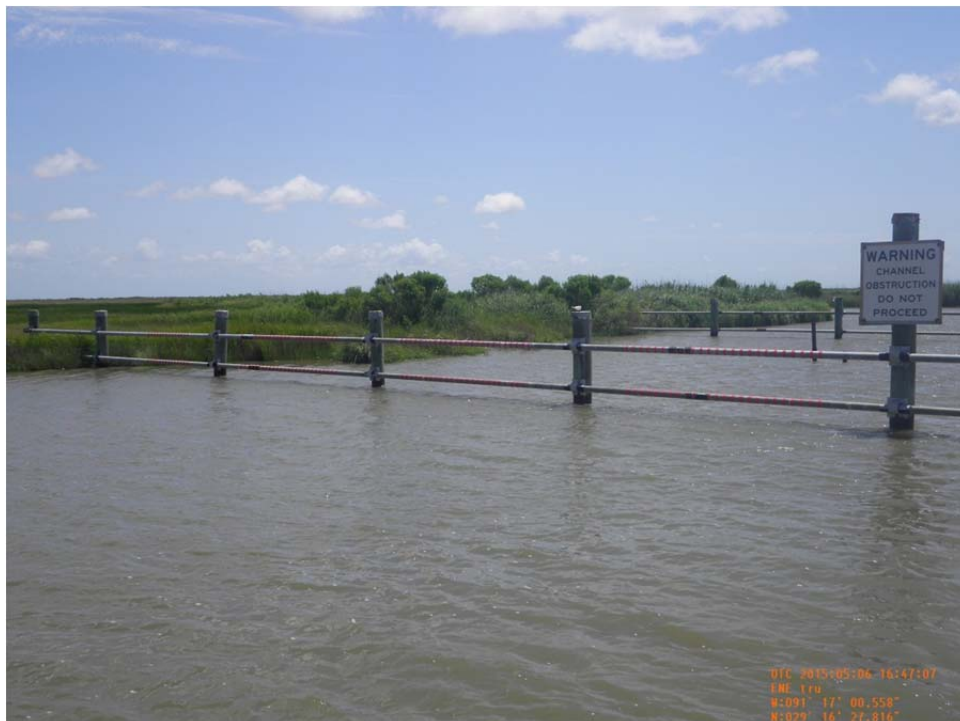
Photo 10: View of rock weir, timber barricade system and warnings sign on the northeast bank of Structure No.7.
