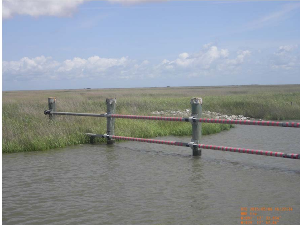
Photo 1: View of rock weir, timber barricades, and signs, and northwest bank tie-in on Structure No.1
