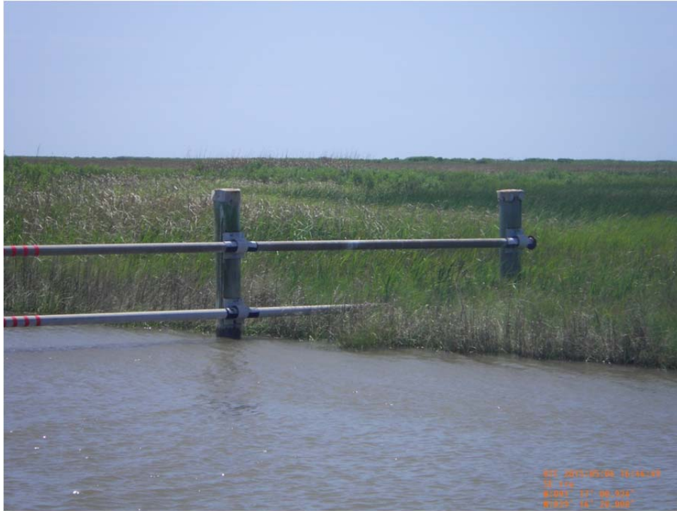
Photo 7: View of timber barricade system along southwest bank of Structure No.7.
