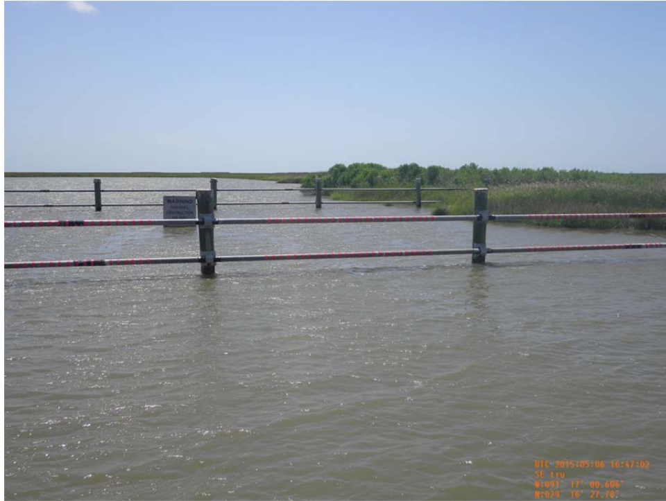
Photo 9: View of rock weir and timber barricade system along southwest bank of Structure No.7.
