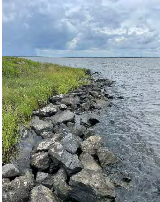
Northern Section – Station 113+70 (Looking Northerly) Lat: 29°25'38"N Long: 90°40'36"W
