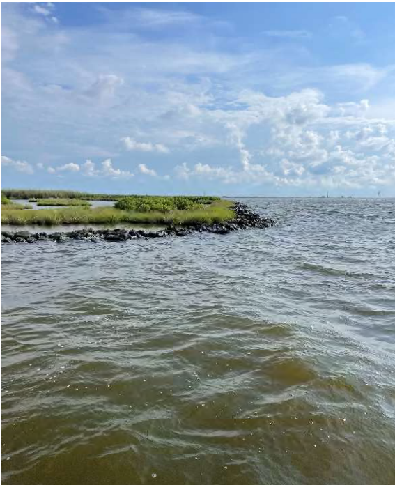
Northern Section – Station 116+60 (Looking Northerly) Lat: 29°25'34"N Long: 90°40'38"W
