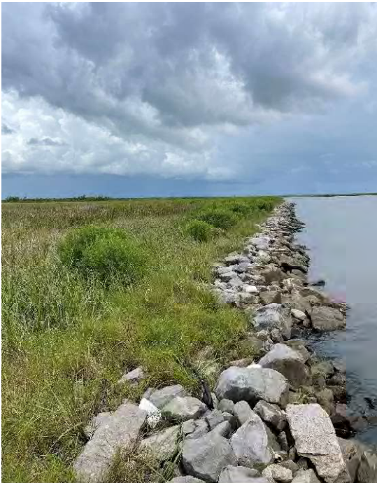
Northern Section – Station 107+20 (Looking Northerly) Lat: 29°25'44"N Long: 90°40'38"W
