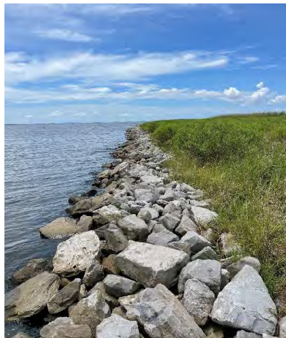
Northern Section – Station 107+20 (Looking Southerly) Lat: 29°25'44"N Long: 90°40'38"W
