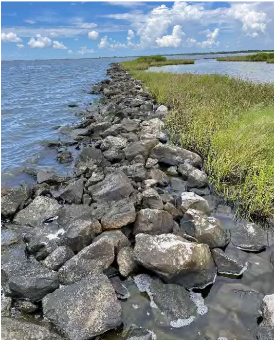
Northern Section – Station 112+45 (Looking Southerly) Lat: 29°25'39"N Long: 90°40'35"W
