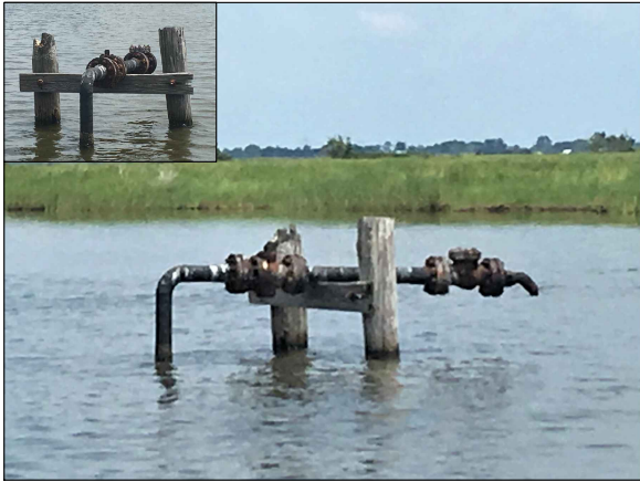
24 PIPELINE TAP ON PILES 1225
