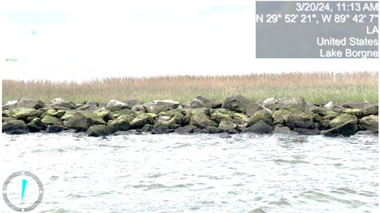
Photo 16: Reach 3 Rock breakwater in generally good condition
