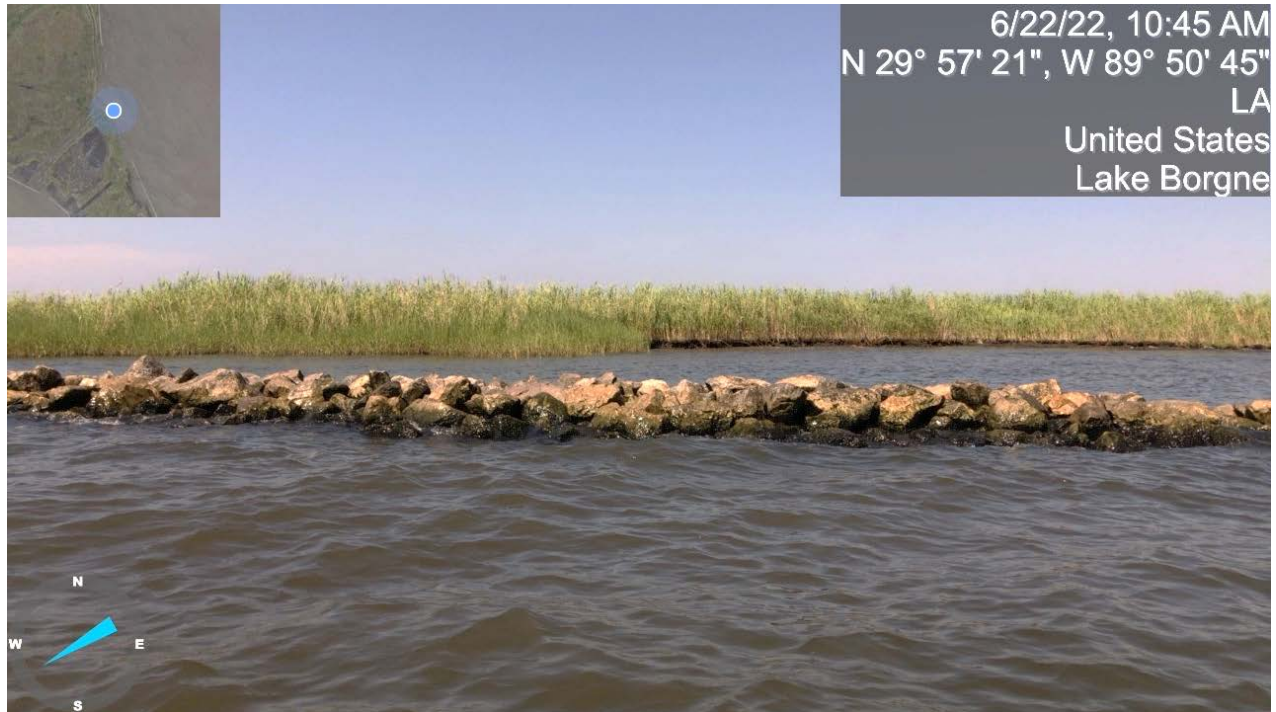
Photo 9: Reach 1 Rock breakwater in generally good condition
