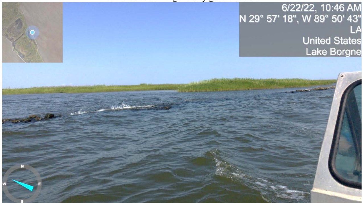
Photo 10: Reach 1 This area of the rock breakwater has experienced significant settlement.
