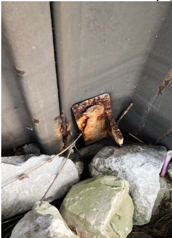
Photos 4 & 5: Fabricated metal piece was loosely attached to the sheetpile and fell off when touched. This photo is from downstream northeast bank. An identical piece was found at roughly the same location on the upstream northeast bank.
