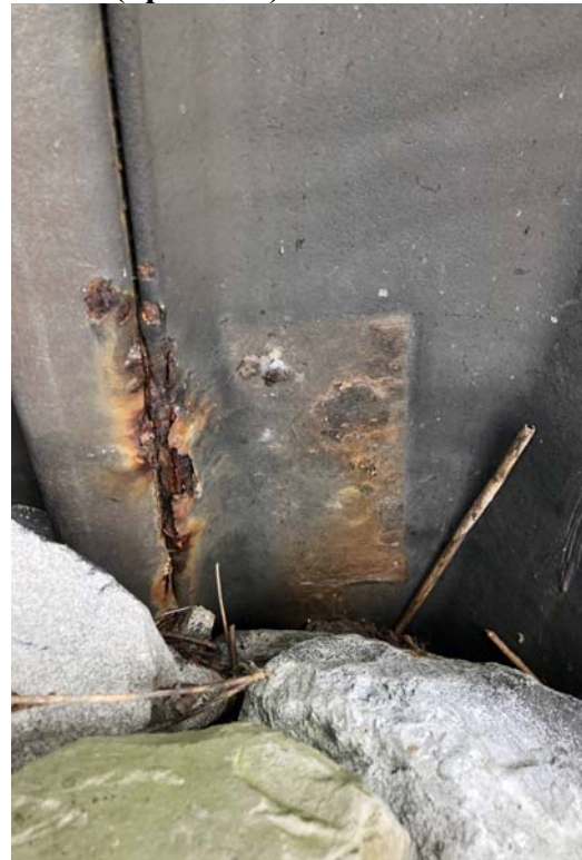
Photos 4 & 5: Fabricated metal piece was loosely attached to the sheetpile and fell off when touched. This photo is from downstream northeast bank. An identical piece was found at roughly the same location on the upstream northeast bank.
