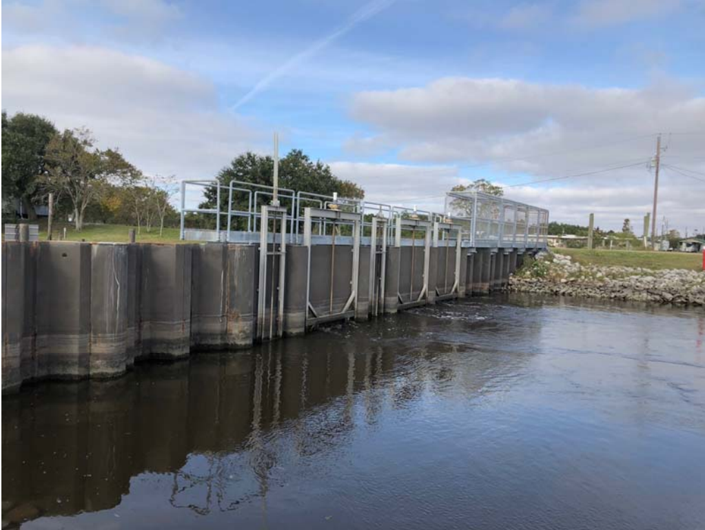
Photo 1: Structure viewed from project exterior (downstream) on southern bank
