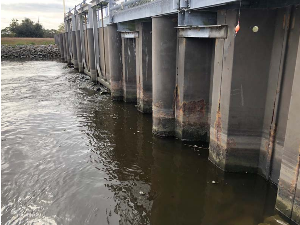
Photo 2: Structure viewed from project exterior (downstream) on northern bank
