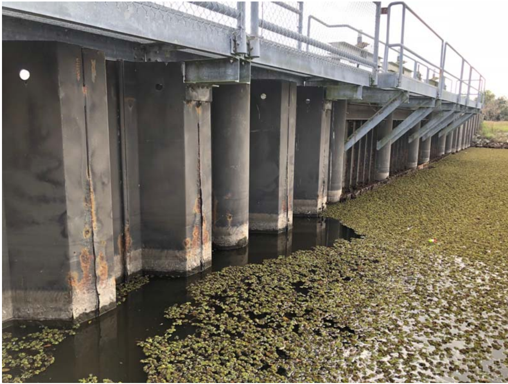
Photo 3: Structure viewed from project interior (upstream) northern bank
