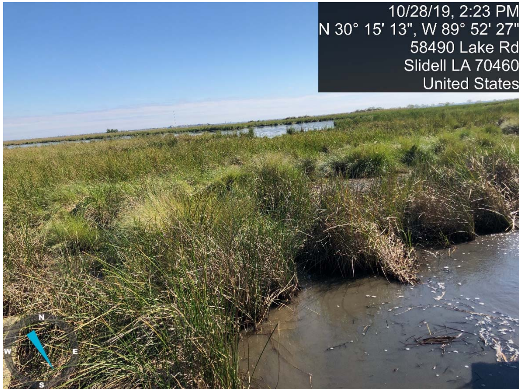
Photo 17: Marsh Creation Area 4 Earthen containment dike at the NE corner of MCA 4
