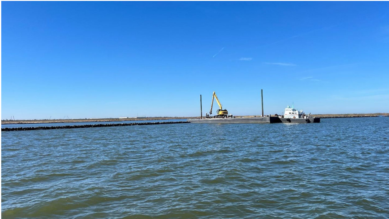
Photo #3 – Northern Reach (Nav Aid Installation).
