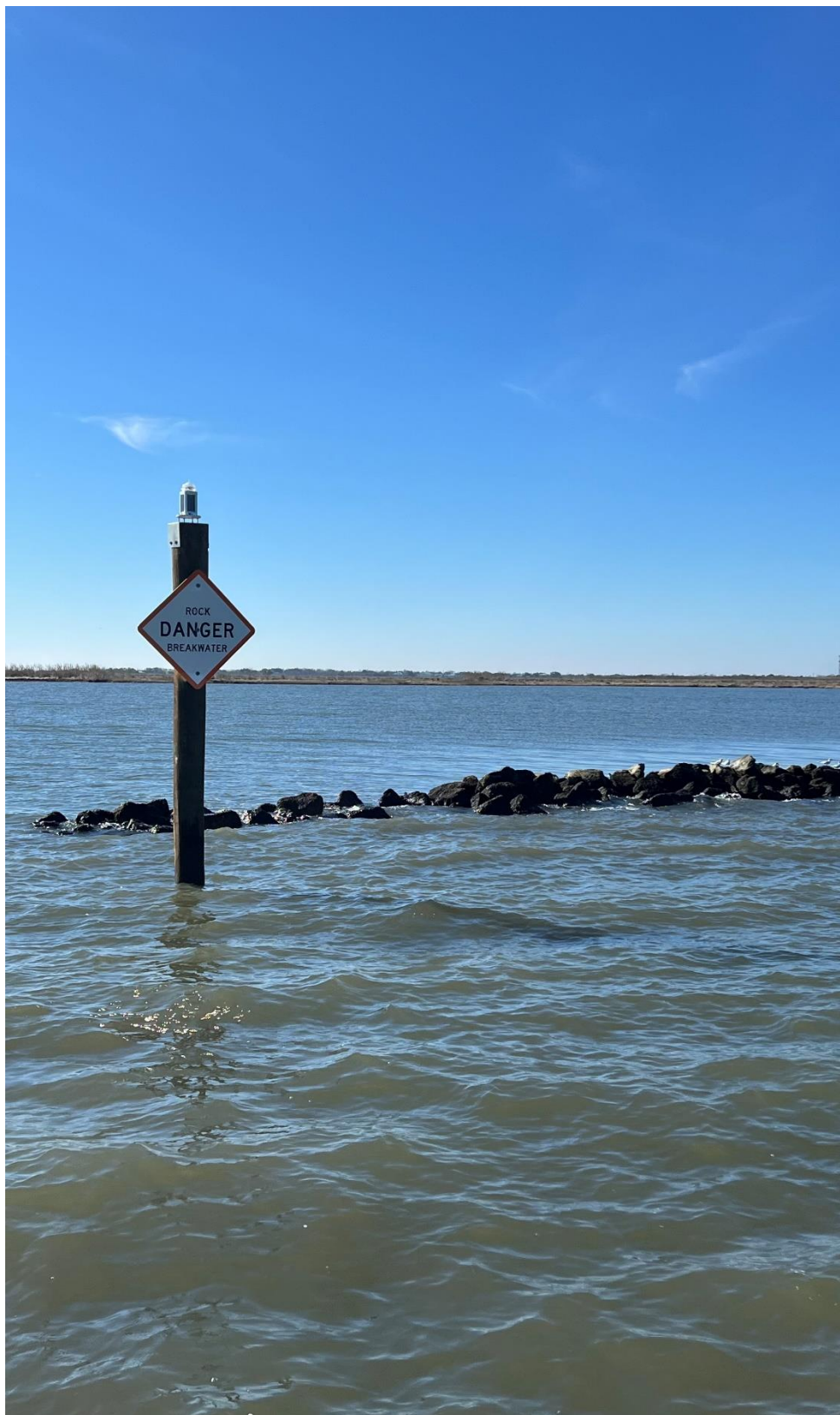
Photo #2 – Installed Nav Aid.
