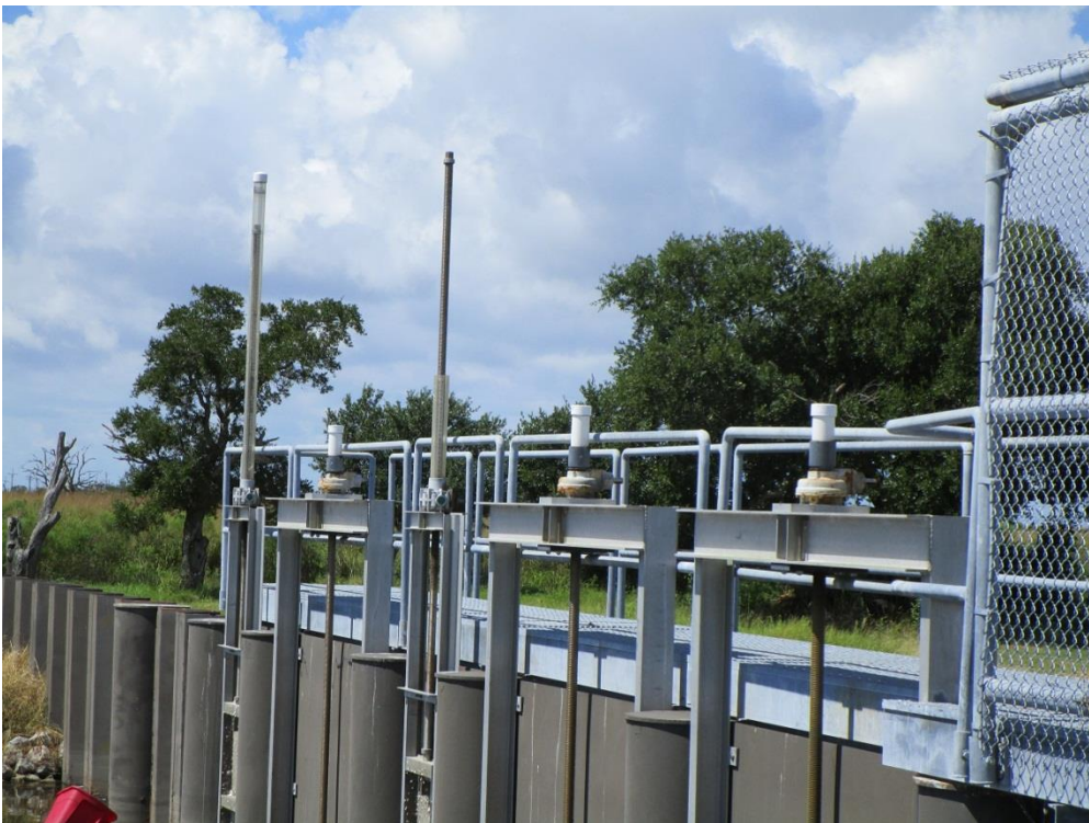
Photo 2. Damaged Stem Cover
