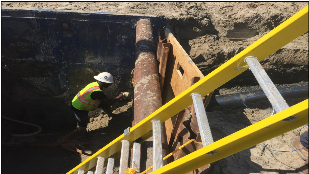
Figure 2: Waterline Relocation – View of the Trench Box and HDPE Pipe During the Waterline Relocation
