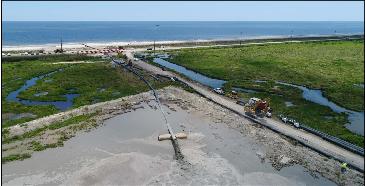
Figure 9: Aerial of WMI Placing Marsh Fill Within MCA 3
