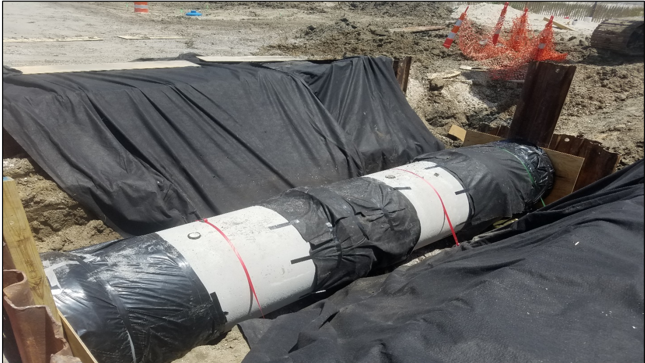
Figure 3: Concrete Casing Pipe Installation (Eastbound Lane on 5/16/2017)
