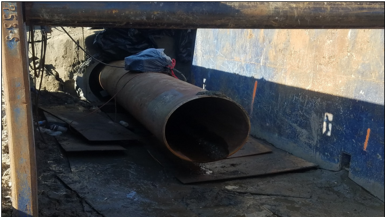
Figure 4: View of the temporary sediment pipeline installation within the concrete casing pipe
