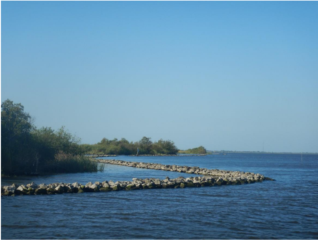
Photo 5: Zoomed-In View of ME-22 Rock Rip Rap Shoreline Protection Feature, Facing West
