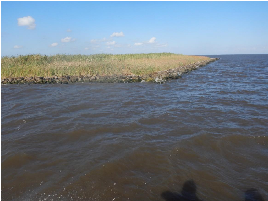
Photo 18: View of ME-22 Rock Rip Rap Shoreline Protection Feature, Pictured Near Entrance Into Bear Lake, Facing West
