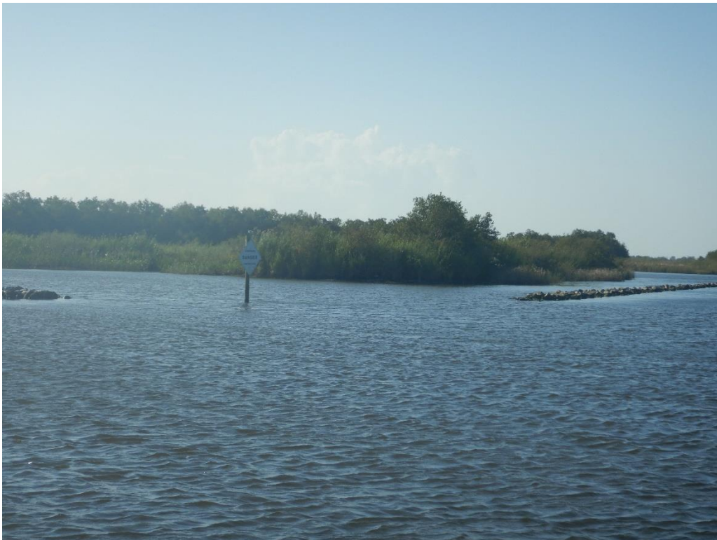
Photo 4: Photograph of ME-22 Rock Rip Rap Shoreline Protection Feature, Pictured Near Eastern End of Project Footprint, Warning Sign and Fisheries Access Gap Shown, Facing Southwest
