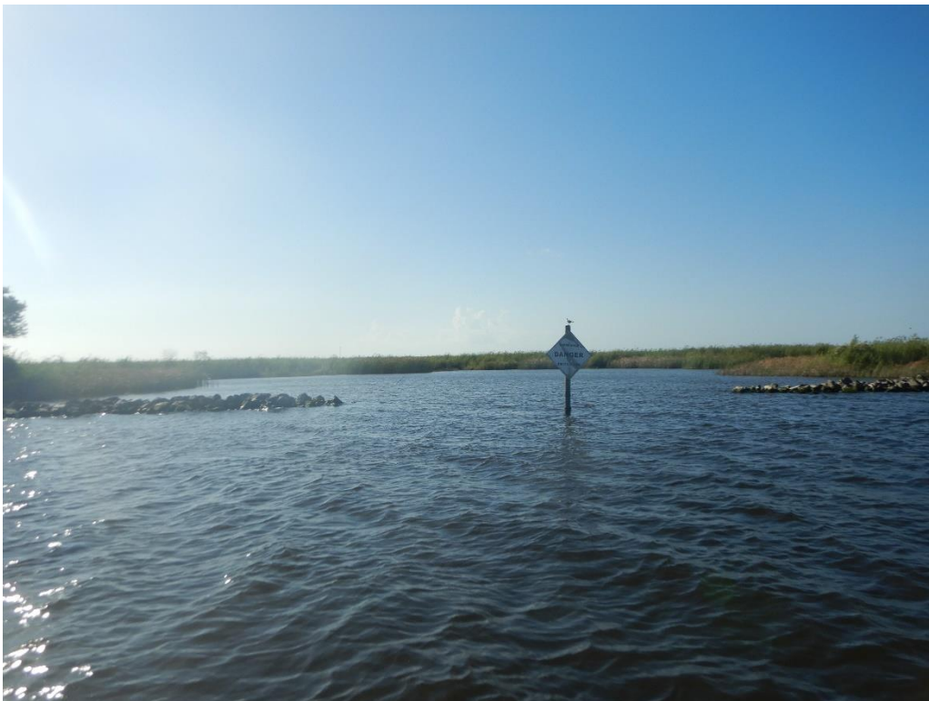
Photo 8: Photograph of ME-22 Rock Rip Rap Shoreline Protection Feature, Pictured Near Central Portion of Project Footprint, Warning Sign and Fisheries Access Gap Shown, Warning Sign Maintenance Needed, Facing South
