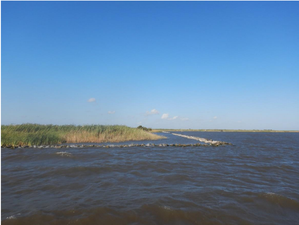
Photo 14: Photograph of ME-22 Rock Rip Rap Shoreline Protection Feature, Pictured Near Western End of Project Footprint, Facing West
