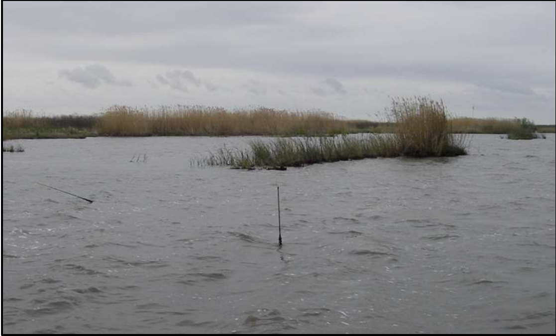
Figure 13. Many terraces have eroded since construction, especially the lakeside terraces (e.g. LS42) which were intended to be sacrificial and buffer the marsh side terraces. Note the cane poles that mark the original corners of the terrace. Picture was taken on March 24, 2010.
