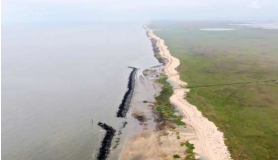
Figure 10. Photograph provided by Philip Trosclair, Rockefeller Refuge Manager taken on 11/16/2023 facing west at the western end of ME-37, which is a continuation from the western extent of ME-0018. This photograph demonstrates the sediment stabilization behind the structure.
