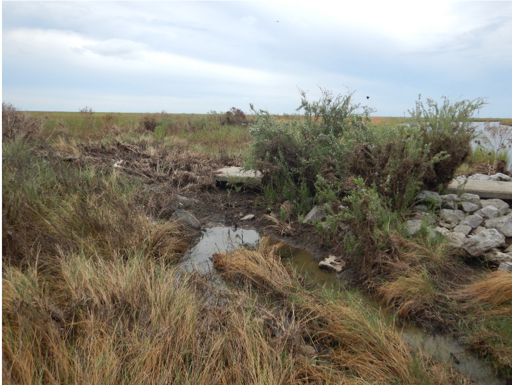
Photo No. 5, Little Constance Structure – Erosion and scour around end of structure.
