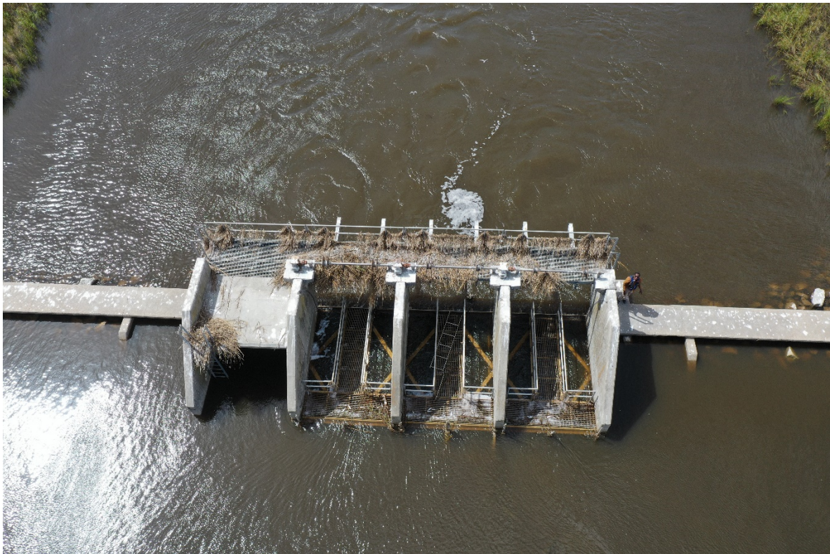
Photo No. 6, Little Constance Structure – Vegetative wrack on structure.
