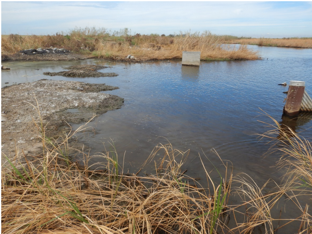
Photo No. 2, Perry Bayou Structure - Risers and wing wall destroyed. Portion of Levee and armament washed away.
