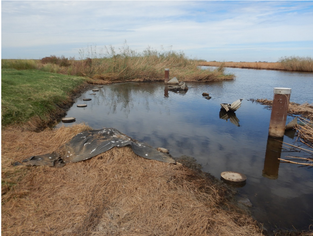
Photo No. 3, McNee Bayou Structure - Risers and wing wall destroyed. Portion of Levee and armament washed away.
