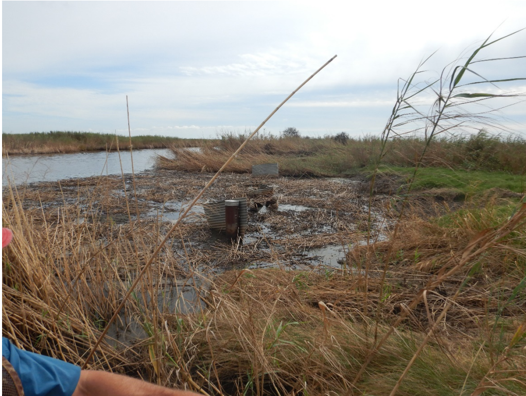
Photo No. 1, New Cop Cop Structure - Risers and wing wall destroyed. Portion of Levee and armament washed away.
