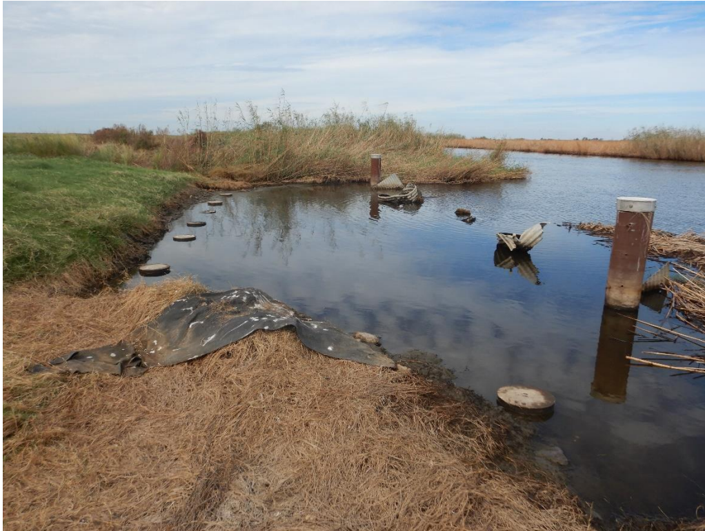
Photo No. 3, McNeece Bayou Structure - Risers and wing wall destroyed. Portion of Levee and armament washed away.
