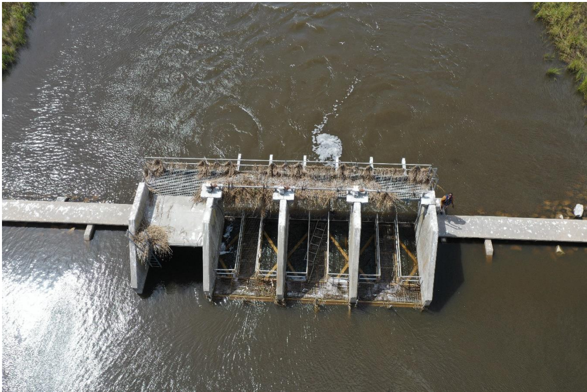
Photo No. 6, Little Constance Structure – Vegetative rack on structure.
