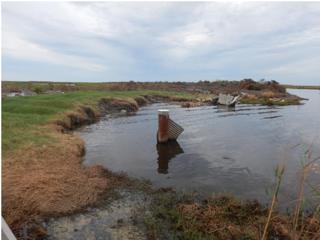
Photo No. 4, Hess Structure - Risers and wing wall destroyed. Portion of Levee and armament washed away.
