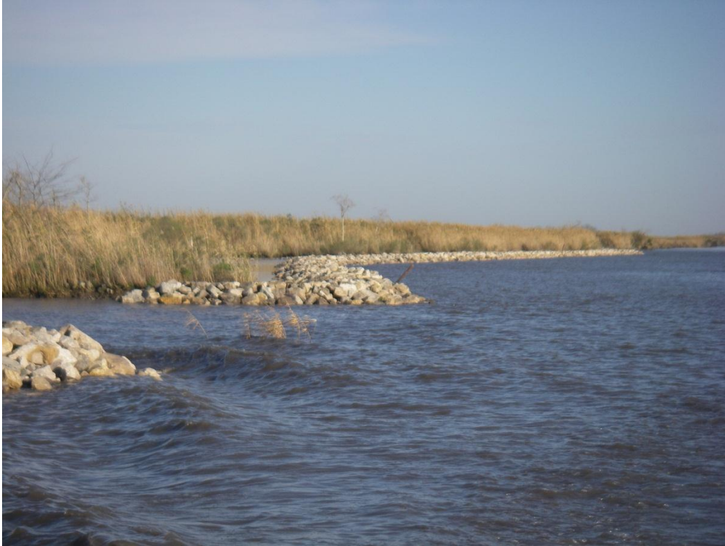
Photo No. 3, Typical Rock Dike
