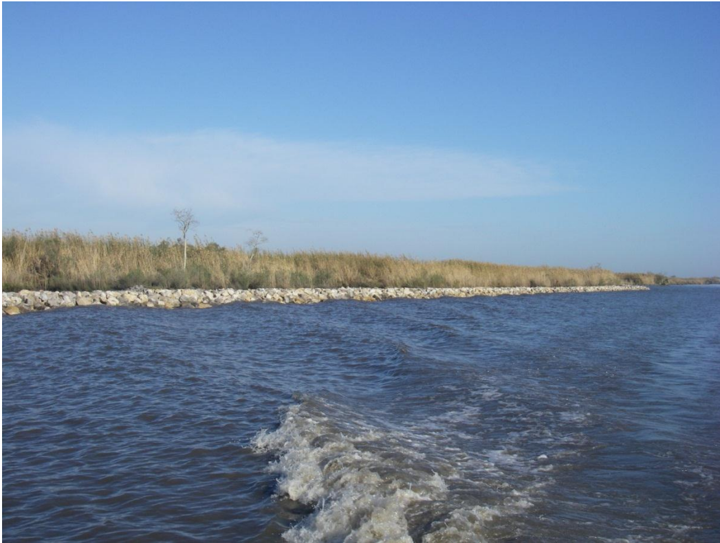
Photo No. 1, Typical Rock Dike
