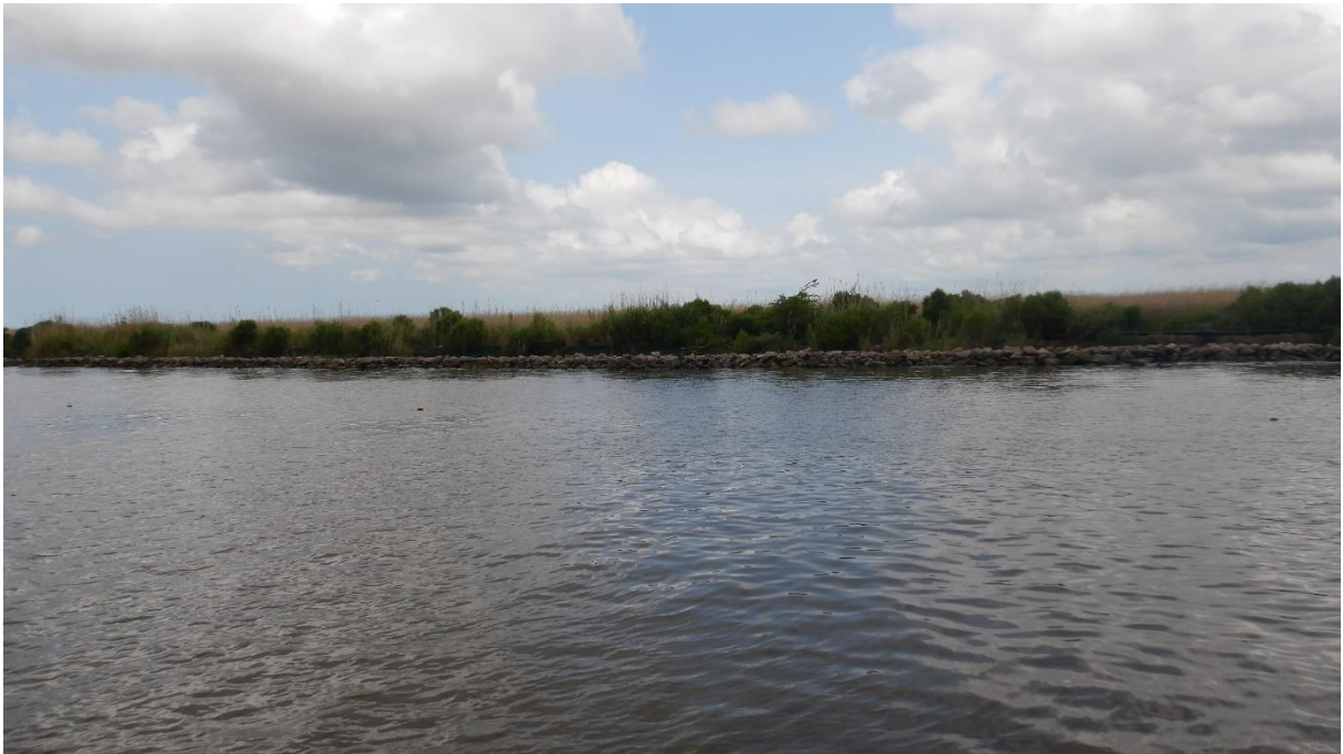
Photo No. 2, Typical Rock Dike ME-13
