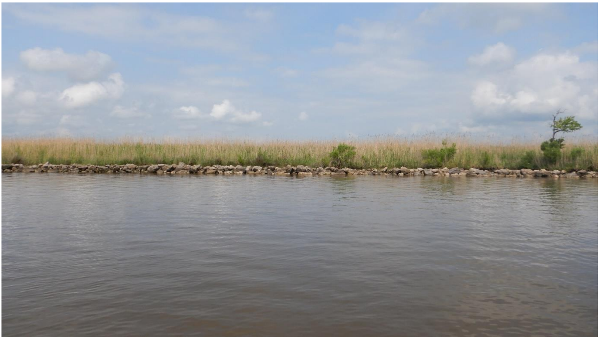
Photo No. 4, Typical Rock Dike ME-13
