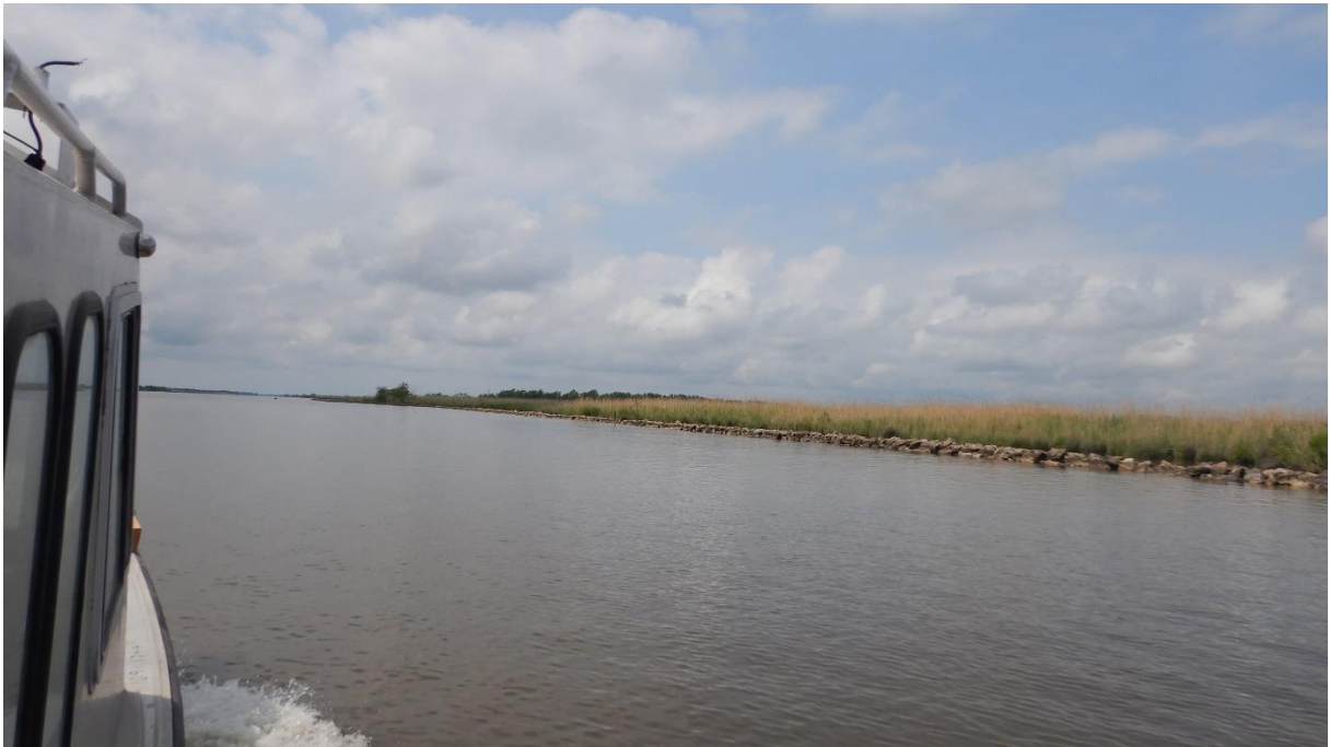
Photo No. 6, Typical Rock Dike ME-13
