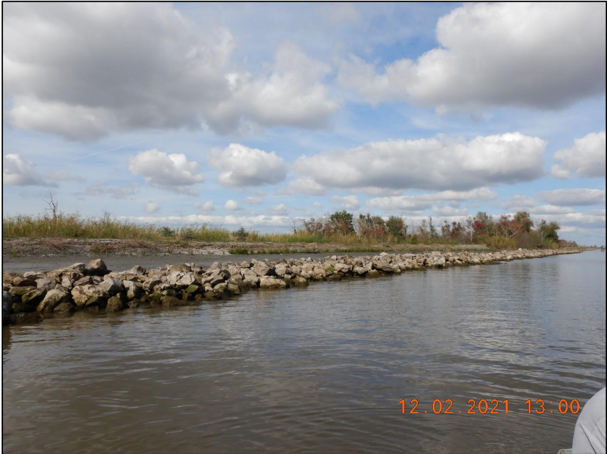
Figure 13. A photograph representing the rock dock condition along the ME-04 and ME-13 shorelines during the most recent data collection effort in 2021.
