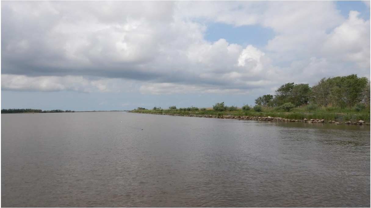
Photo No. 1, Typical Rock Dike ME-04
