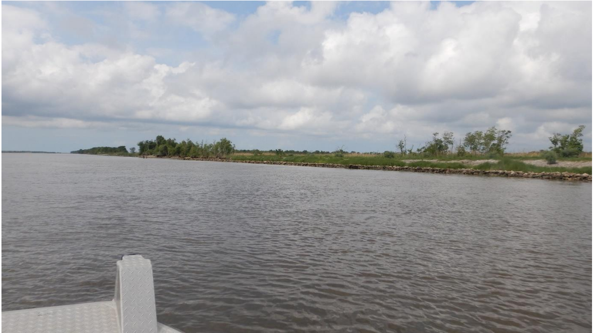
Photo No. 3, Typical Rock Dike ME-04
