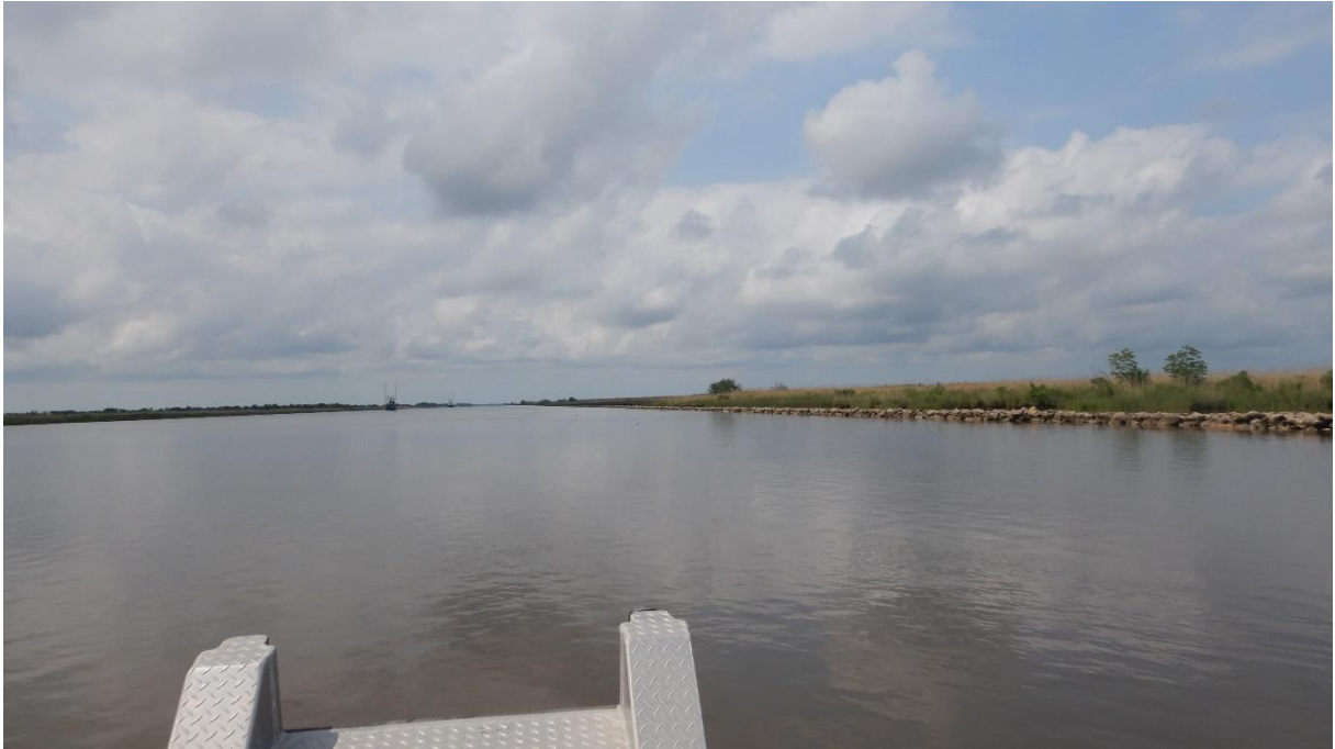
Photo No. 5, Typical Rock Dike ME-13
