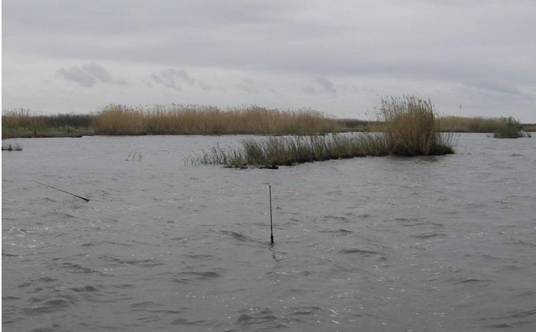
Figure 10. Many terraces have eroded since construction, especially the lakeside terraces (e.g. LS42) which were intended to be sacrificial and buffer the marsh side terraces. Note the cane poles that mark the original corners of the terrace. Picture was taken on March 24, 2010.
