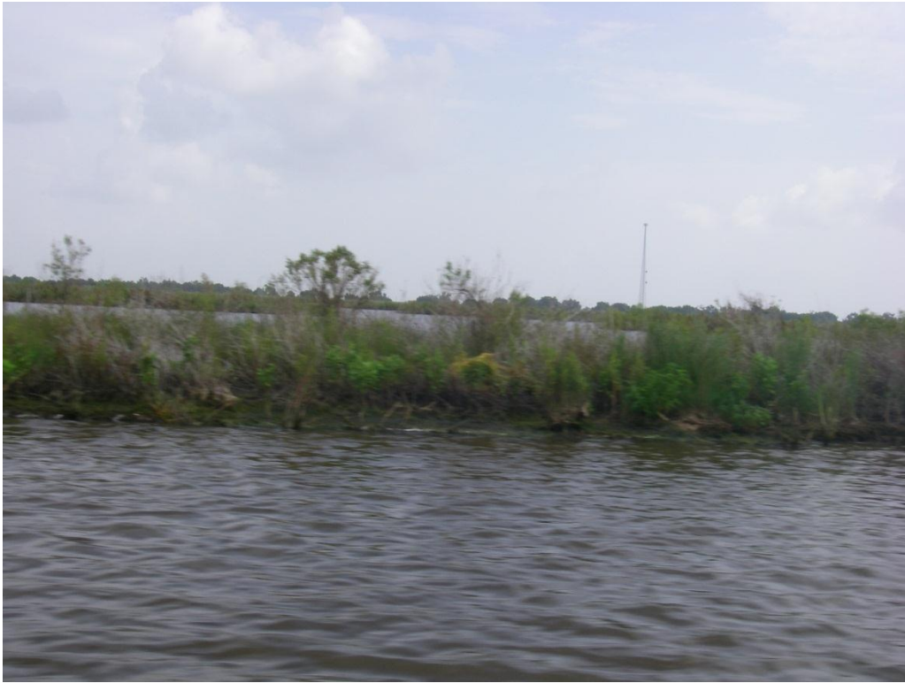
Photo No. 1, Southern Earthen Terraces
