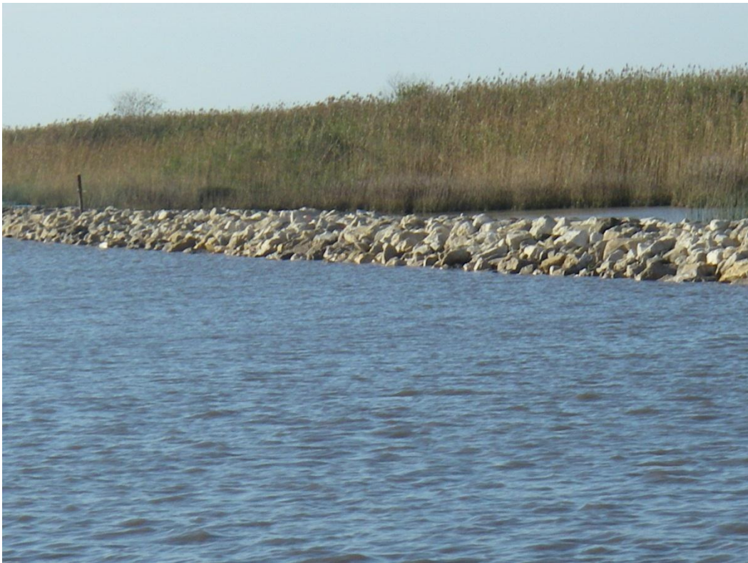
Photo No. 2 , Vegetation Behind Rock Dike
