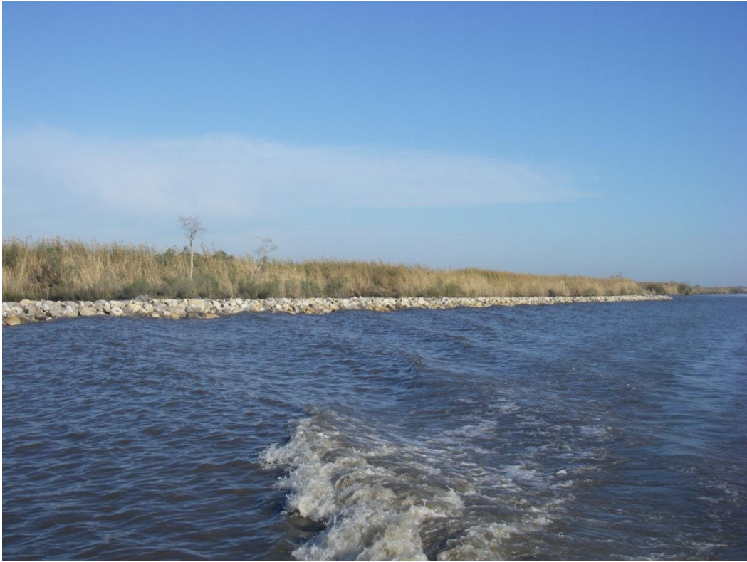
Photo No. 1 , Typical Rock Dike
