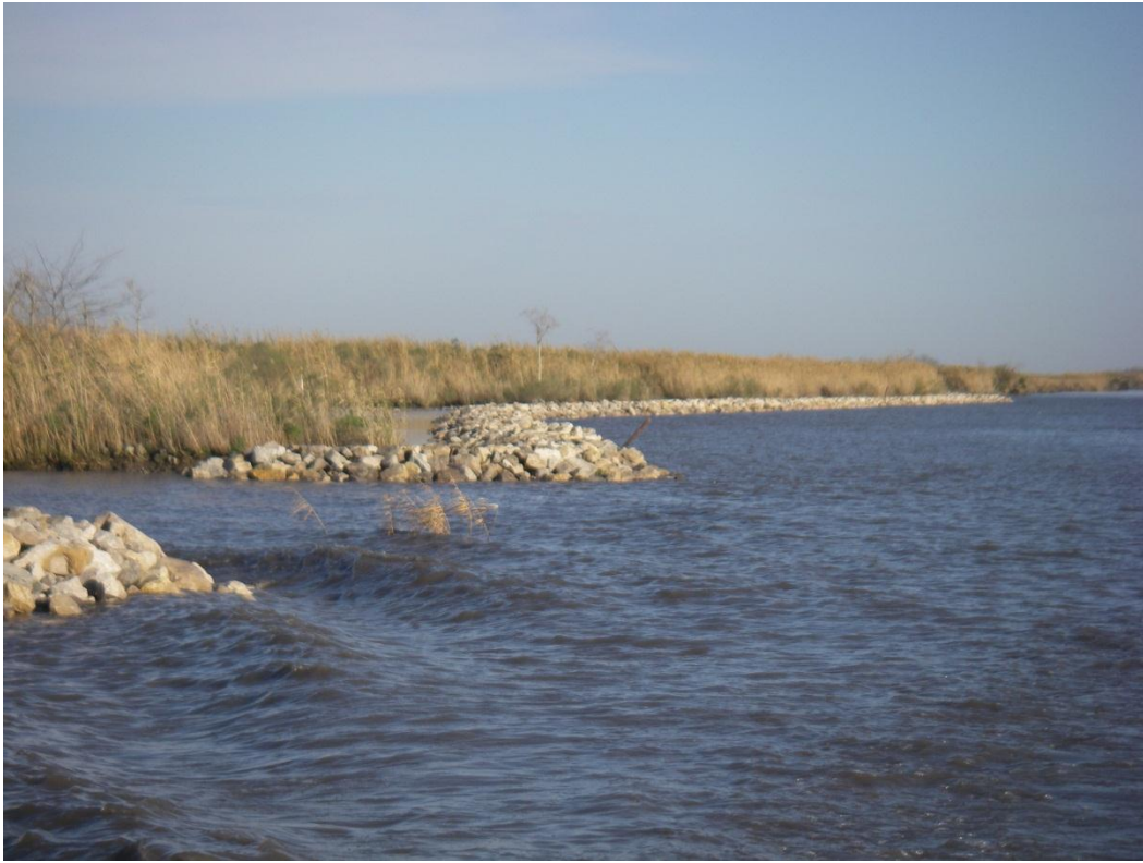
Photo No. 3, Typical Rock Dike
