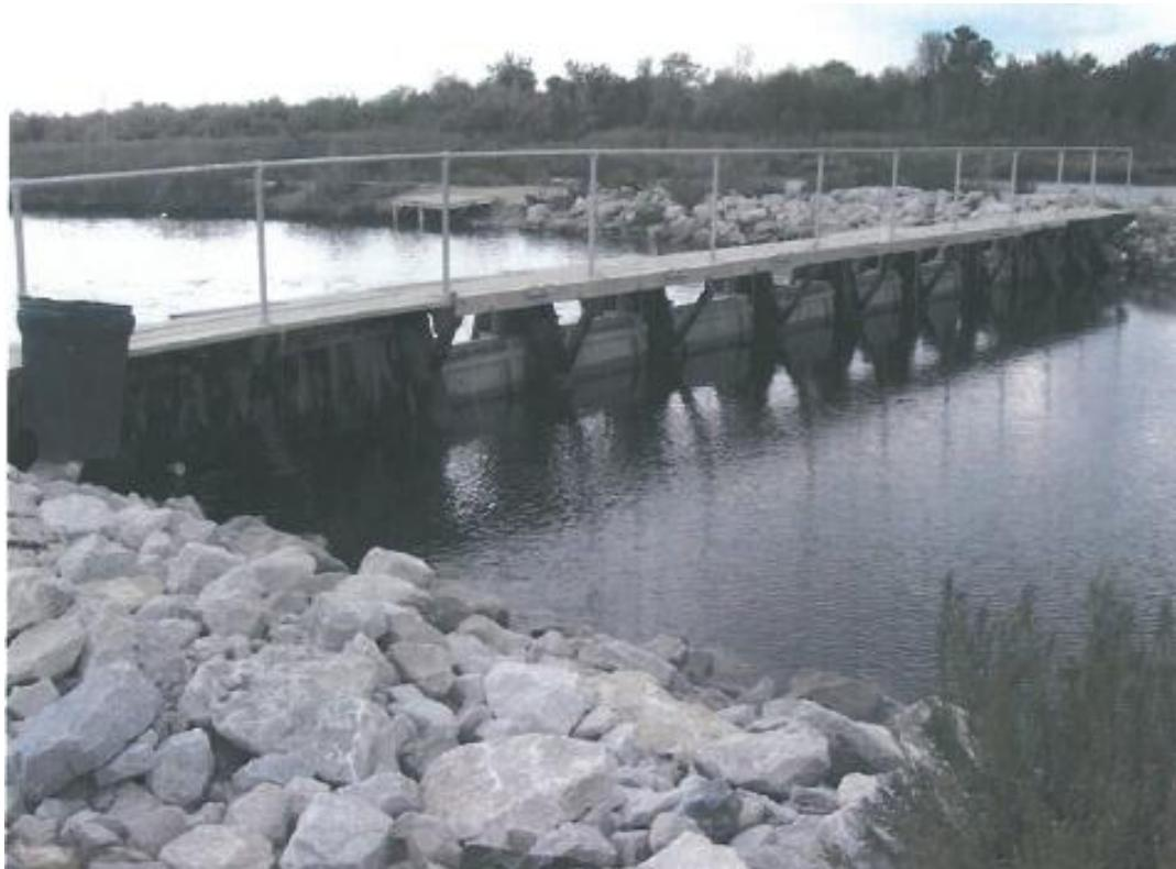
**Figure 18: Variable Crest Weir Water Control Structure**
