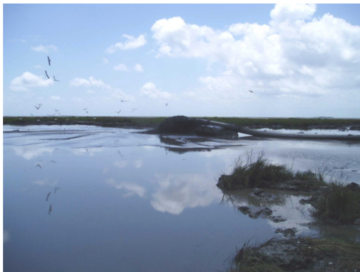
This 24-inch dredge pipe is actively rebuilding marsh by depositing sediment dredged from the lake. As the project progresses, the placed sediment will reach an elevation conducive for growing and sustaining marsh vegetation.
