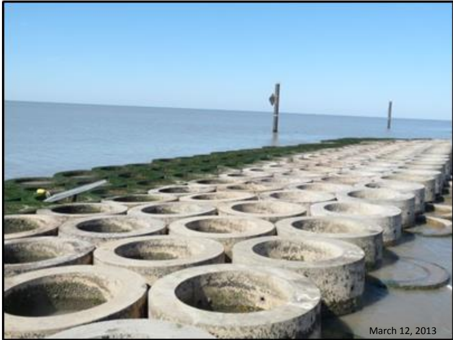
Figure A-6. Standard-Weight Concrete (SW) Oysterbreak showing Algae-Encrusted Gulfward Rings.
