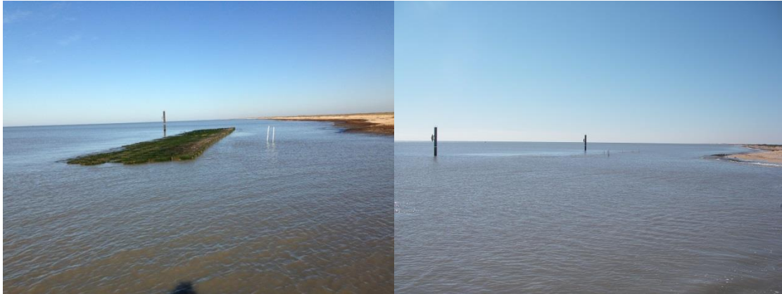
Figure A-11. View Looking West at OysterKrete Oysterbreak at Near-Low Tide (left photo) and again at Near-High Tide (right photo) on March, 12, 2013. Photo by Tommy McGinnis.
