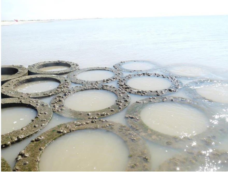
Figure A-15. Colonization of Oysters on a Top-Tier Ring of the Standard-Weight Oysterbreak on October 28, 2013.
