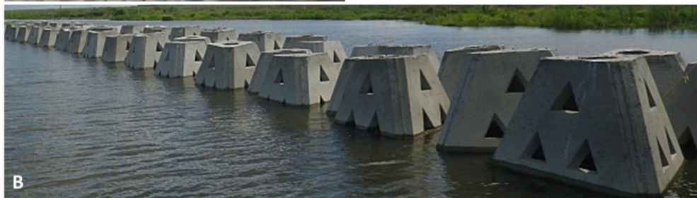
Figure 6. (A) Installation of Wave Attenuation Devices (WADs). Note metal bands attaching the base to the bottom of the WAD. (B) The initial alignment of WADs at Shark Island along the northeastern shore of Vermilion Bay for LA-0016 Non-rock Alternatives to Shoreline Protection Demonstration Project.
