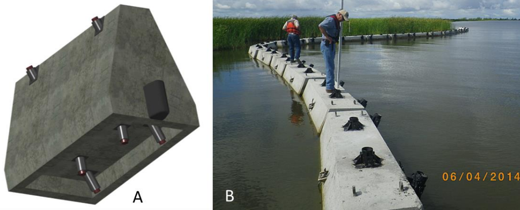
Figure 22. (A) A bottom-view, isometric drawing of a Buoyancy Compensated Erosion Control Modular System (BCECMS) module displays position of pin pilings. (B) The southern half of the BCECMS at Shark Island along the northeastern shore of Vermilion Bay for LA-0016 Non-rock Alternatives to Shoreline Protection Demonstration Project.
