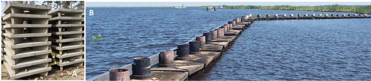
Figure 16. (A) Stacks of EcoSystem Units (ESUs) plates prior to installation. Note hole in the middle of plates for placement around a piling. (B) The northern end of the ESUs after removal of top plate and added brace to stabilize the pilings at Shark Island along the northeastern shore of Vermilion Bay for LA-0016 Non-rock Alternatives to Shoreline Protection Demonstration Project.
