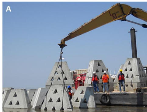
Figure 6. (A) Installation of Wave Attenuation Devices (WADs). Note metal bands attaching the base to the bottom of the WAD. (B) The initial alignment of WADs at Shark Island along the northeastern shore of Vermilion Bay for LA-0016 Non-rock Alternatives to Shoreline Protection Demonstration Project.
