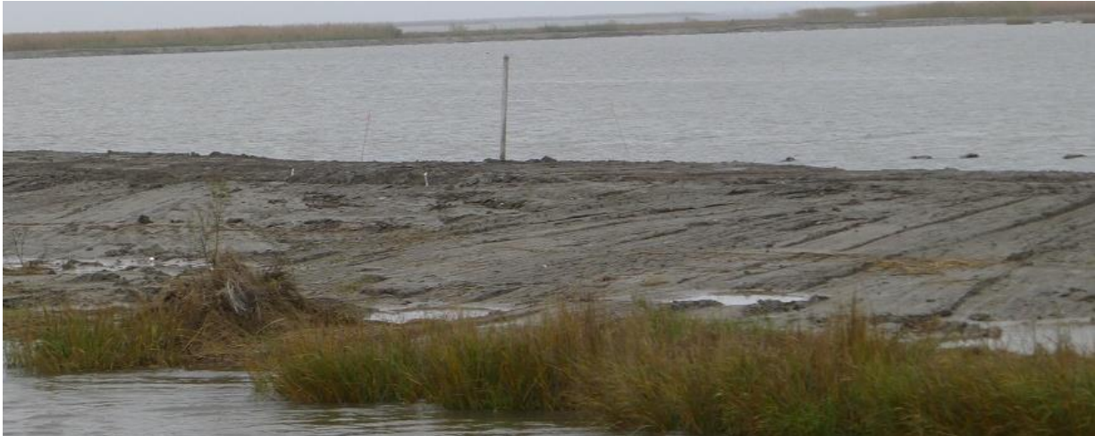
Figure 7: Earthen Ridge and Settlement Plate Photograph
