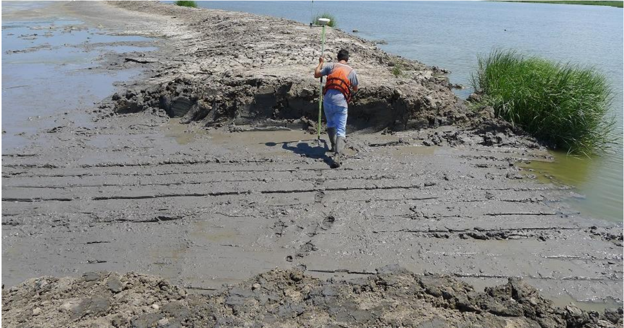
Figure 10: Earthen Containment Dike Gap Photograph
